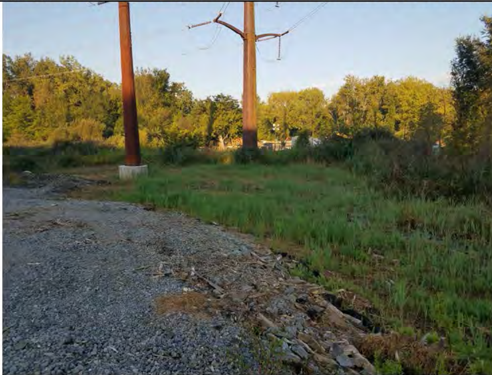
Photo 4: 08/30/2018, Danbury: Map 6, Str1012, stabilization in progress, natural regrowth of vegetation within wetland W1. Photo taken facing west from the gravel pull pad (to remain in place), west side of the north end of Old Sherman Turnpike.
