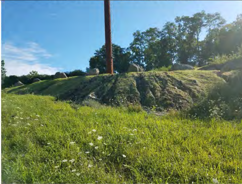
Photo 15: 08/02/2018, Bethel/Brookfield: Map 12, Str1023, slope erosion, south and west slopes. Reference Additional Comments section Page 6 for additional details. Photo taken facing northeast.
