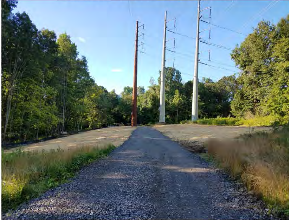
Photo 7: 08/02/2018, Bethel: Maps 07-08, Str1015, work pad restoration. Photo taken facing south.
