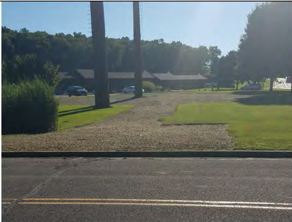
Photo 10: 08/02/2018, Bethel: Map 12, Str1022, work pad restoration, hydroseeded. Photo taken facing east.
