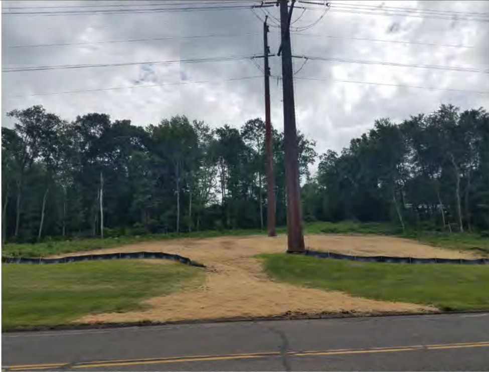
Photo 1: 07/26/2018, Bethel: Map 12, Str1021, work pad restoration performed. Photo taken facing east.
