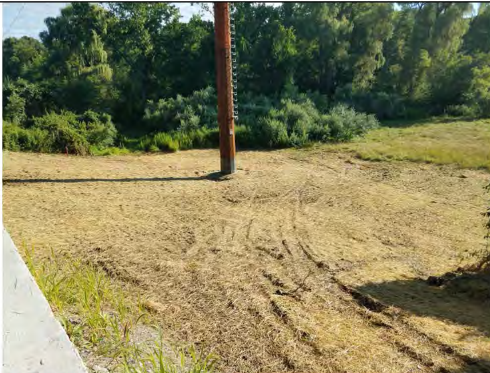
Photo 8: 08/02/2018, Bethel: Map 08, Str1016, work pad restoration. Photo taken facing north.
