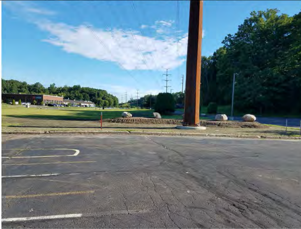
Photo 9: 08/02/2018, Bethel: Map 10, Str1020, work pad restoration, hydroseeded. Photo taken facing north.
