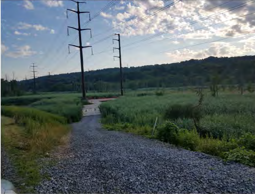
Photo 1: 07/13/2018, Danbury: Map 05, Str1010, access road and timber mat pad. Work pad is within wetland W1. Photo taken facing northeast.
