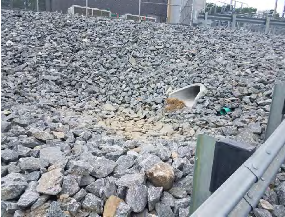
Photo 3: 07/05/18, Stony Hill Substation slope stabilization and site drainage feature abutting wetland W7. Photo taken facing southwest towards the substation from the access road shown in Photo 2.
