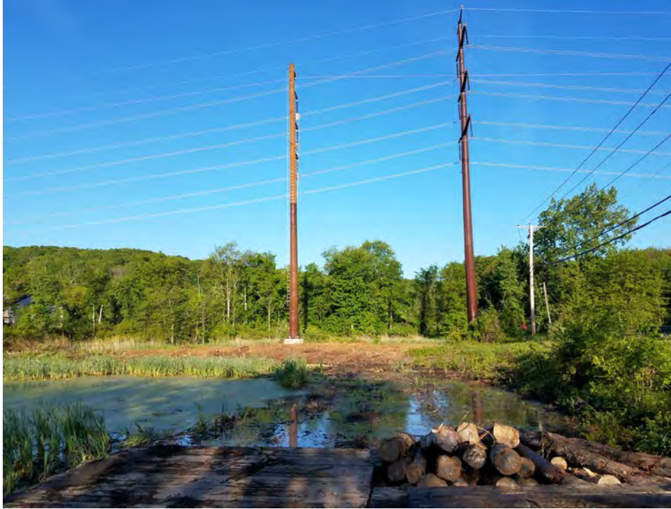
Photo 1: Bethel: Map 03, Str1007 and Wetland W1, Removal of timber mat access and work pad. Photo taken facing west, Structure Str1007 shown central in the photo.
