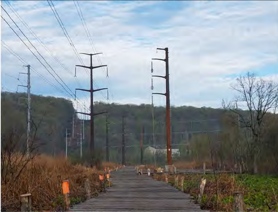
Photo 3: 05/04/2018, Bethel: Map 02, Str1004 through Str1005, weathered steel structures installed. Photo taken facing west from Str1003 toward Str1005 in the distance.
