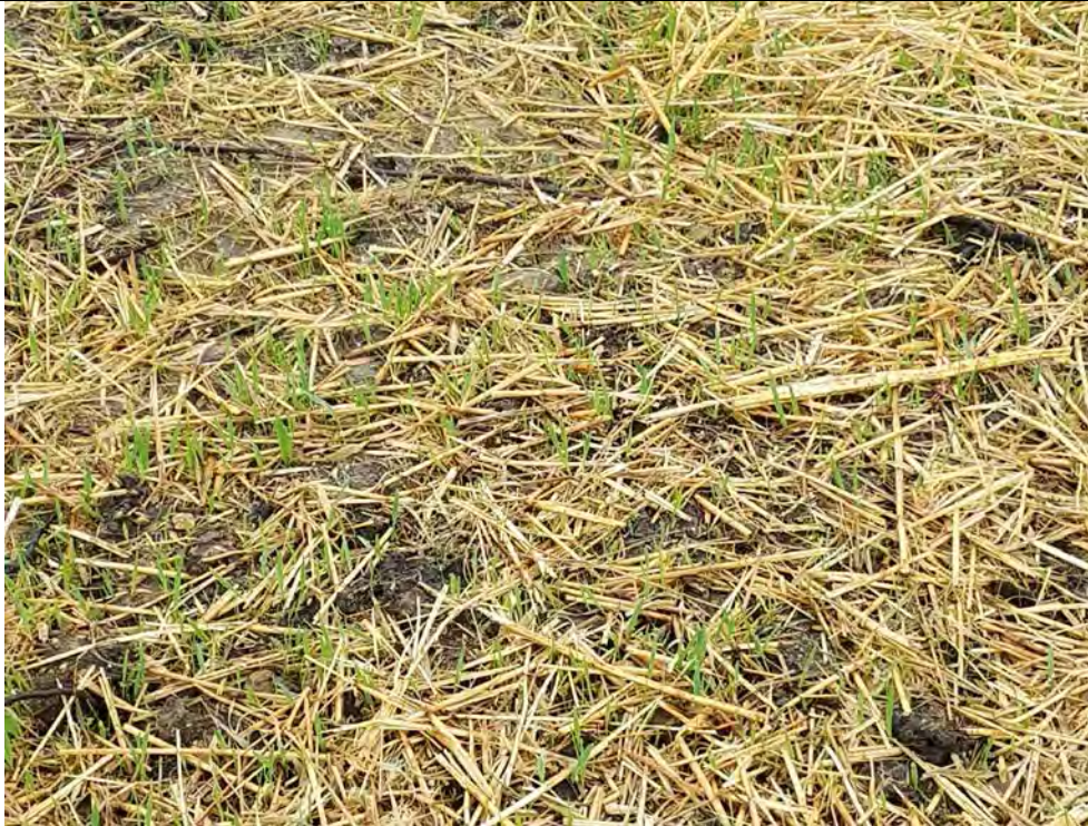
Photo 6: 04/26/2018, Danbury, Map 06, slope and exposed soil stabilization, new grass growth at the area shown in Photo 3.
