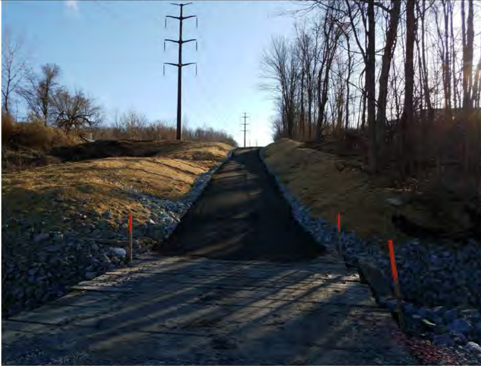
Photo 1: 4/05/2018, Danbury: Map 06, paved access road construction to Str1013.
