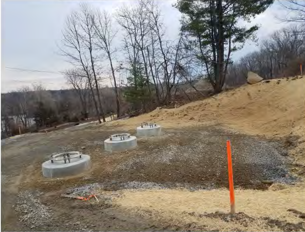
Photo 5: 04/13/2018, Brookfield: Map 13, Str1026 structure foundations. Photo taken facing east.
