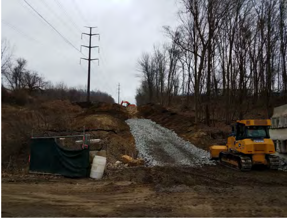
Photo 5: 03/28/2018, Danbury: Map 06, access road construction to Str1013.
