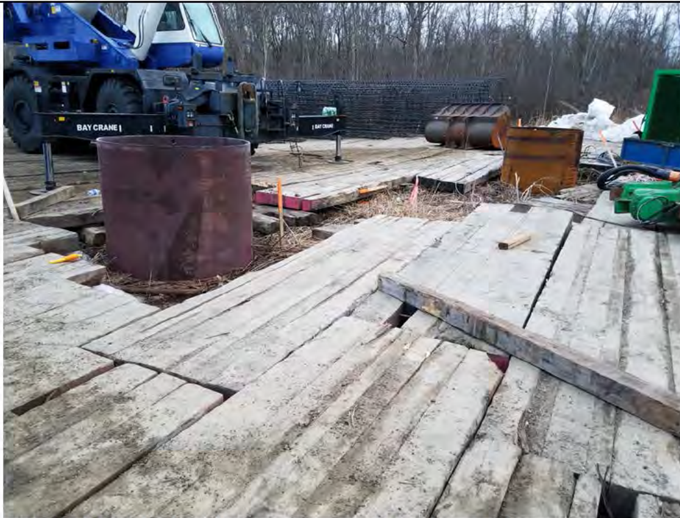
Photo 2: 03/23/2018, Bethel: Map 02, Str1002, drilling structure foundation holes.
