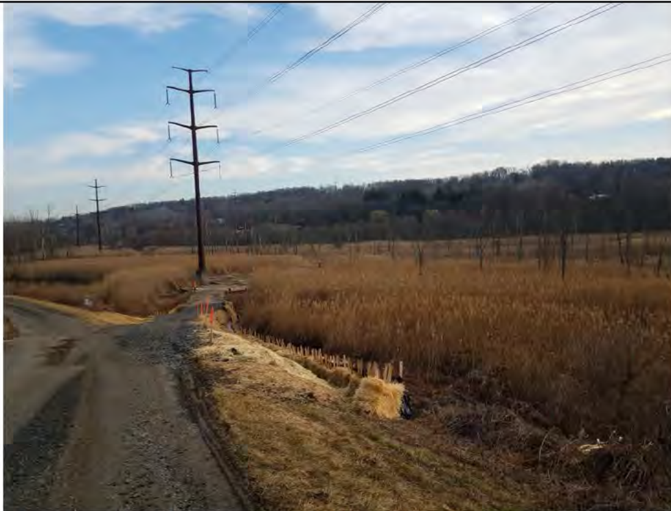
Photo 8: 03/01/2018, Danbury: Map 05, access road to Str1010, E&S installed between the gravel road and Wetland W1.
