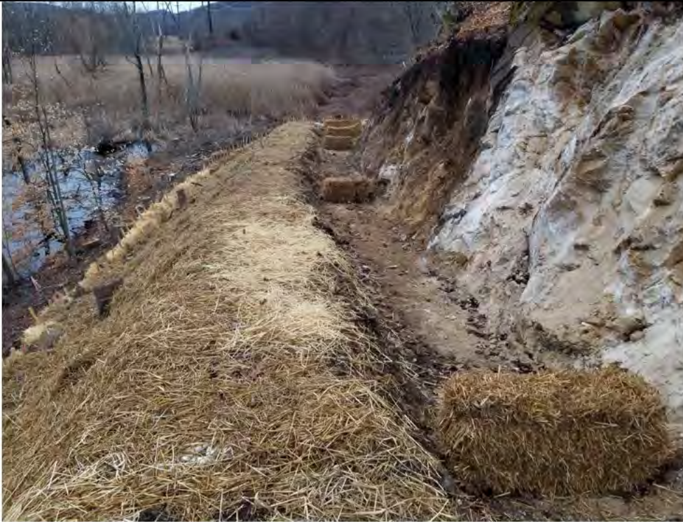
Photo 5: 02/22/2018, Danbury: Map 04, swale with check dams, mulch placement, and hay bales abutting Wetland W1 at bottom of slope east of Str1009, photo taken facing south towards Str1008.
