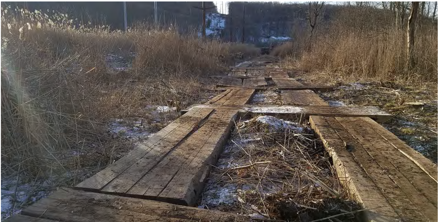
Photo #4: 1/3 – Near Structure 1003 west of Plumtree Substation – Alternate view of the location shown in Photo #3. Facing west.
