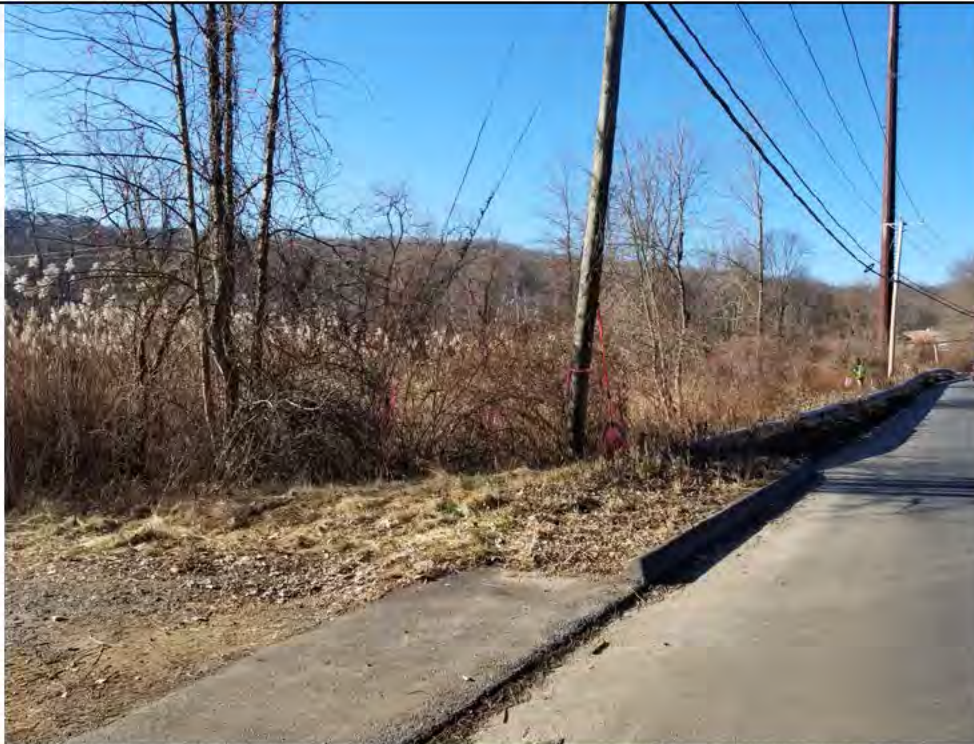
Photo 8: 12/21/17, Bethel: Map 3, Pond Area off Shelter Rock Road, Temporary Wetland Impact Area, proposed access road to Str1007, timber mats to be used for construction of access road.
