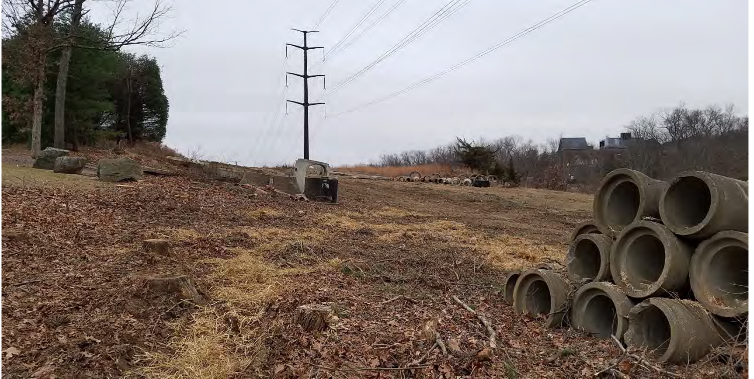
Photo #3: 12/22 – Between Park Ridge Road and Structure 1023 - Straw mulch applied over exposed soils post-tree clearing. Facing southwest towards Structure 1023.
