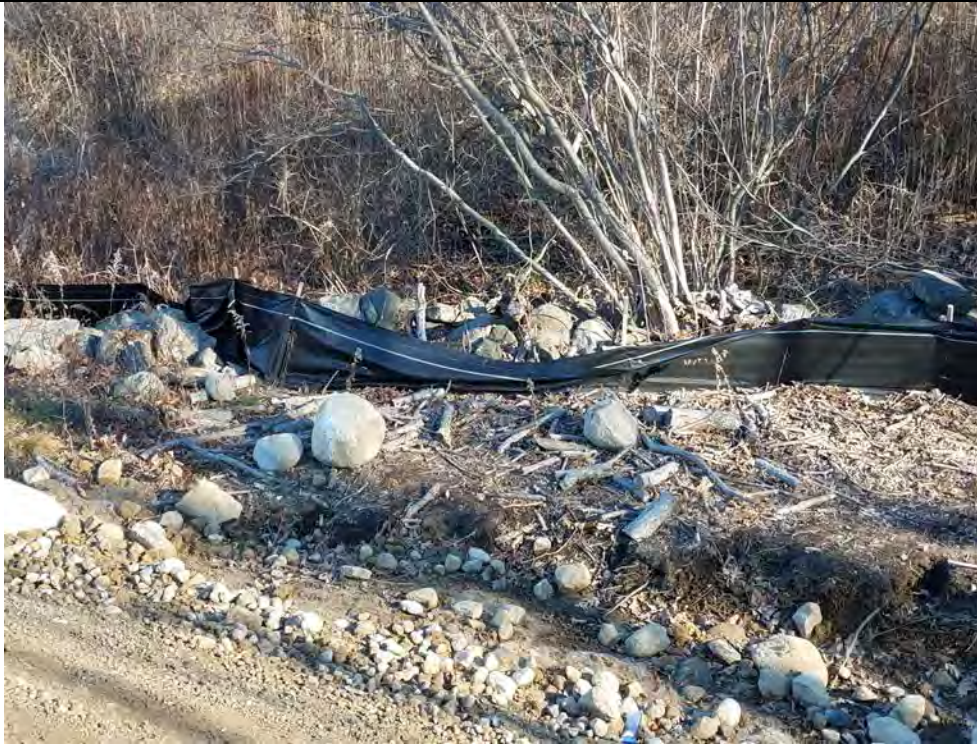
Photo 1: 12/07/17, Str4647A, northeast corner silt fence line, photo taken facing east.
