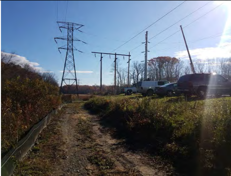
Photo 2: 11/09/17, Stony Hill Substation, north perimeter silt fence, photo taken facing east.
