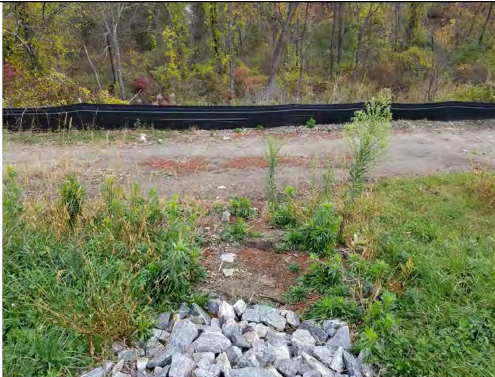
Photo 8:10/26/17: Stony Hill Substation, Str4647A and substation access road drainage, photo taken facing north.
