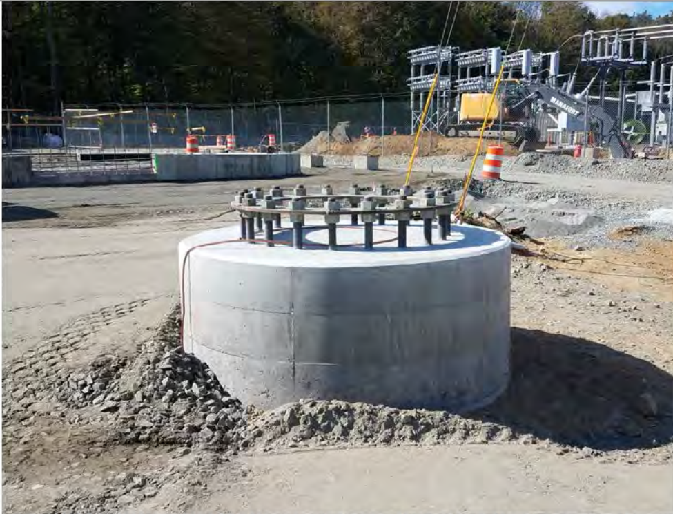
Photo 1: 10/05/17, Stony Hill Substation, Str4647A concrete base, photo taken facing southwest.
