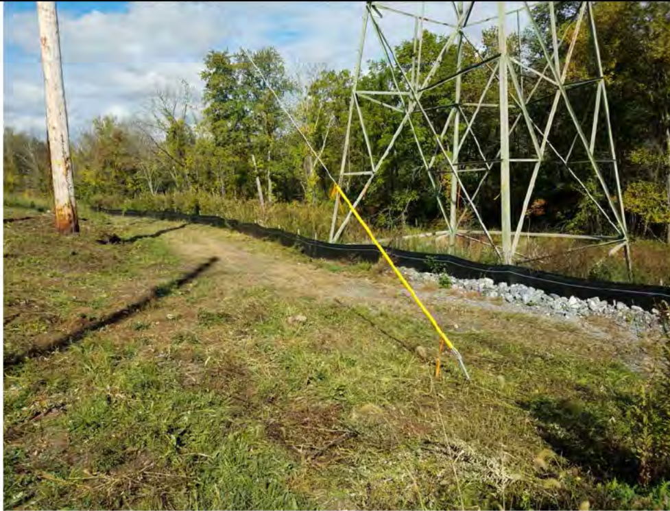
Photo 3: 10/12/17: Stony Hill Substation, silt fencing placement, photo taken facing east.
