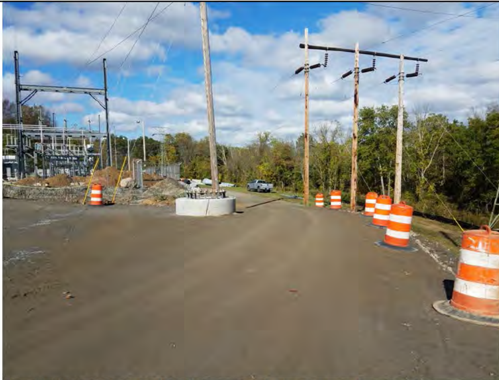
Photo 2: 10/12/17: Stony Hill Substation, Str4647A access road, photo taken facing west.
