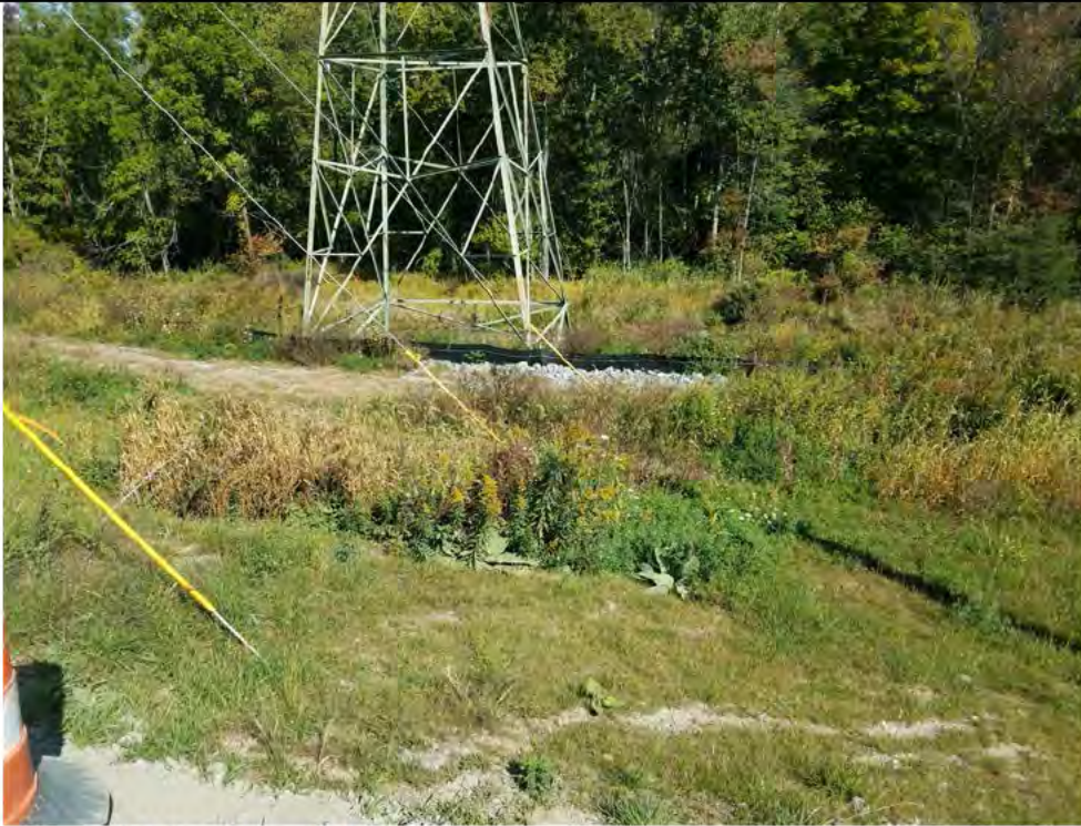
Photo 3: 10/05/17, Stony Hill Substation, silt fence installation along veg clearing limits.
