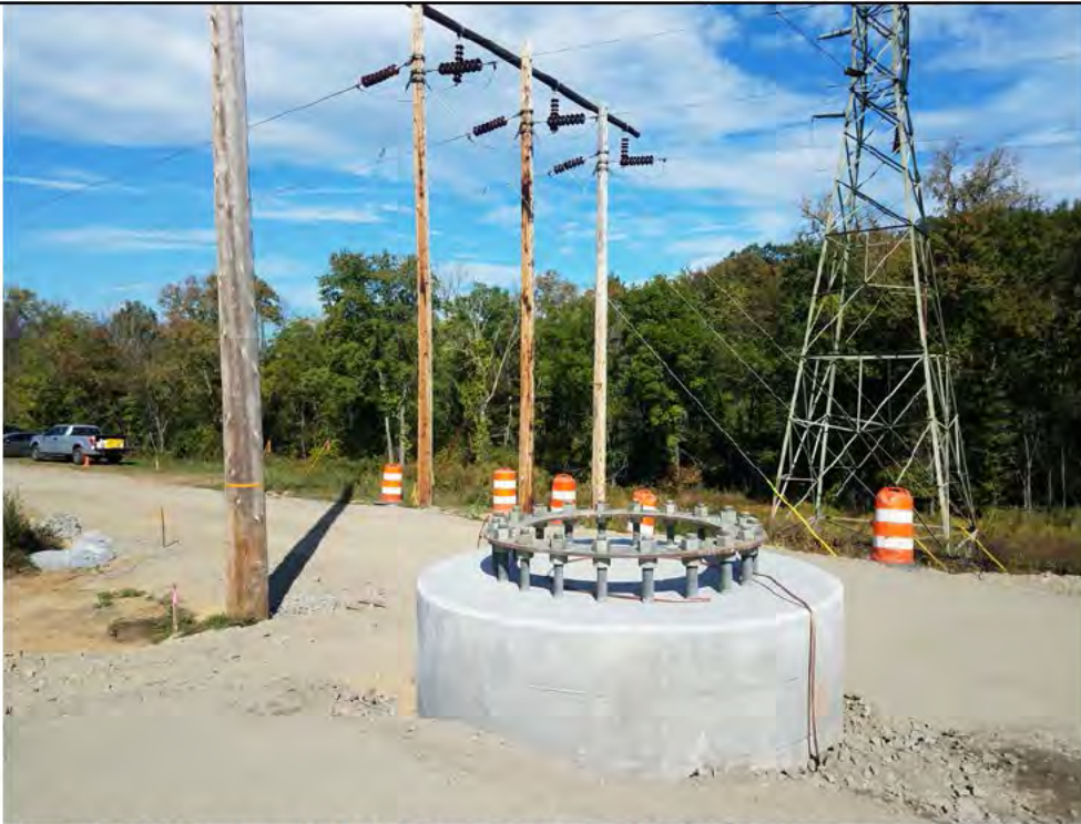
Photo 2: 10/05/17, Stony Hill Substation, Str4647A concrete base, photo taken facing north.
