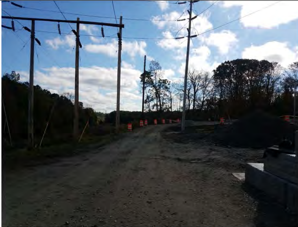
Photo 1: 10/12/17: Stony Hill Substation, Str4647A access road, photo taken facing east.
