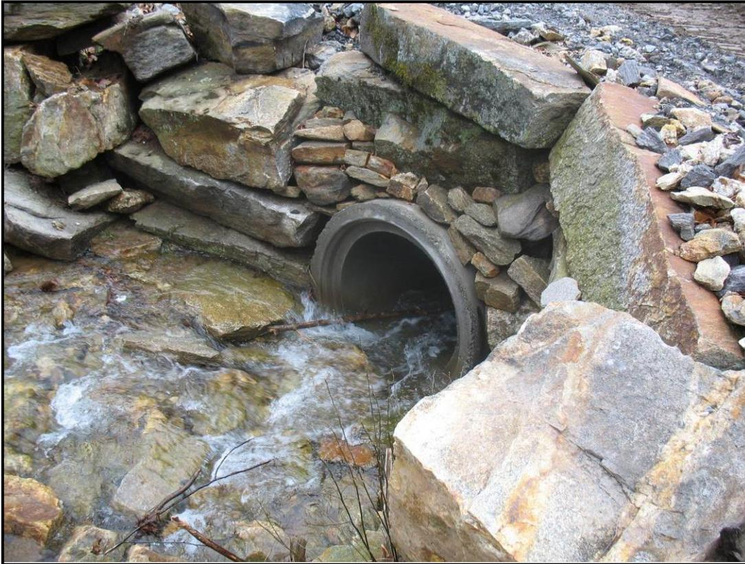
Culvert and riprap for stream crossing.
