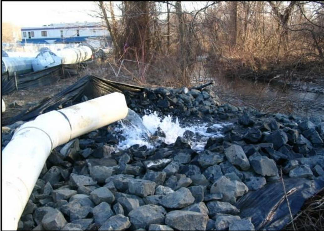
Riprap underlain by geotextile fabric
