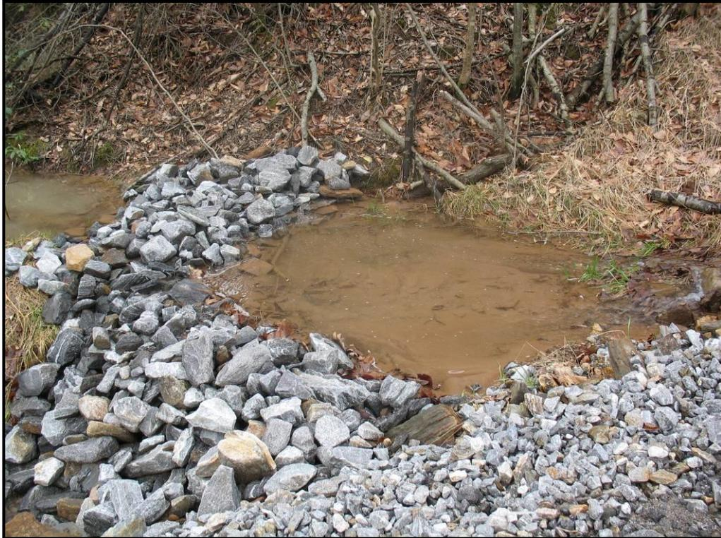
Stone check dam at construction site.
