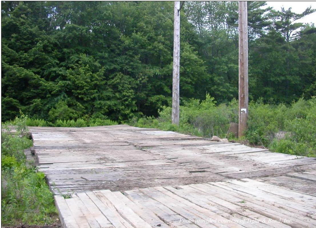
Construction mat wetland work-pad for de-energized work.
