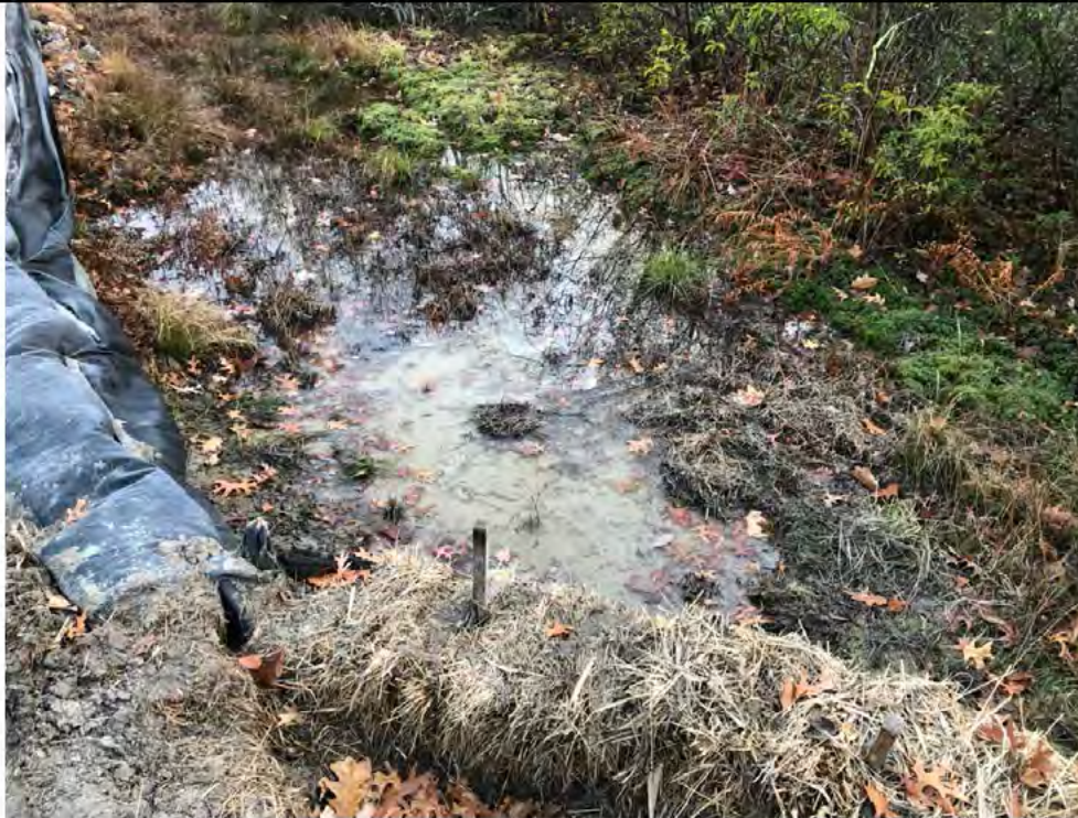
Photo 9: 12/01/17, Watertown: Map 14, sediment impacts to W-C20 awaiting restoration.
