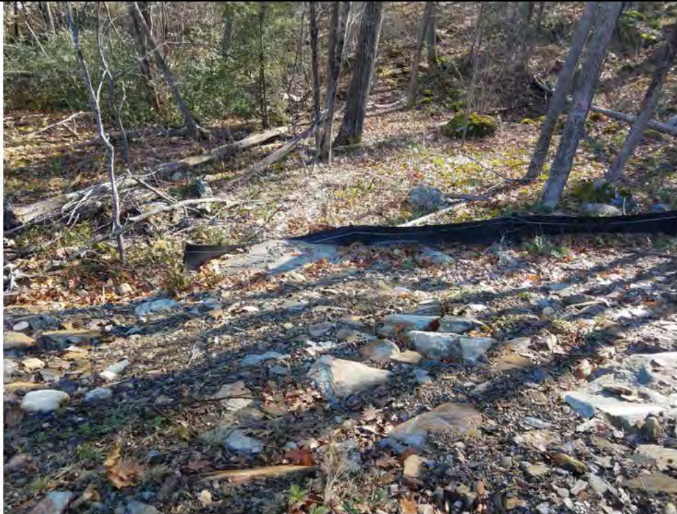
Photo 5: 11/24/17, Thomaston: Map 22, Str69 at the toe of the east slope, silt fence repairs required.
