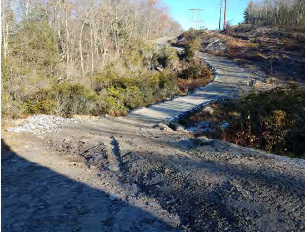
Photo 7: 11/24/17, Watertown: Map 14, CORRECTIVE ACTION-Formed water bar upland of W-C20.
