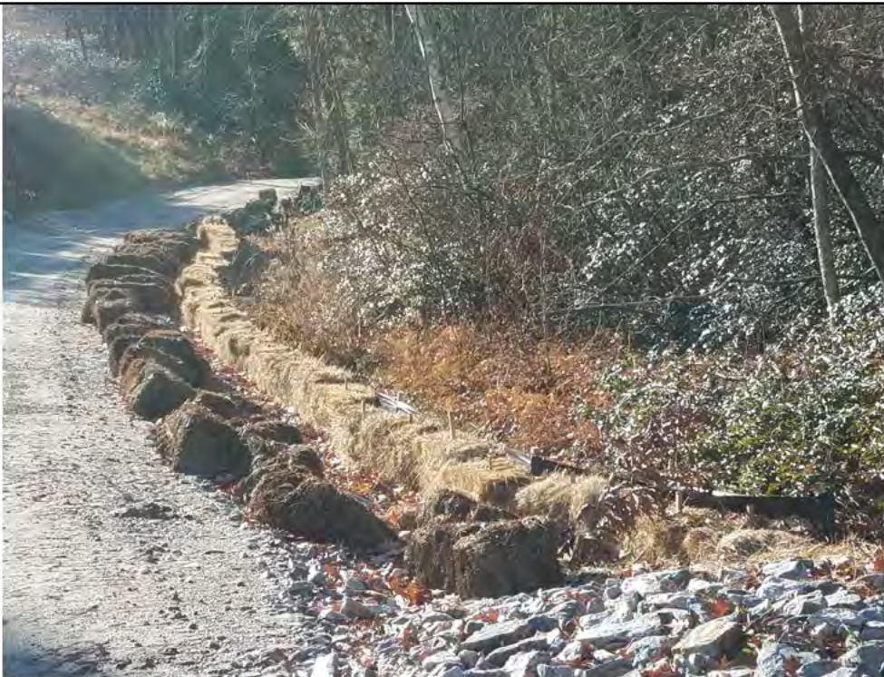
Photo 8: 11/24/17, Watertown: Maps 09-14, CORRECTIVE ACTION-Replaced hay bales at many locations throughout the ROW.
