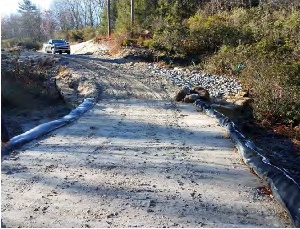
Photo 1: 11/24/17, Watertown: Map 14, timber mat crossing conditions at W-C20, buildup of sediments on timber mats.
