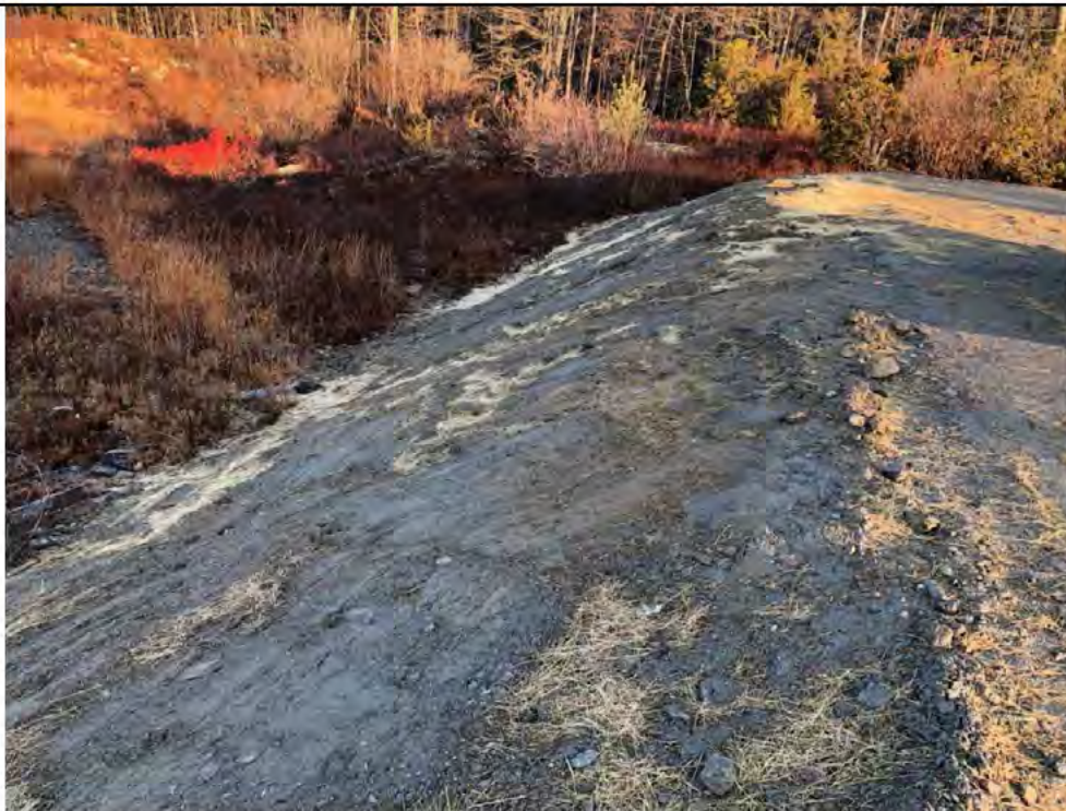
Photo 10: 12/01/17, Watertown: Maps 3-4, various areas of pads between Str3 and Str9, straw and grass seed blown off by wind conditions.
