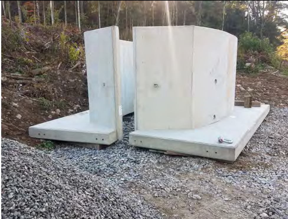
Photo 6: 10/20/2017, Harwinton: Map 32, culvert replacement at W-F11/S-F10, culvert halves pictured.
