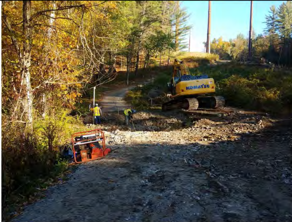
Photo 7: 10/20/2017, Harwinton: Map 32, culvert replacement at W-F11/S-F10, southwest of Str87.
