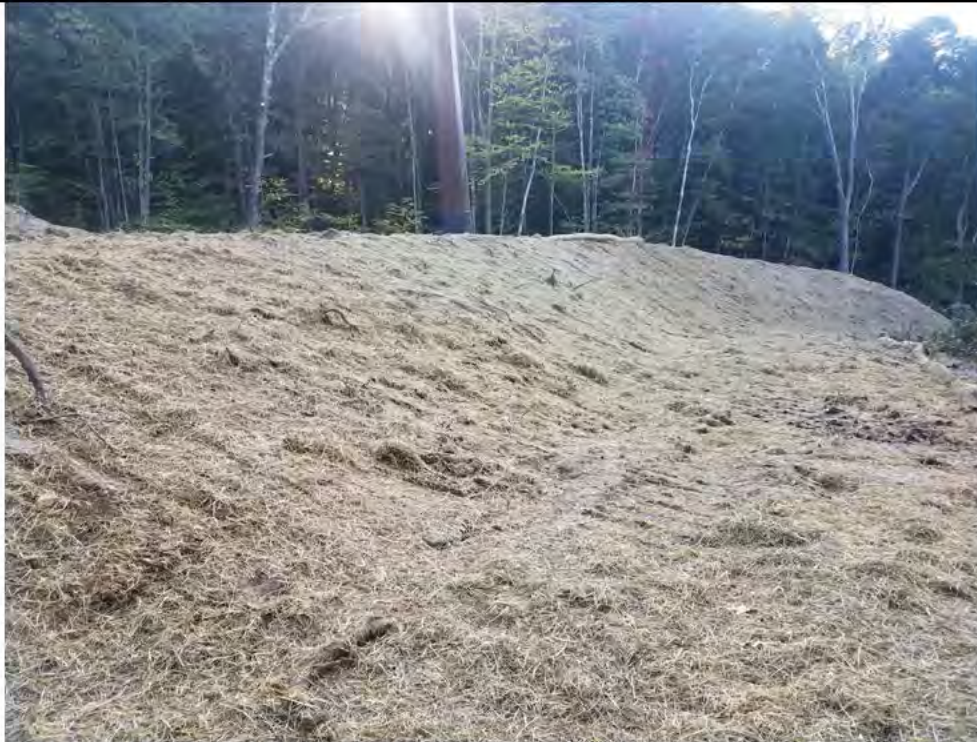
Photo 3: 10/06/2017, Thomaston: Map 18, Str51 restoration completed.
