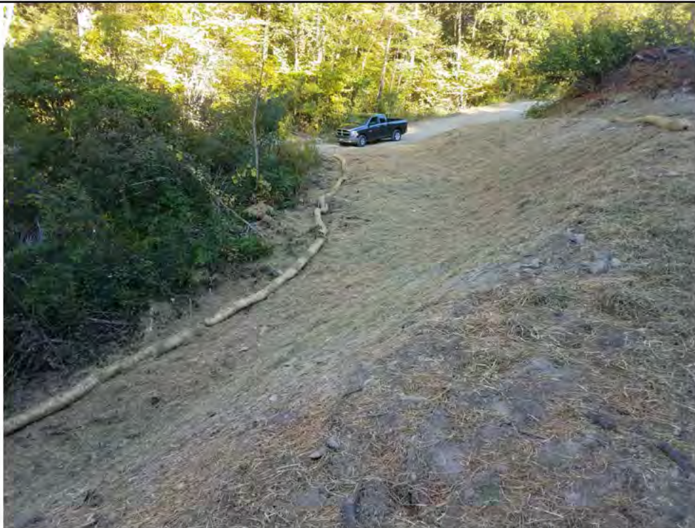
Photo 4: 10/06/2017, Thomaston: Map 18, Str51 restoration completed, straw wattle placement.
