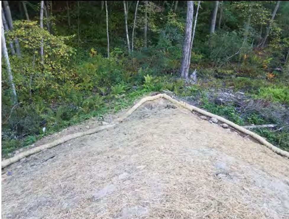
Photo 5: 10/06/2017, Thomaston: Map 18, Str51 restoration completed, straw wattle placement.
