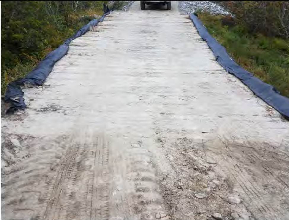
Photo 1: 10/06/2017, Watertown: Map 14, Wetland W-C20 timber mat crossing, sediment buildup on mats.
