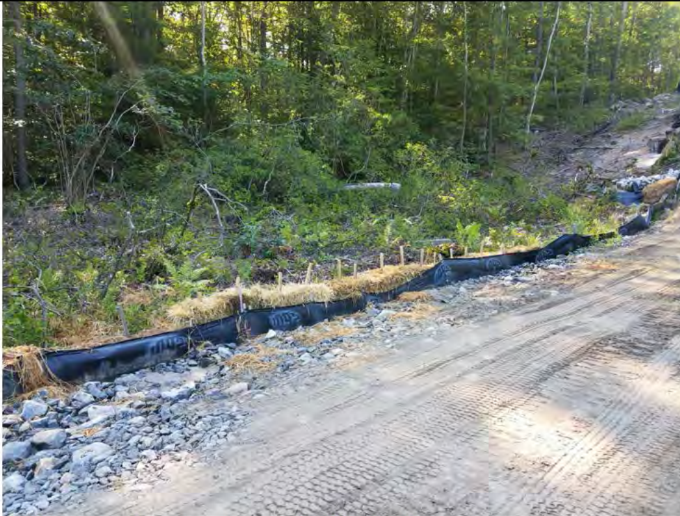
Photo 4: 07/21/2017, Watertown: Map 11, access road at W-C12, E&S repairs.
