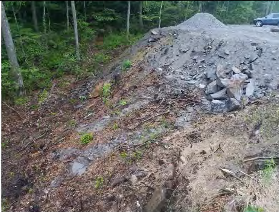
Photo 5: 07/07/2017, Watertown: Northwest corner of Str38 pad, rills and sedimentation off pad slope and visible surface water runoff from access road down slope.
