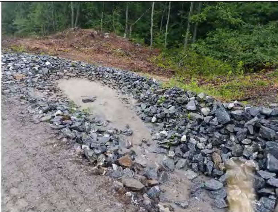
Photo 8: 07/07/2017, Watertown: Access road to Str43, excess sediment buildup in temporary sediment trap.
