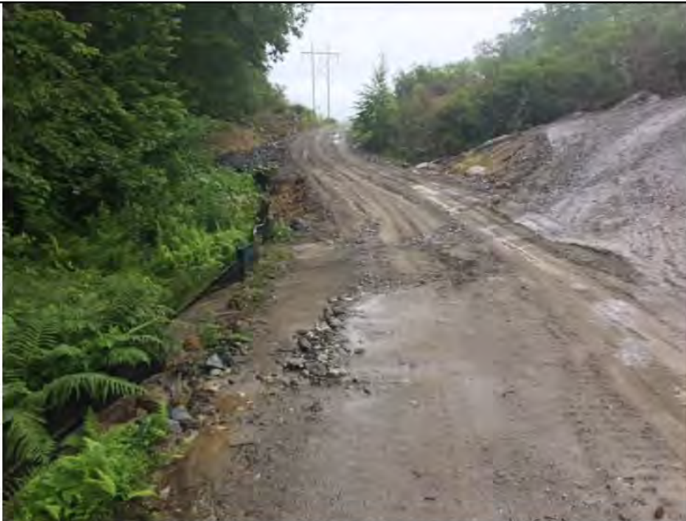
Photo 4: 07/07/2017, Watertown: Area of Str37 at W-C18, silt fence failure, sedimentation into W-C18.
