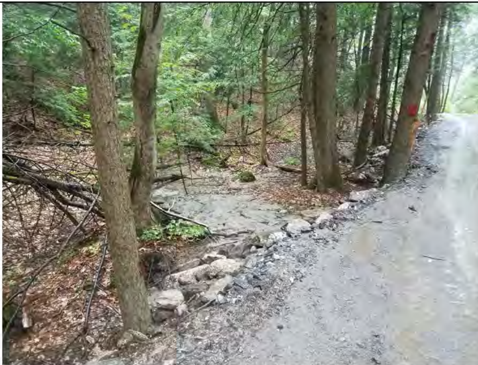
Photo 10: 07/07/2017, Watertown: Access road to Str45, surface water runoff, sedimentation into wooded area.
