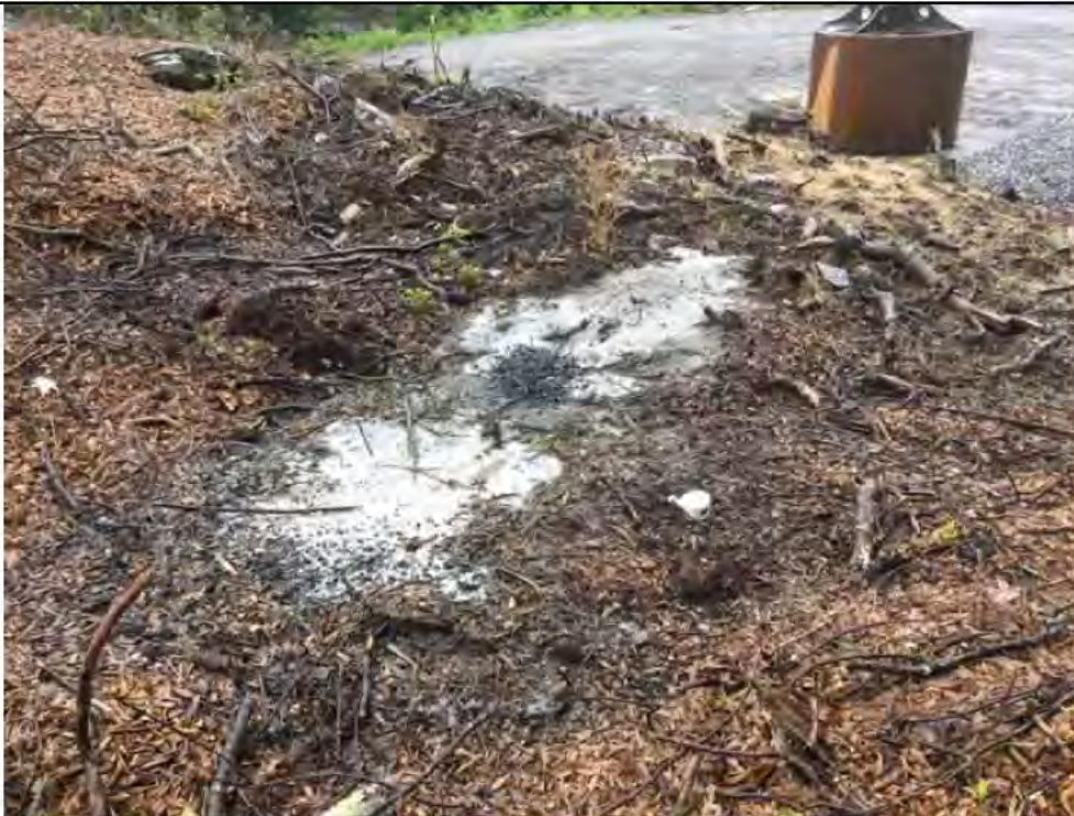
Photo 6: 07/07/2017, Watertown: Upland of Str38 pad, concrete discharge (truck cleanout).
