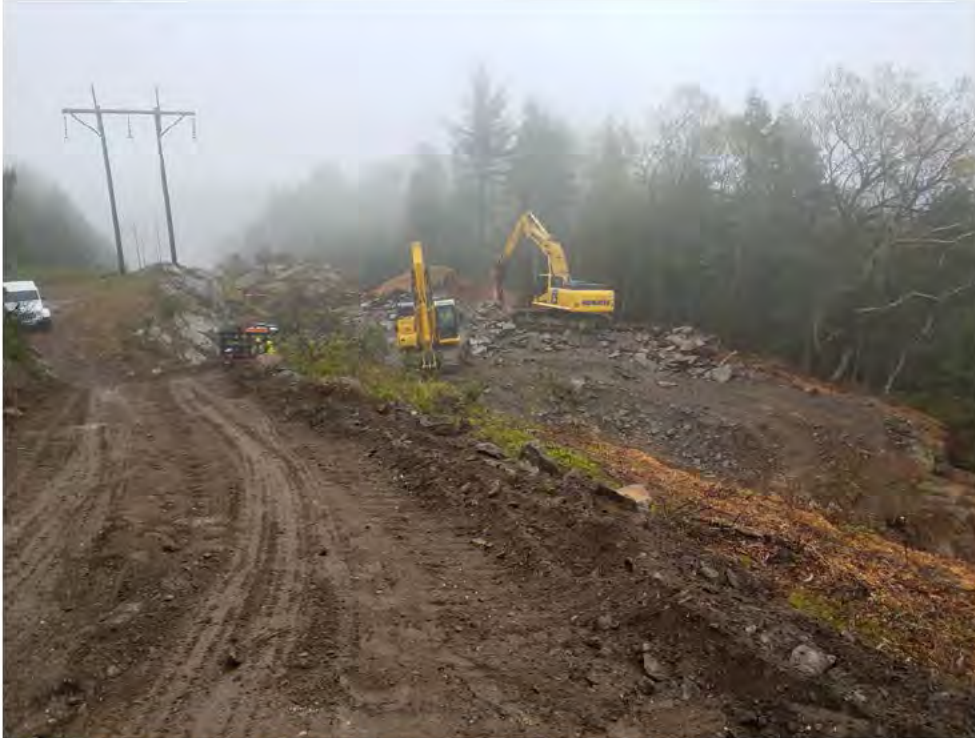
Photo 7: 05/05/2017, Watertown: Map 17, Str49 Pad construction, rock hammering and rough grading.
