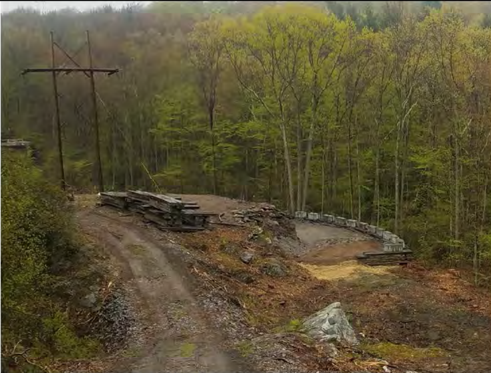
Photo 8: 05/05/2017, Thomaston: Map 18, Str50 pad construction completed.
