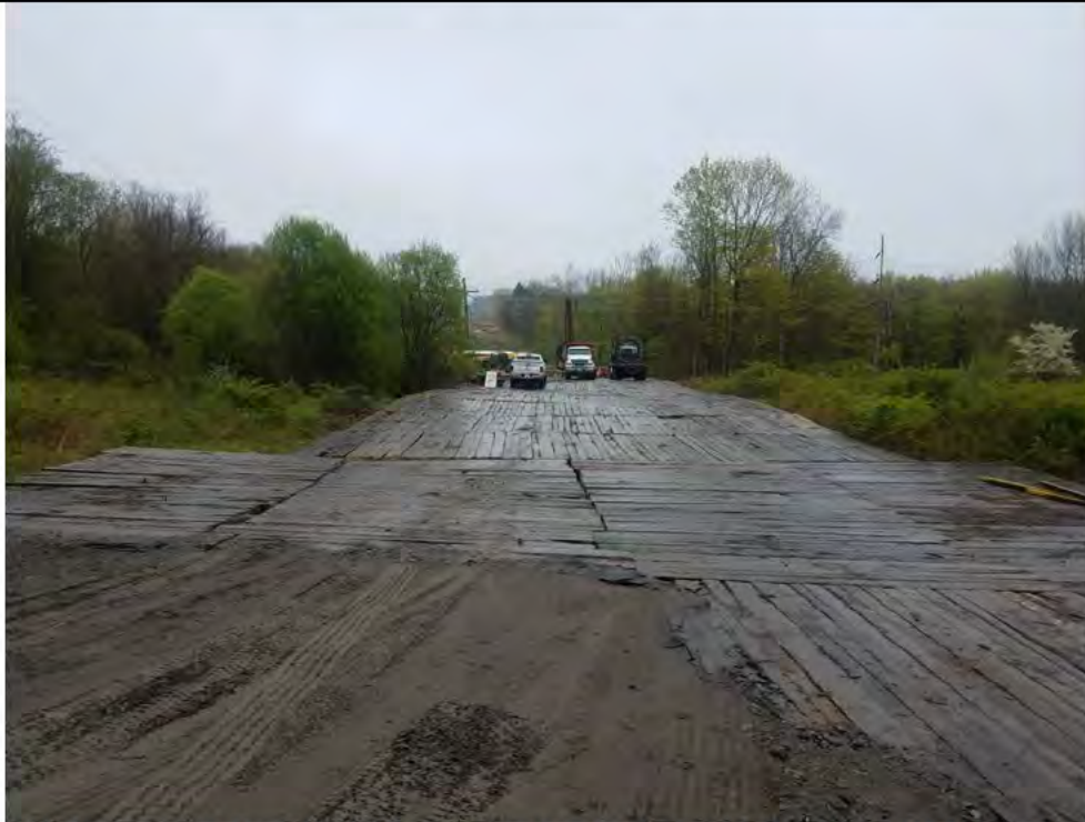
Photo 10: 05/05/2017, Thomaston: Map 22, timber mat pad at Str63-Str64, & wetland W-D12 and vernal pool VP-D12-1.
