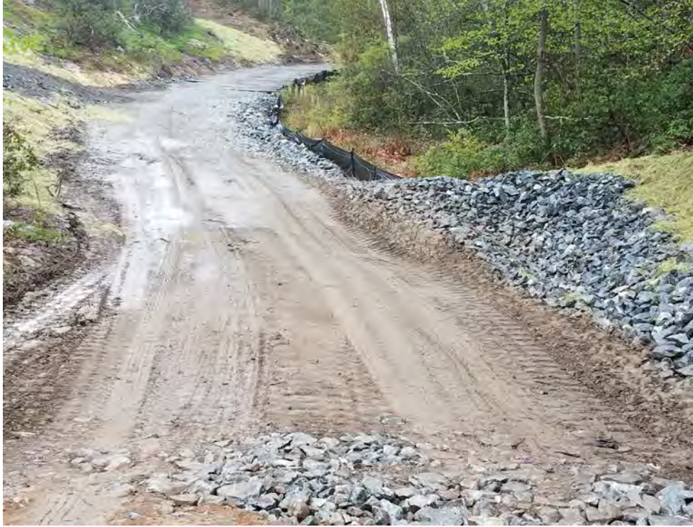
Photo 5: 05/05/2017, Watertown: Map 13, E&S controls and access road improvements in area of wetland W-C18.
