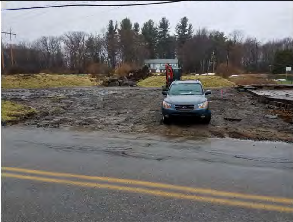
Photo 8: 3/31/2017, Litchfield: Map 29, Str81 abutting Campville Road, E&S, tracking pad, and catch basin protection needed. Corrections were reportedly made on this day after the time of this inspection.
