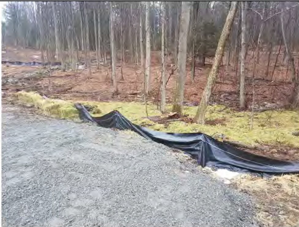
Photo 12: 3/31/2017, Harwinton: Map 35, Str96 abutting W-G1, restoration and installation of E&S, post wetland impact.
