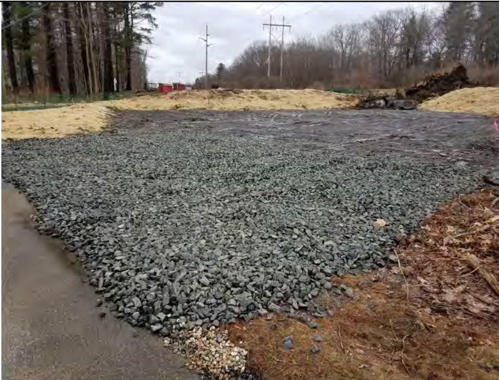
Photo 18: 04/07/2017, Litchfield: Map 29, Stone tracking pad at Str81 and Campville Road.
