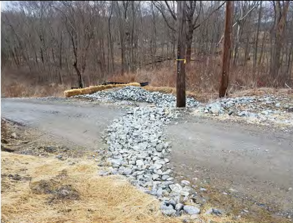
Photo 17: 04/07/2017, Litchfield: Map 26, waterbar to temporary sediment basin/trap.
