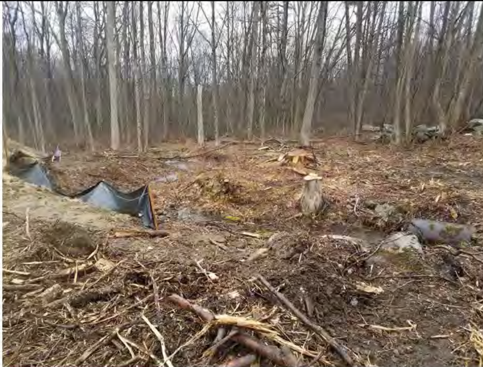
Photo 9: 3/31/2017, Litchfield: Map 29, Str83 abutting W-F4 and S-F2, failing E&S.
