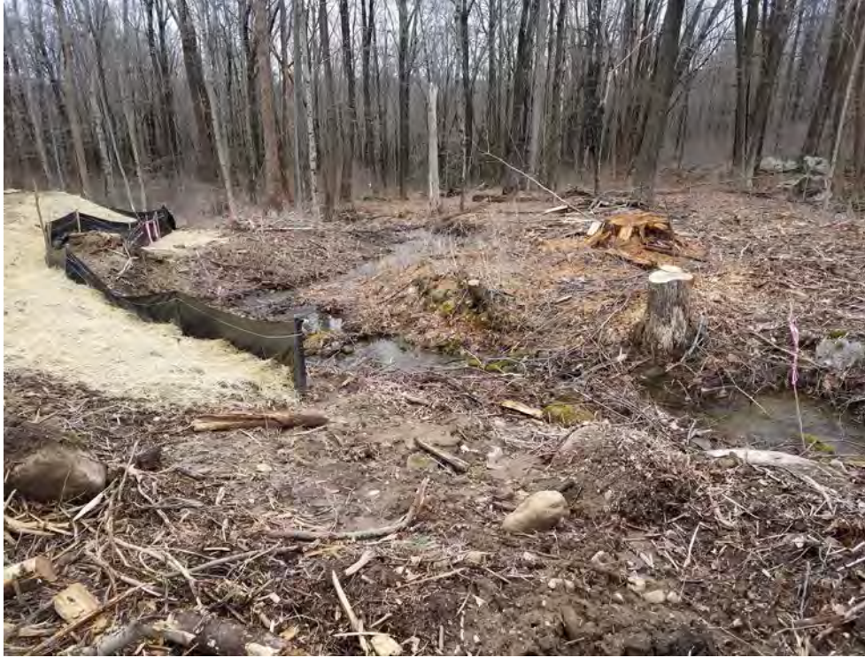
Photo 21: 04/07/2017, Litchfield: Map 29, E&S controls at Str83 and W-F4/S-F2.
