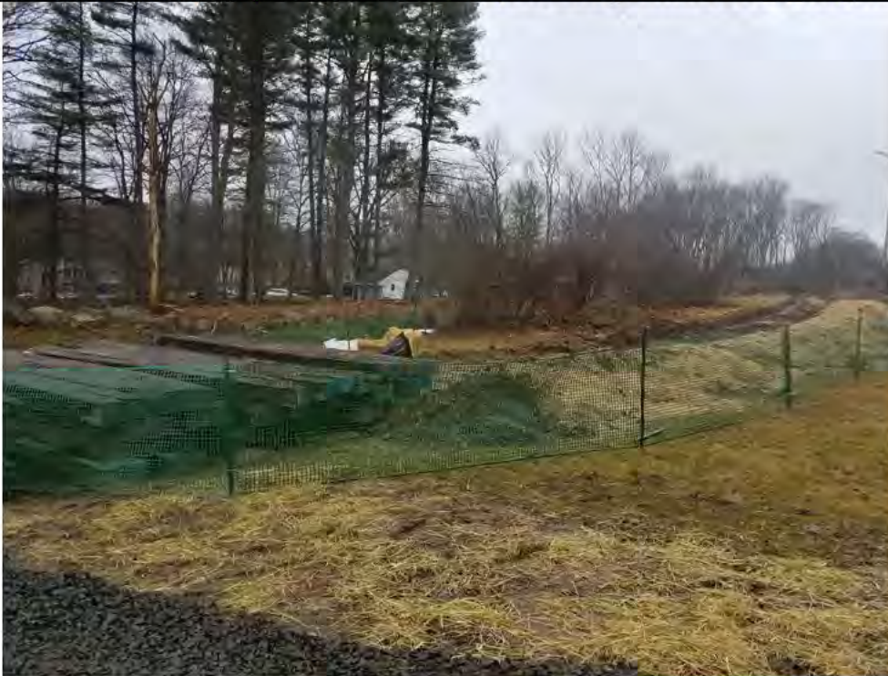
Photo 2: 3/31/2017, Litchfield: Maps 28 & 29, access road to Str80 abutting private driveway.
