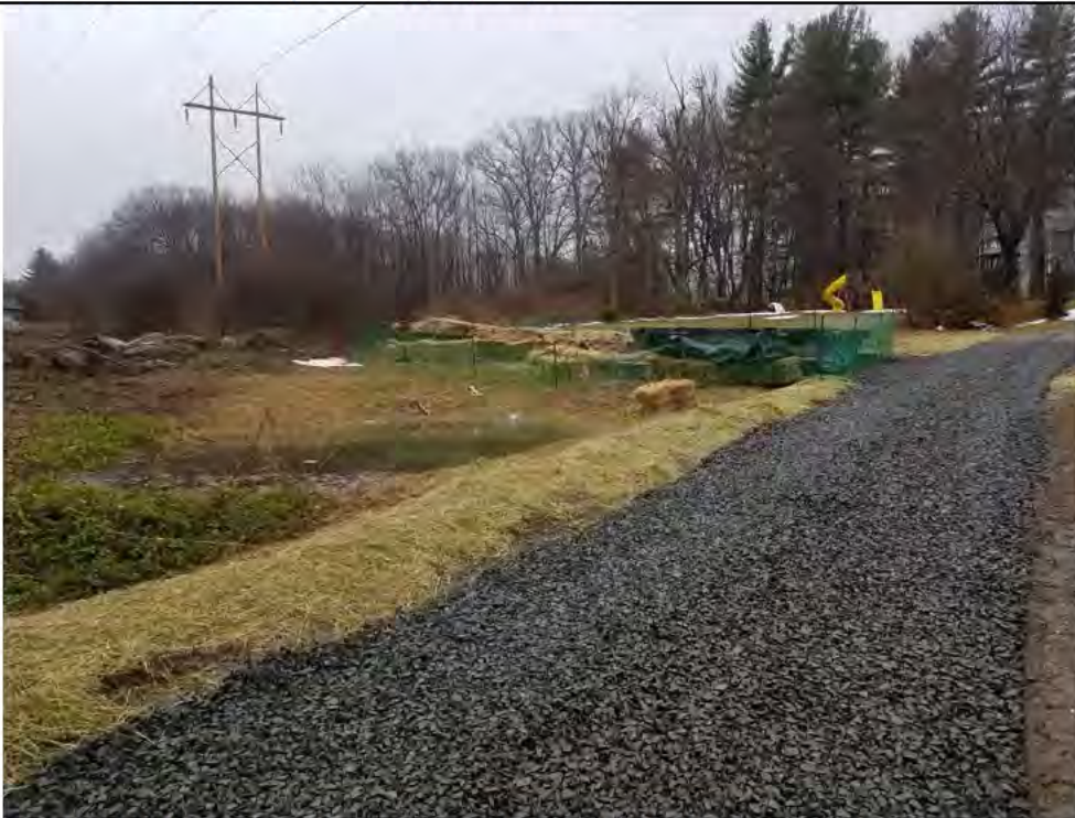
Photo 4: 3/31/2017, Litchfield: Maps 28 & 29, access road to Str80 abutting private driveway, repairs made to driveway after surface water runoff erosion was reported by property owner.
