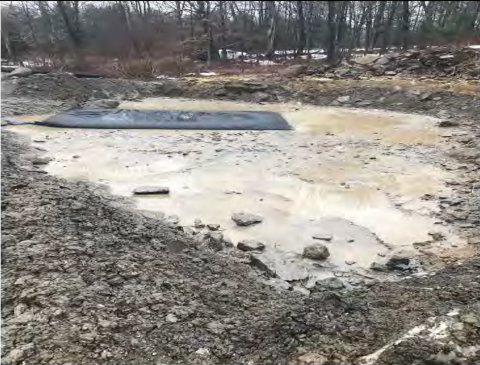
Photo 14: 3/31/2017, Harwinton: Map 35, Str96 abutting W-G1, silt bag and dirt berm, area of release (Photo provided by Matt Davison).
