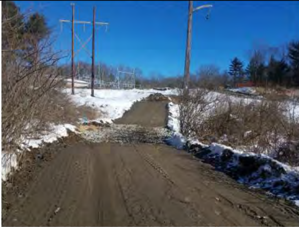
Photo 1: 2/17/2017, Harwinton, Map 35: Hard bottom crossing at S-G3 between Str97 and Str96.
