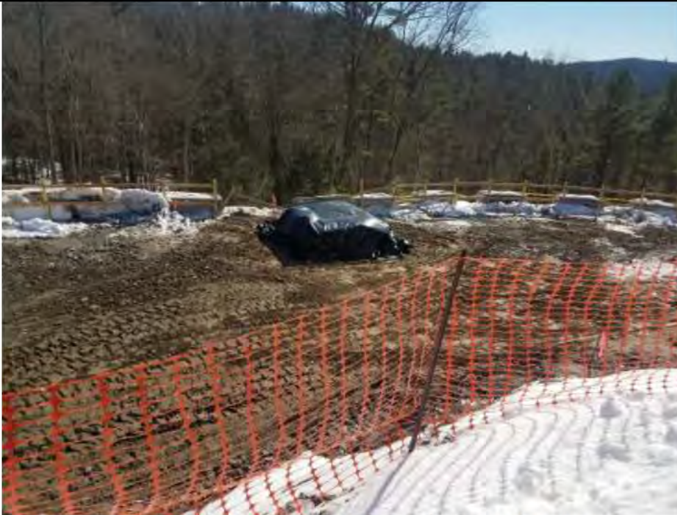
Photo 3: 2/17/2017, Harwinton, Map 32: Construction of Str88, poured concrete foundation.
