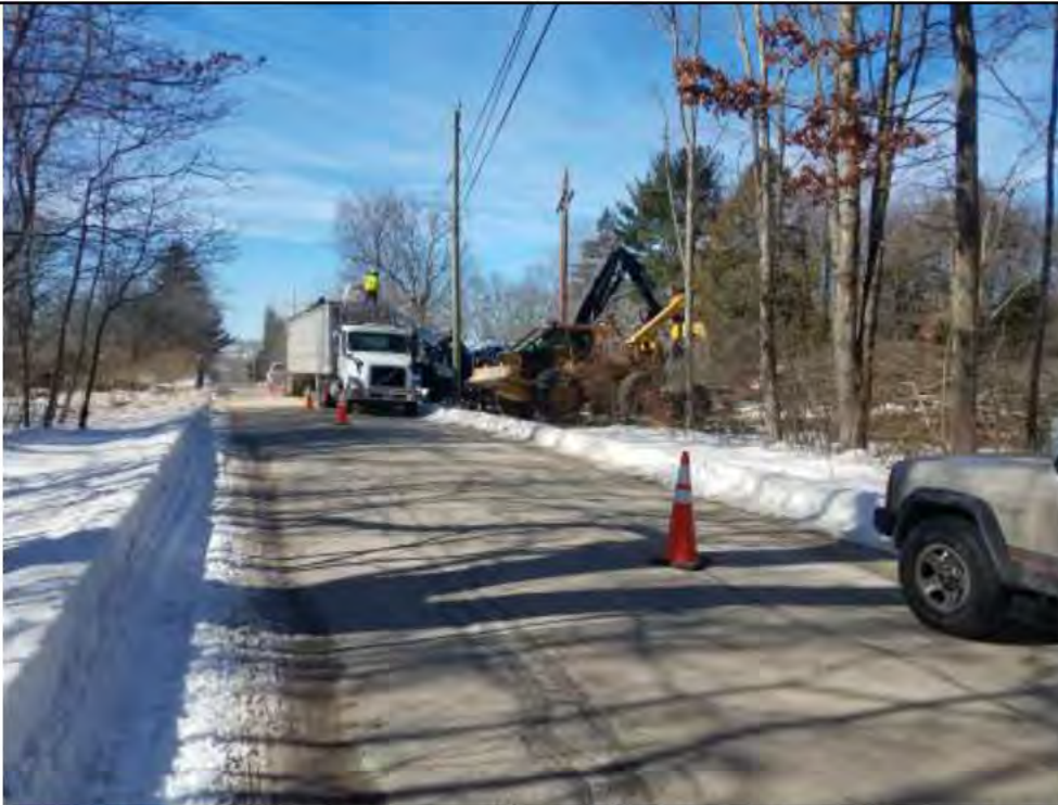
Photo 4: 2/17/2017, Litchfield, Map 26: Wood chipping at area of mechanical clearing between Str74 and Str77.
