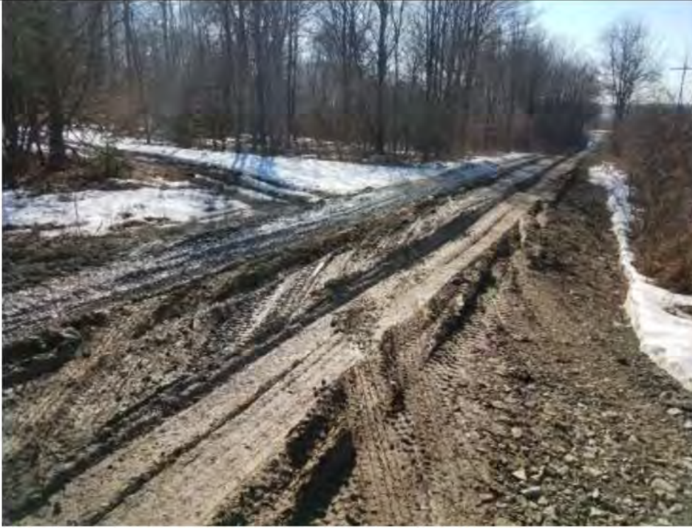
Photo 11: 2/23/2017, Watertown, Map 9A: Soft ground conditions, tire rutting occurring.
