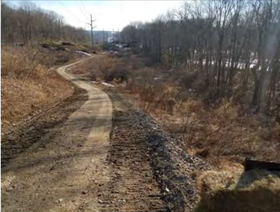
Photo 17: 2/23/2017, Litchfield, Map 26: Access road below water bar and plunge pool upland of W-E2, DVP-E2-1 and DVP-E2-2.
