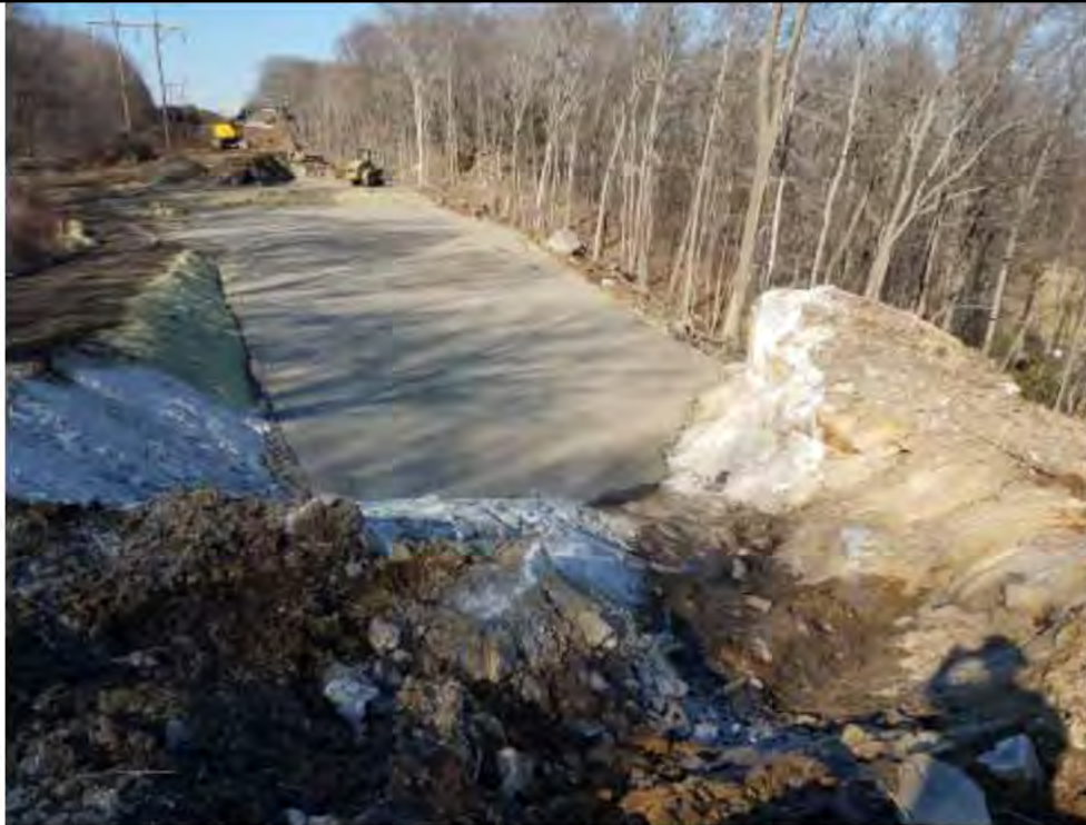
Photo 15: 2/23/2017, Watertown, Map 10: Str27 and Str28 pad construction.
