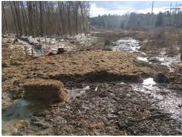
Photo #35:1/26/17, Harwinton- Access road to Str97, surface water runoff to wetlands W-G1
