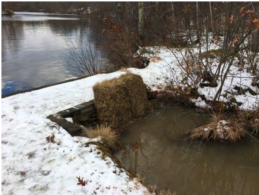
Photo #42: Thomaston- Morton Property- Morton Pond, implementation of E&S controls
