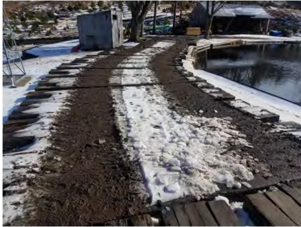
Photo #28:1/26/17, Thomaston- Robert K. & Jean R. Morton Property(41033, Map 21), access road to Str58-Str60, timber mats
