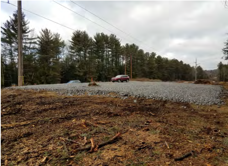
Photo #4:1/19/17, Harwinton: Str91 pad completed
