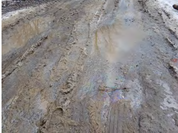
Photo #37:1/26/17, Harwinton- Campville Substation access road, petroleum release to ground
