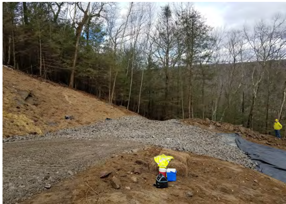
Photo #14:1/19/17, Litchfield: Access road to Str86, Str3236, Str3171 construction
