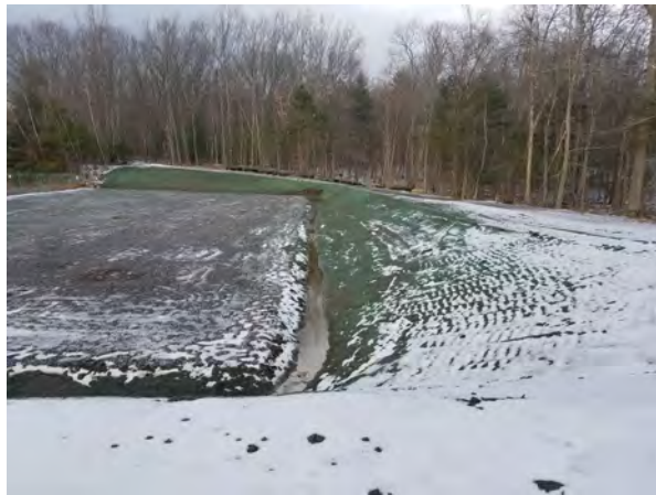
Photo #32:1/26/17, Harwinton- Campville Substation expansion, swale and surface water drainage conditions
