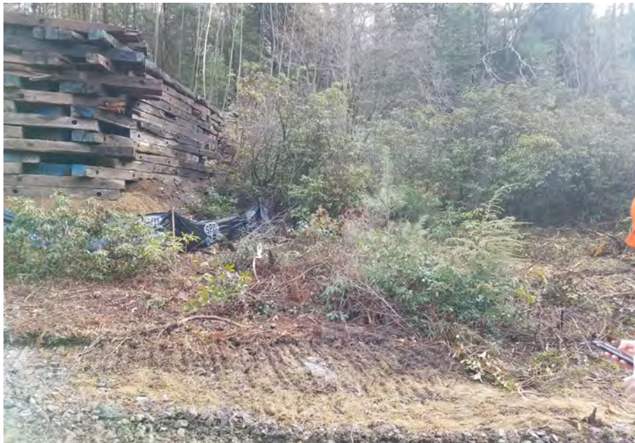
Photo #10: 1/19/17, Harwinton: W-F13 southwest corner of Str90 pad
