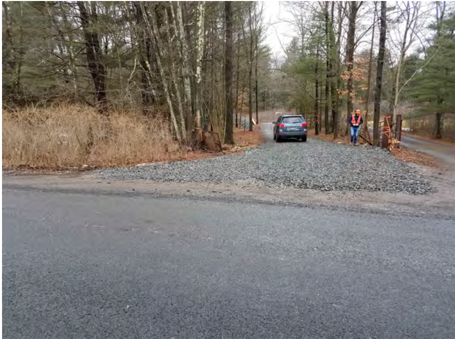
Photo #1: 1/19/17, Harwinton: Stone apron at access road entrance to Str94-Str88
