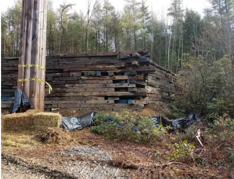
Photo #7: 1/19/17, Harwinton: Timber mat wall surrounding Str90
