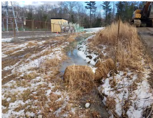
Photo #33:1/26/17, Harwinton- Campville Substation expansion, swale and surface water drainage conditions
