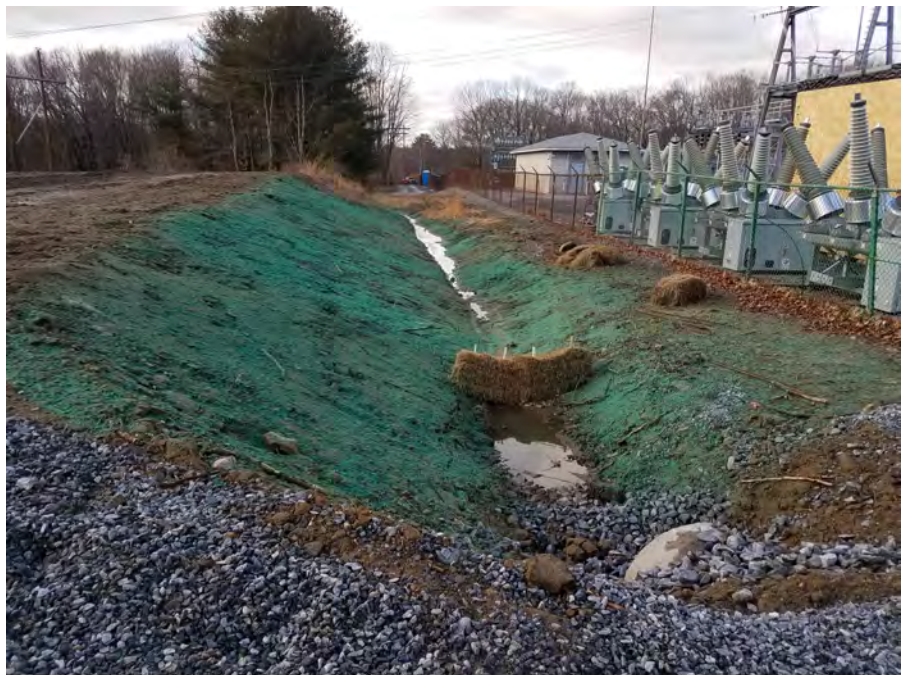
Photo #18:1/19/17, Harwinton: Campville Substation Expansion, drainage swale south side of Substation
