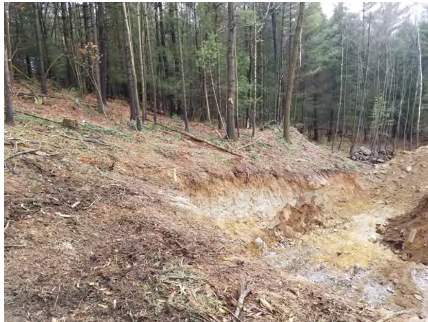
Photo #6:1/19/17, Harwinton: Str90 Pad construction prep
