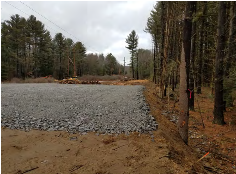
Photo #2: 1/19/17, Harwinton: Str92 pad, completed
