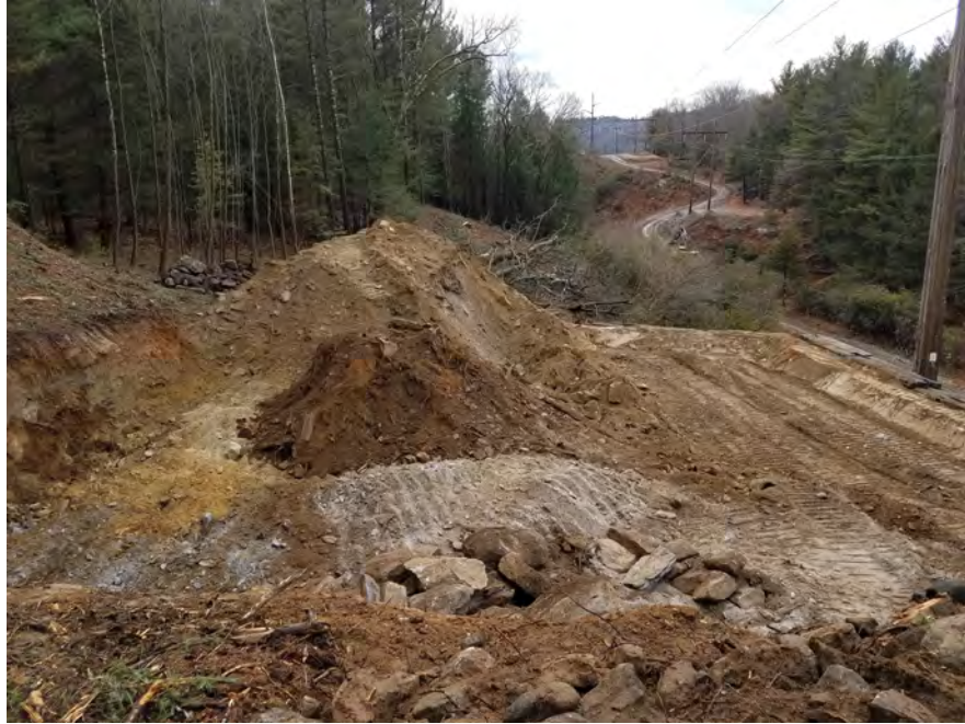
Photo #5:1/19/17, Harwinton: Str90 pad construction, soil and rock removal
