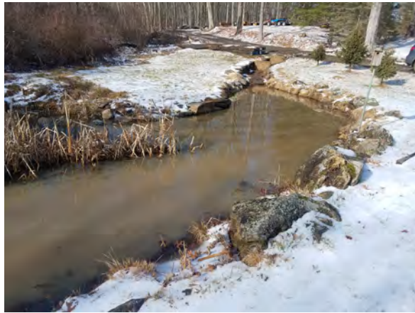
Photo #26:1/26/17, Thomaston- Robert K. & Jean R. Morton Property(41033, Map 21), access road to Str58-Str60, run off to Morton Pond
