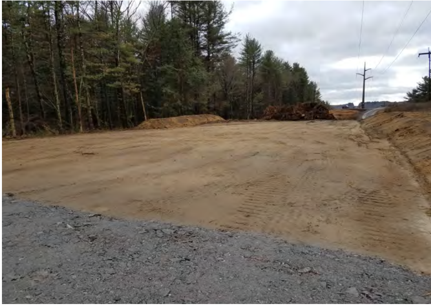
Photo #3 1/19/17, Harwinton: Pull pad between Str92 and Str91 construction:
