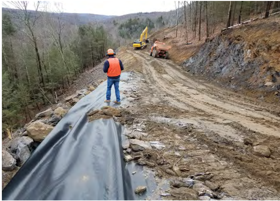
Photo #13:1/19/17, Litchfield: Access road to Str86, Str3236, Str3171 construction
