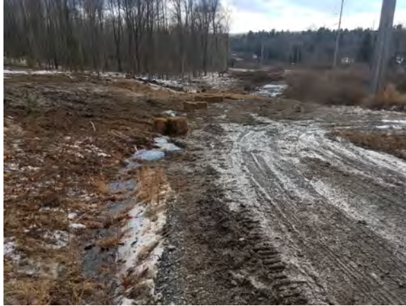
Photo #34:1/26/17, Harwinton- Access road to Str97, surface water runoff to wetland W-G1
