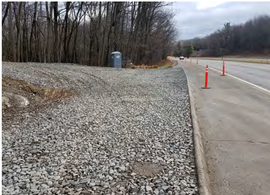
Photo #16:1/19/17, Litchfield: Access road to Str86, Str3236, Str3171, Rt 8N entrance/exit apron tracking pad
