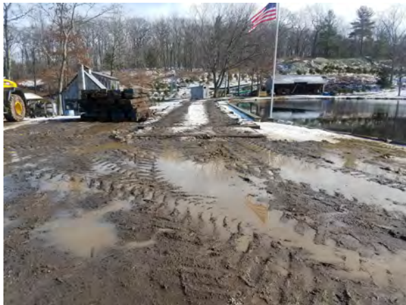
Photo #27:1/26/17, Thomaston- Robert K. & Jean R. Morton Property(41033, Map 21), access road to Str58-Str60, run off to Morton Pond
