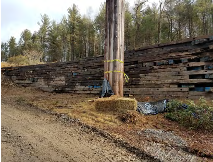
Photo #8: 1/19/17, Harwinton: Timber mat wall surrounding Str90
