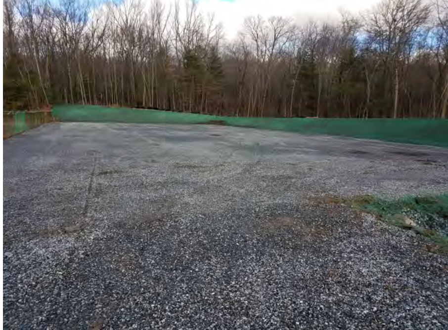
Photo #17:1/19/17, Harwinton: Campville Substation Expansion, hydroseeding embankment
