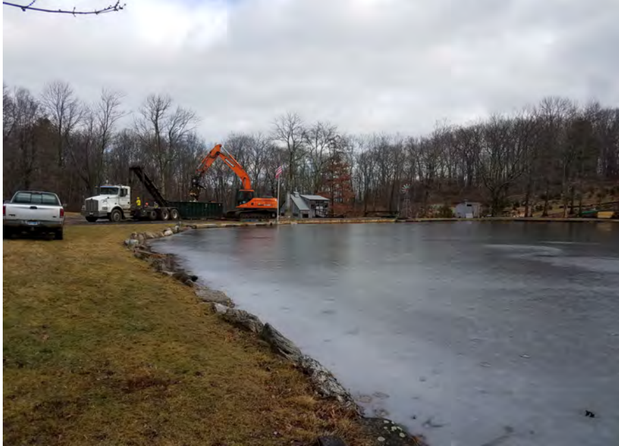
Photo #11:1/19/17, Thomaston: Timber mat placement at watercourse/Morton Pond
