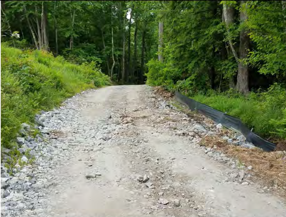
Photo 2: 06/15/2018, Watertown: Map 13, Wetland W-C18, timber mats removed, stone access road graded, and silt fence repaired. No visible impacts to wetland observed.
