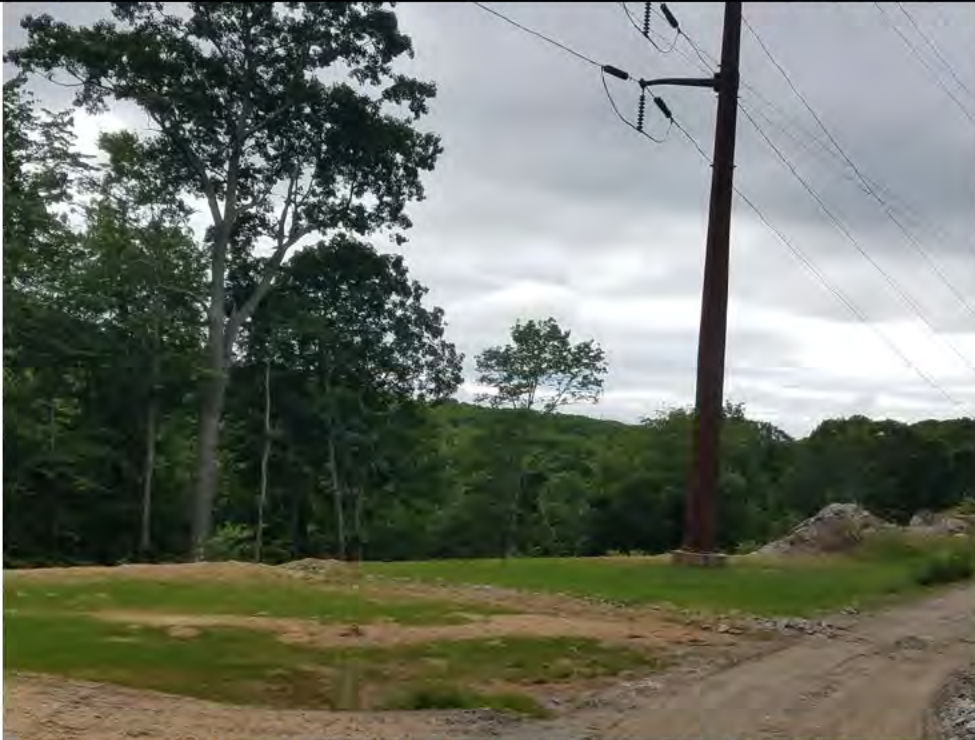
Photo 8: 06/15/2018, Watertown: Map 10, Str28/Str27 work pads, veg growth following hydroseed application approximately 2 weeks prior after regrading and drainage improvements. Access road graded and silt fence removed (as instructed) abutting wetland W-C3 (to the left, out of view in photo).
