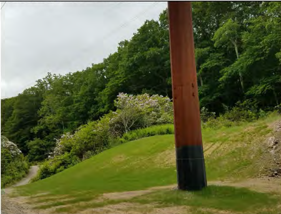
Photo 6: 06/15/2018, Watertown: Map 12, Str33, upland slope and pad, veg growth following hydroseed application approximately 2 weeks prior.
