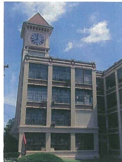
Seth Thomas Building Photo by: Patrick Martin
