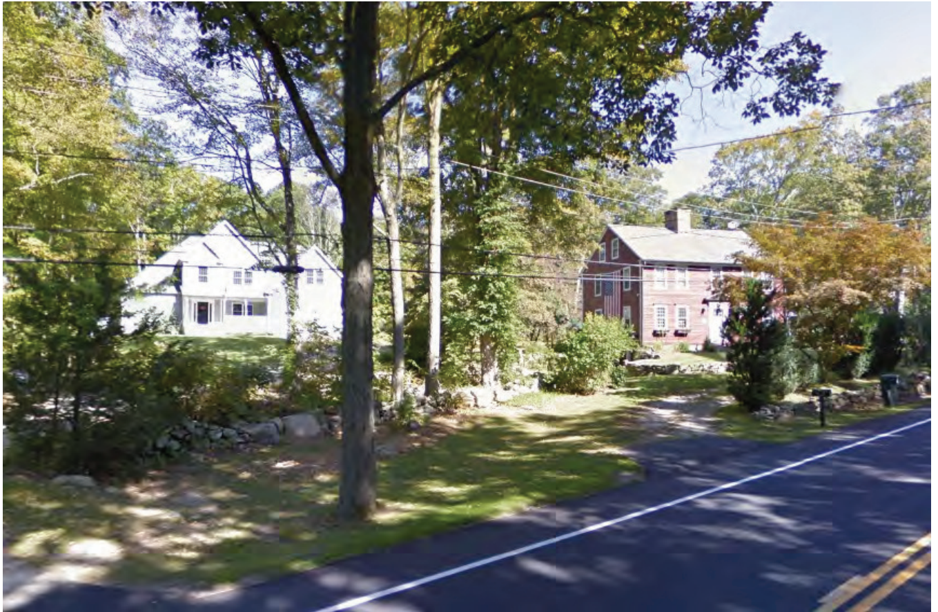
Photograph 13. View looking northeast towards 365 Boston Post Road (ca. 1770) from Boston Post Road. Assessed from Google.com 7/8/2015.
