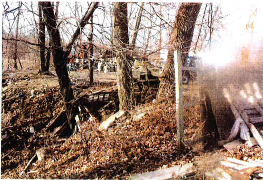
PHOTO NO. 2 – SITE HAS BEEN FILLED OVER THE YEARS VIEW OF THE SOUTHERN SLOPE
