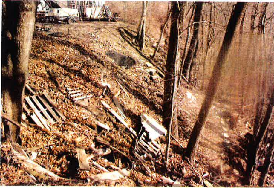
PHOTO NO. 1 – SITE HAS BEEN FILLED OVER THE YEARS VIEW OF THE SOUTHERN SLOPE
