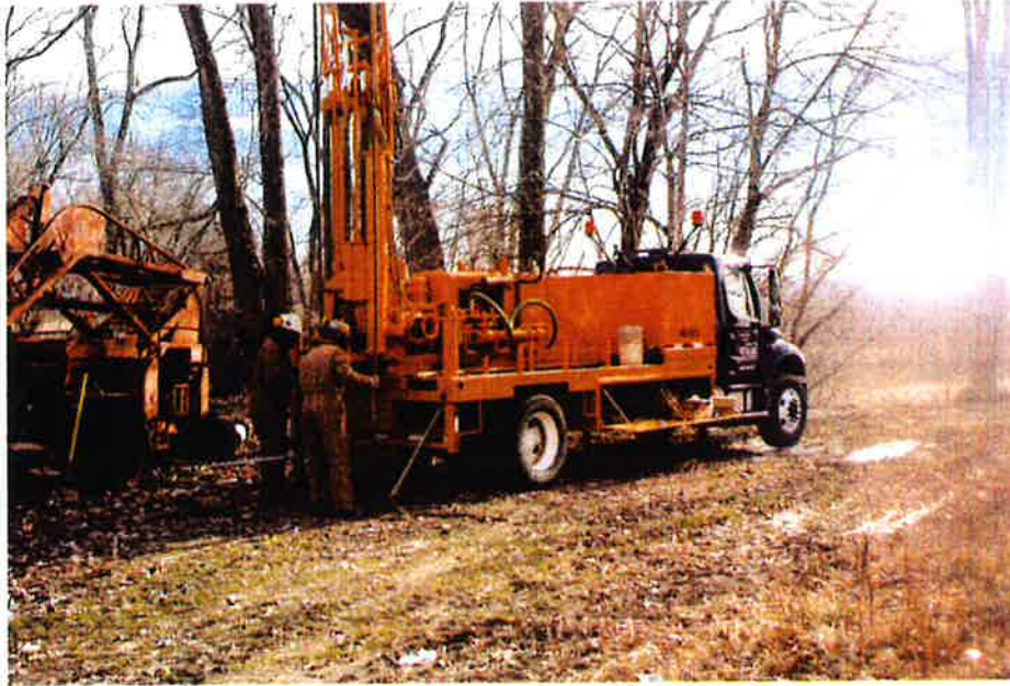
PHOTO NO. 3- DRILLING BORING AT CENTER OF TOWER
