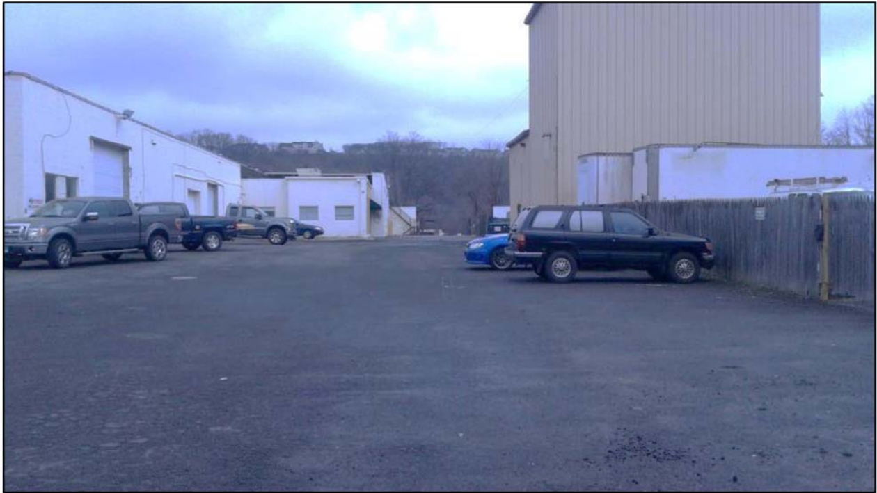
Photo 9. Overview photo of the proposed access road facing east.
