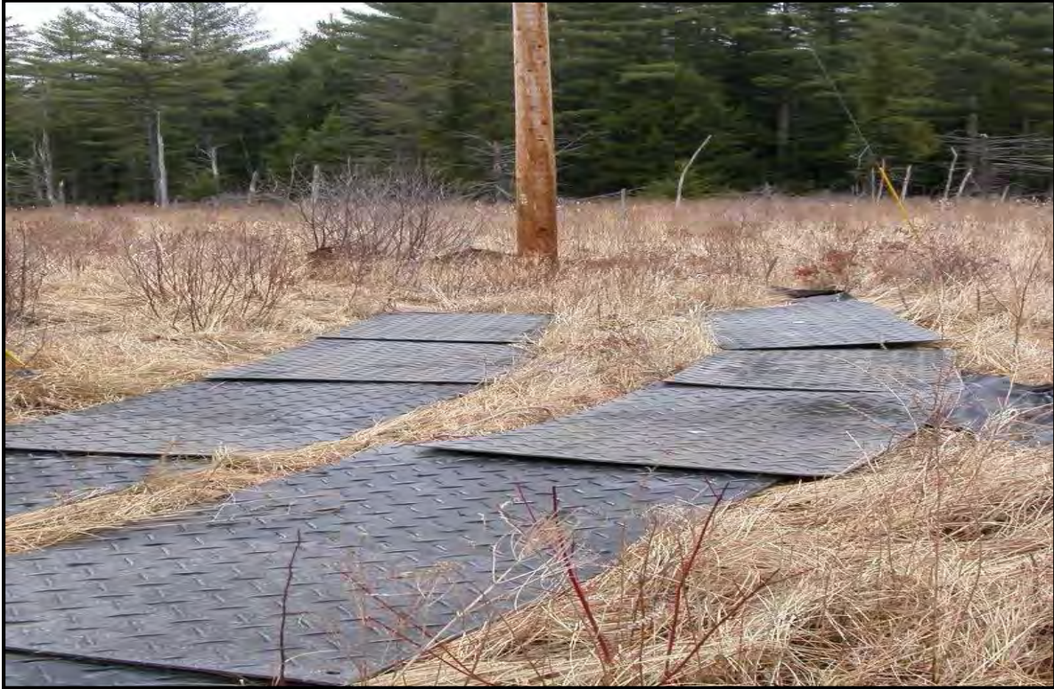
AlturnaMAT® tracks to utility pole in wetland.
