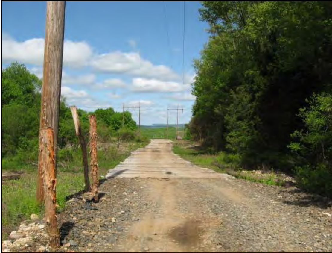
Construction mat access road.
