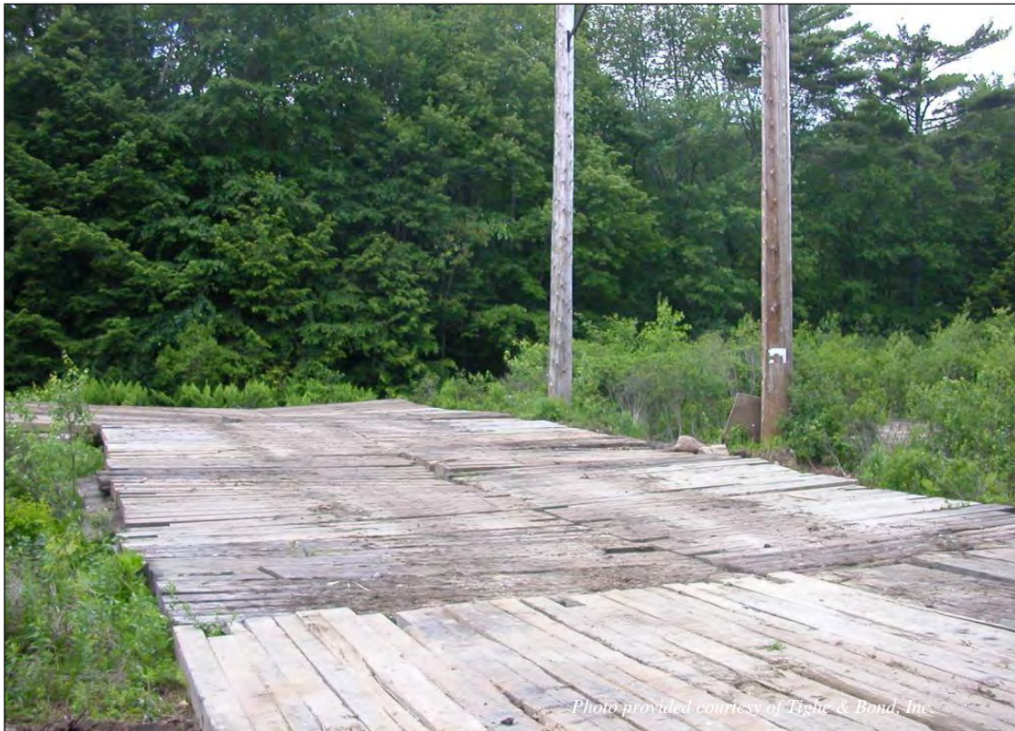
Construction mat wetland work-pad for de-energized work.
