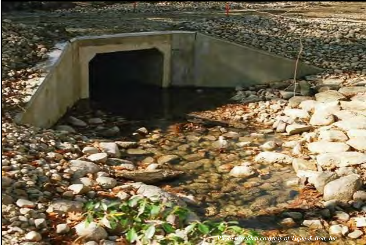
Embedded box culvert with wing walls.
