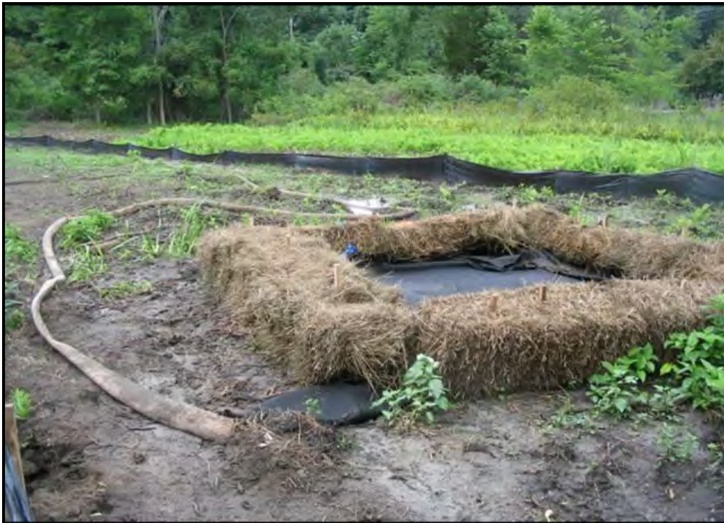
Dewatering to filter “sock” surrounded by hay bales.
