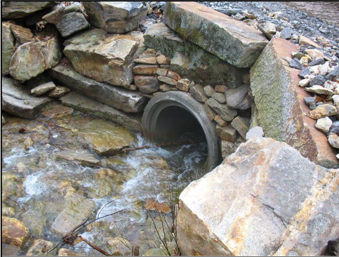
Culvert and riprap for stream crossing.
