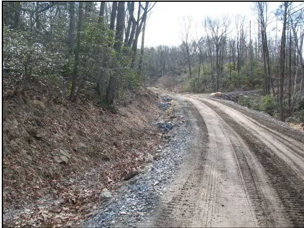
Stone check dams at construction site.
