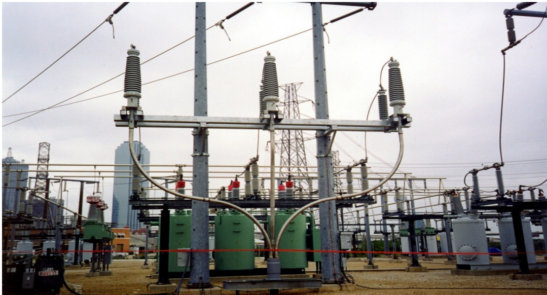
Figure H-9 Typical 115-kV HPFF Termination Structure
