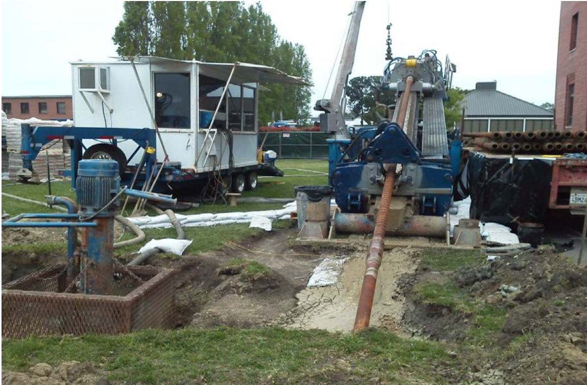
Figure H-6 Typical HDD Setup – Entry Location
