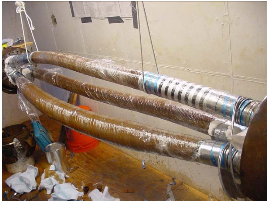
Figure H-8 Typical 115-kV HPFF Splice Assembly
