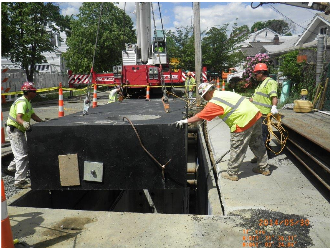
Figure H-4 Typical Splice Vault Installation
