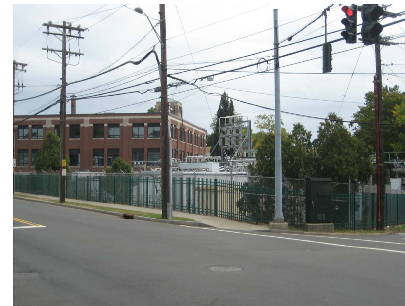
VIEW OF EXISTING FENCES AROUND SUBSTATION STEEL PICKET FENCE AND CHAIN LINK WITH BARBED WIRE FENCE TO BE REPLACED BY PERFORATED METAL FENCE
