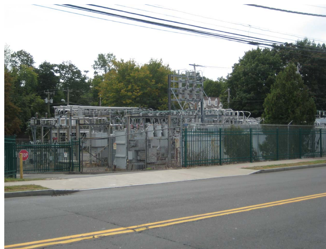
VIEW OF EXISTING FENCES AROUND SUBSTATION STEEL PICKET FENCE AND CHAIN LINK WITH BARBED WIRE FENCE TO BE REPLACED BY PERFORATED METAL FENCE
