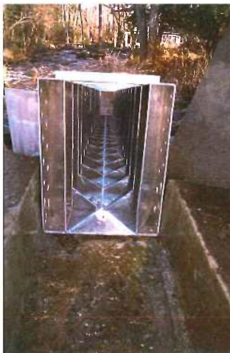
Fish bypass ladder installed on Parker River Dam, Byfield, MA, 2000. NOAA Restoration Center Community-based Restoration Project. Photo Credit: NOAA photo library.
