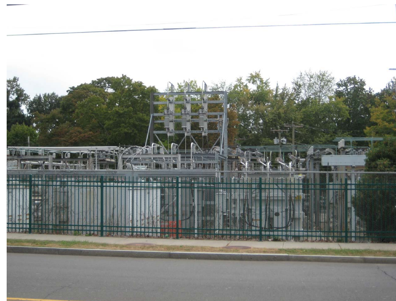
VIEW OF EXISTING FENCES AROUND SUBSTATION STEEL PICKET FENCE AND CHAIN LINK WITH BARBED WIRE FENCE TO BE REPLACED BY PERFORATED METAL FENCE
