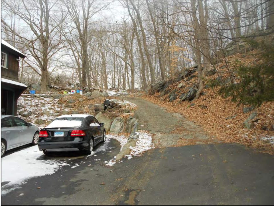
Photo 19. Overview photo of the western portion of the proposed access road facing north (note pavement and concrete in this area).
