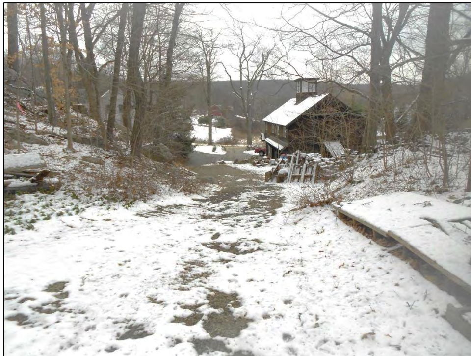
Photo 18. Overview photo of the western portion of the proposed access road facing northeast (note erosion and modern trash throughout the area).
