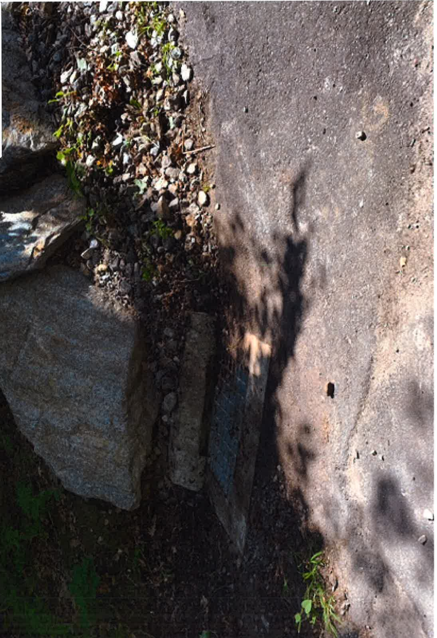
Area Around Access Drive Catch Basin
