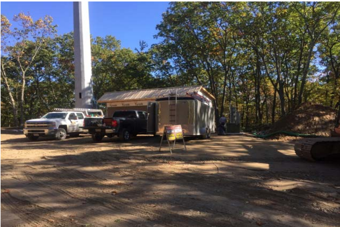
Photo 6: View of compound and tower looking south.
