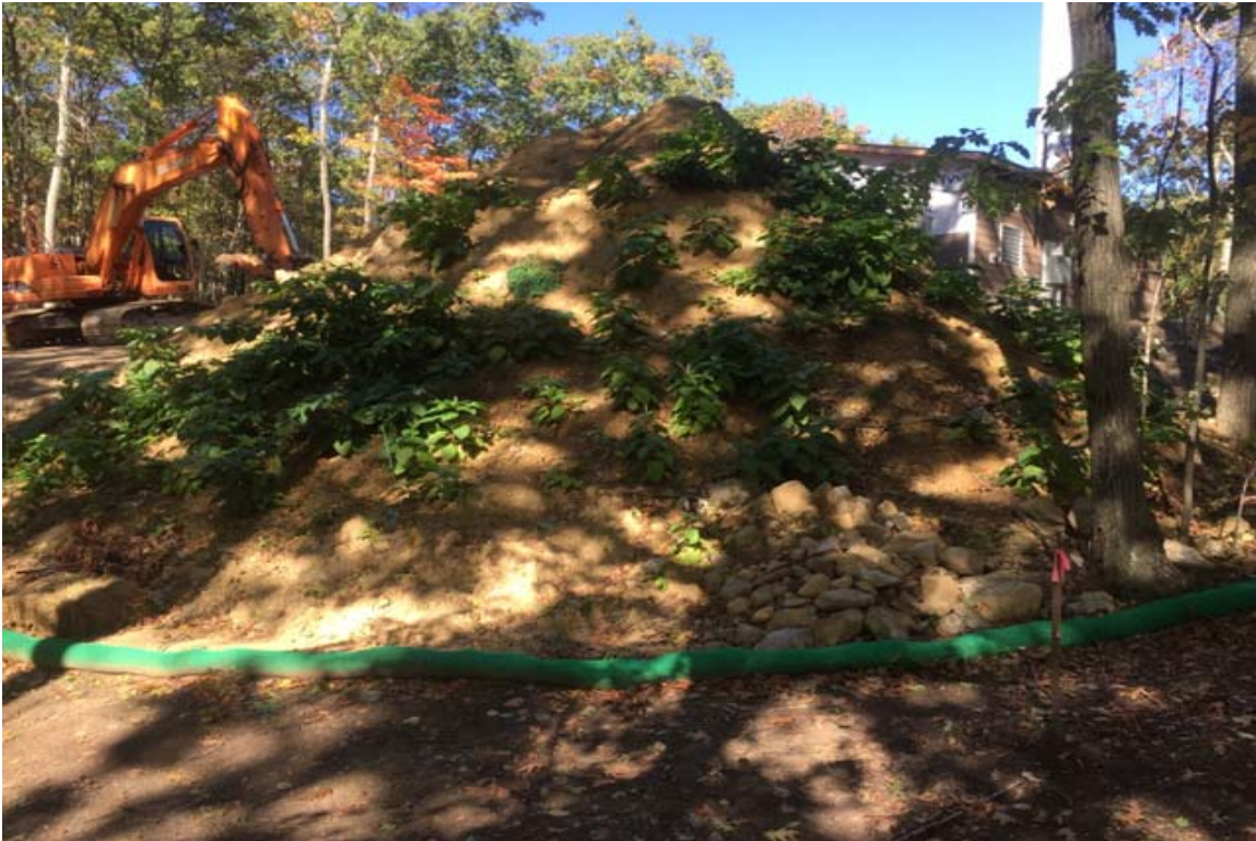
Photo 5: View of temporary soil stockpile (CA#11) looking northeast.
