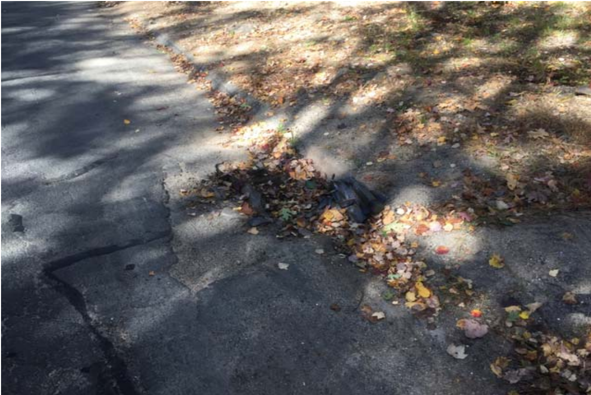
Photo 1: View of CA#8, clean accumulated sediment in silt sock, looking north.
