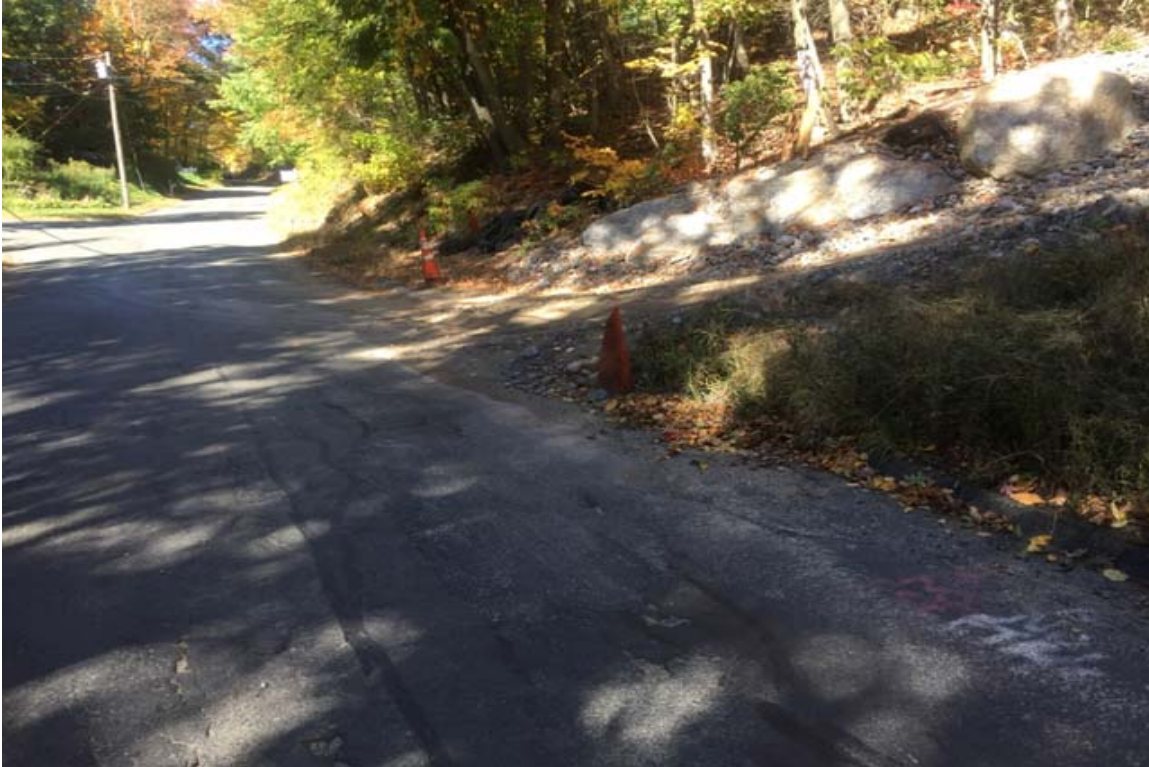
Photo 3: View of CA#10, clean up driveway material from Keegan Road, looking north.
