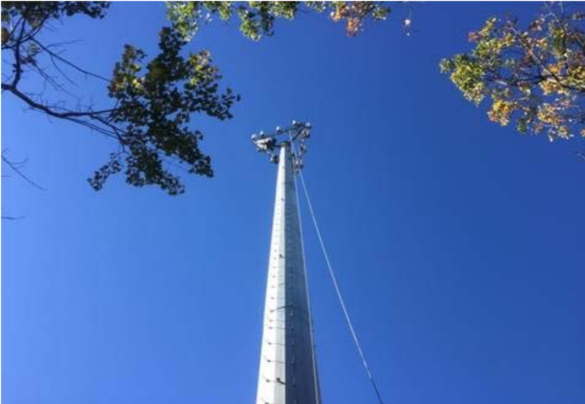
Photo 7: View of tower.
