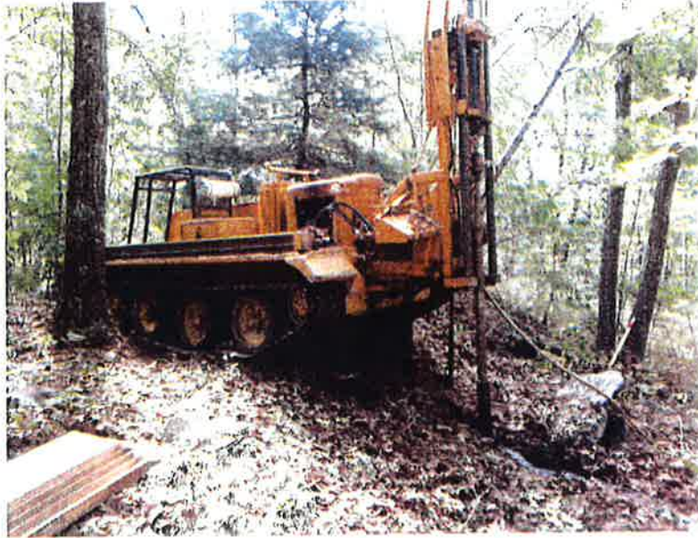
DRILLING BORING No. 1
