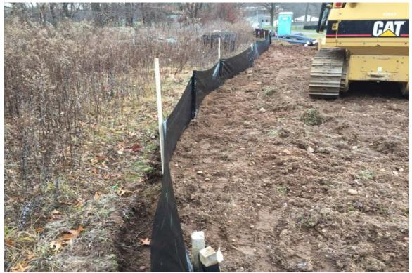
Photo 5: View of fixed buried silt fence looking southeast.
