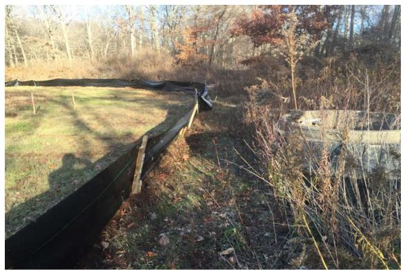
Photo 4: Corrective Area #2 - view of broken stakes looking north.
