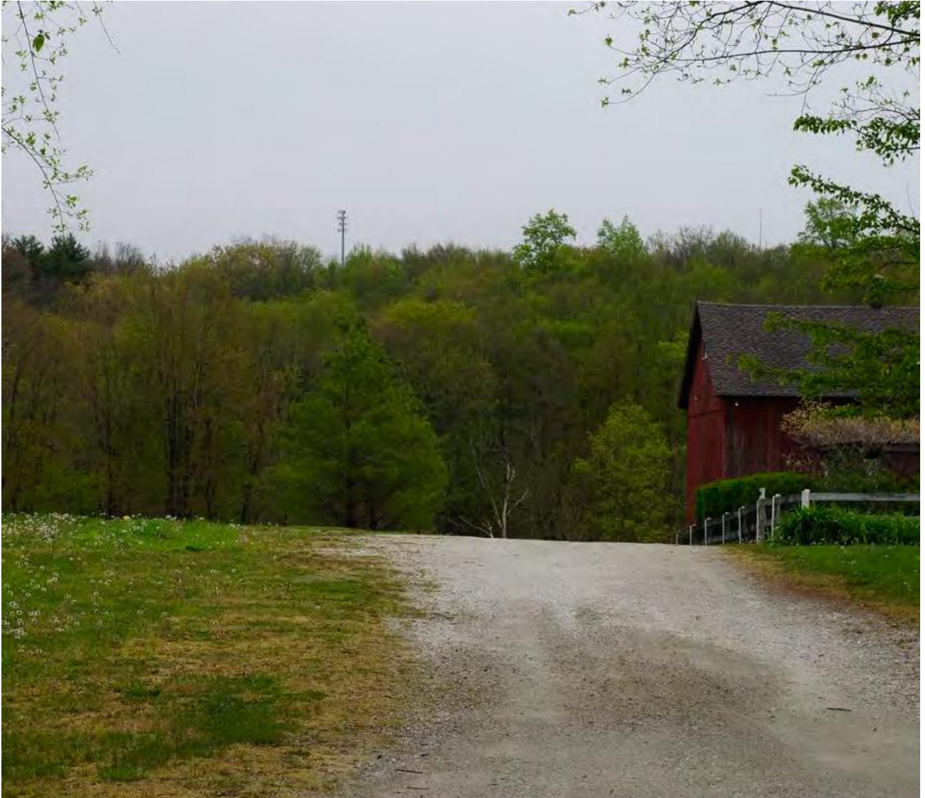
Photo simulation of proposed 160-foot tower. Visibility map location 6. Adjacent to #35-39 Hatch Road, 0.5 miles from site. (AT&T 1, Tab 5)
