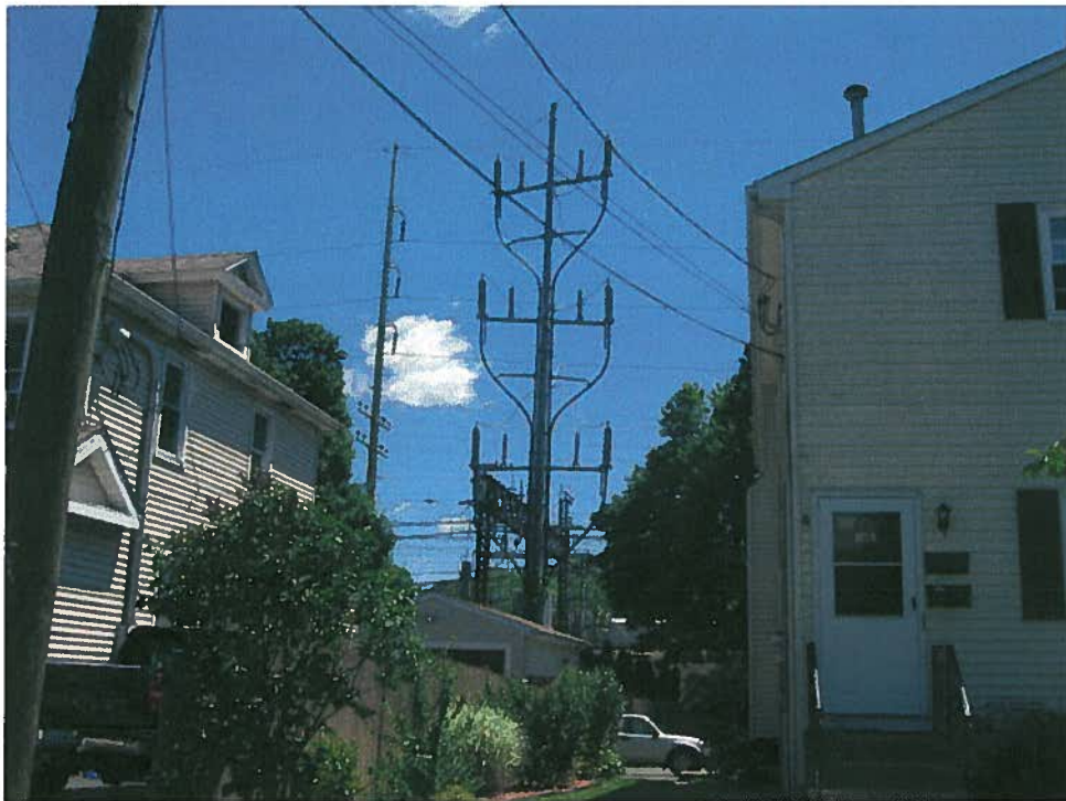
Culloden Rd – Looking at OH/UG Transition into Glenbrook S/S
