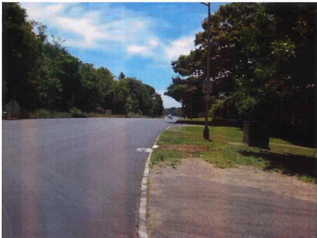
A photograph looking south on Martin Luther King, Jr. Drive from the access driveway
