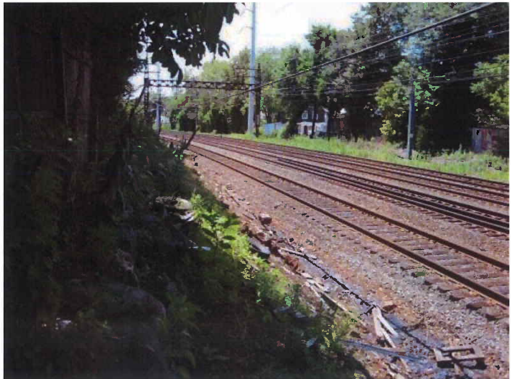
A photograph looking south along the MetroNorth ROW from the southern parcel
