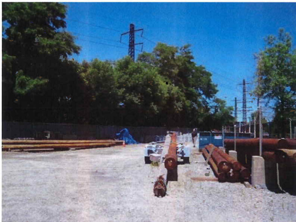
A photograph taken from inside the northern storage area looking northwest
