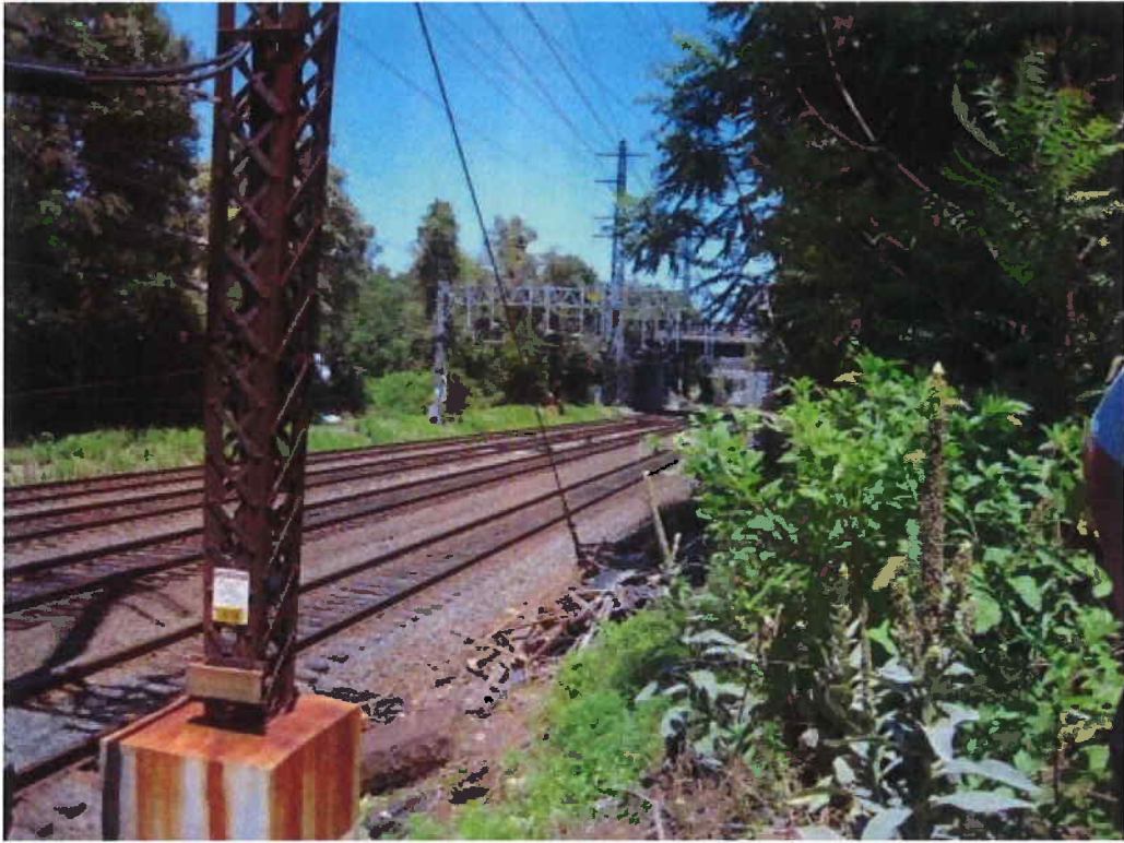
A photograph looking north along the MetroNorth ROW from the southern parcel
