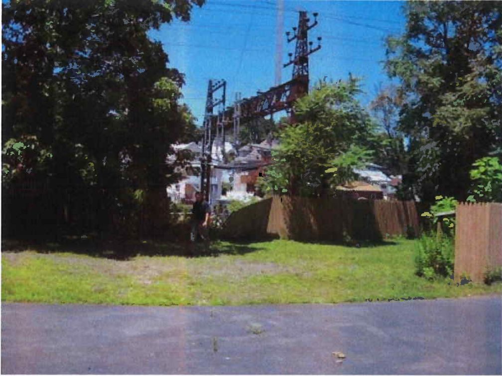
A photograph taken from the southern parcel looking west toward the MetroNorth ROW
