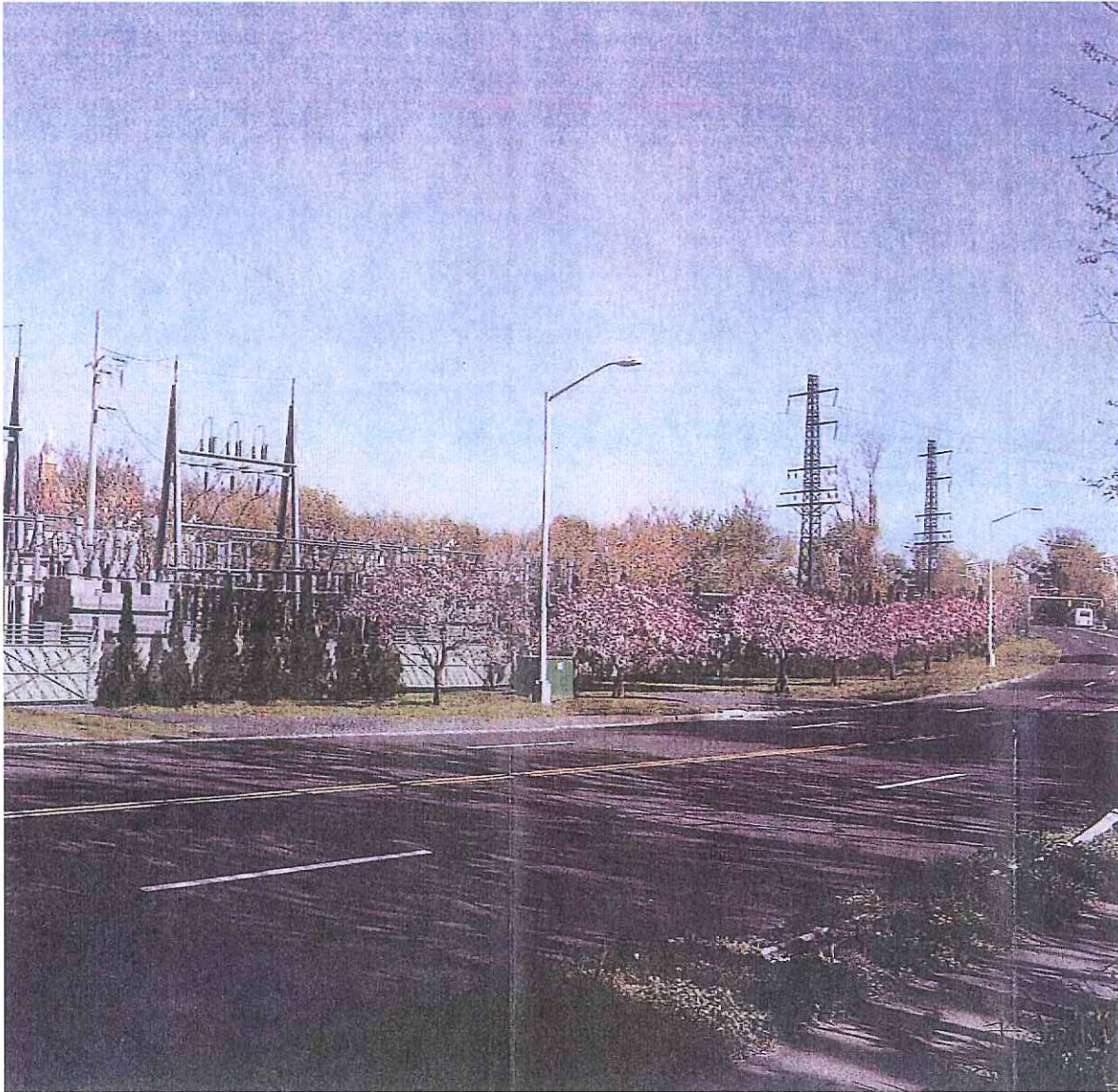
Attachment 5: Photo-simulation of Proposed Substation as viewed from Dr. Martin Luther King, Jr. Drive
