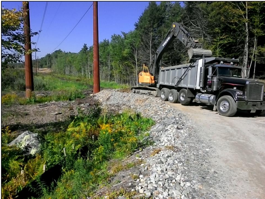
Photo #2: Removal of access road at Str 307. (9/18)
