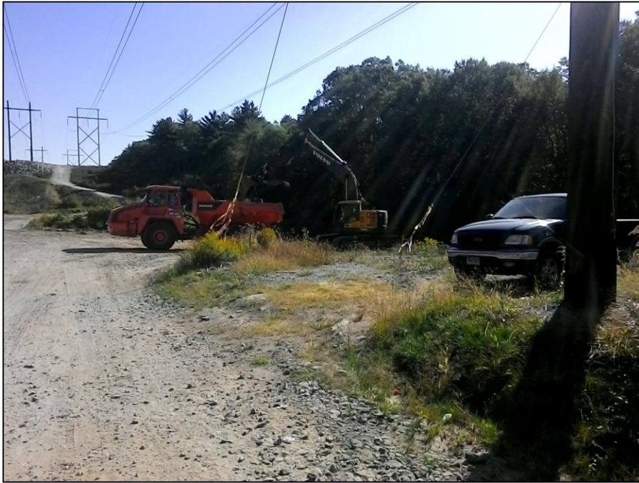
Photo #1: Stone removal at Str 337. (9/18)
