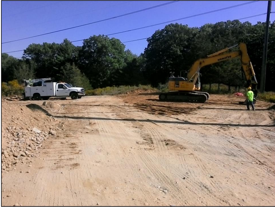
Photo #3: Earthwork at Str 254. (9/18)
