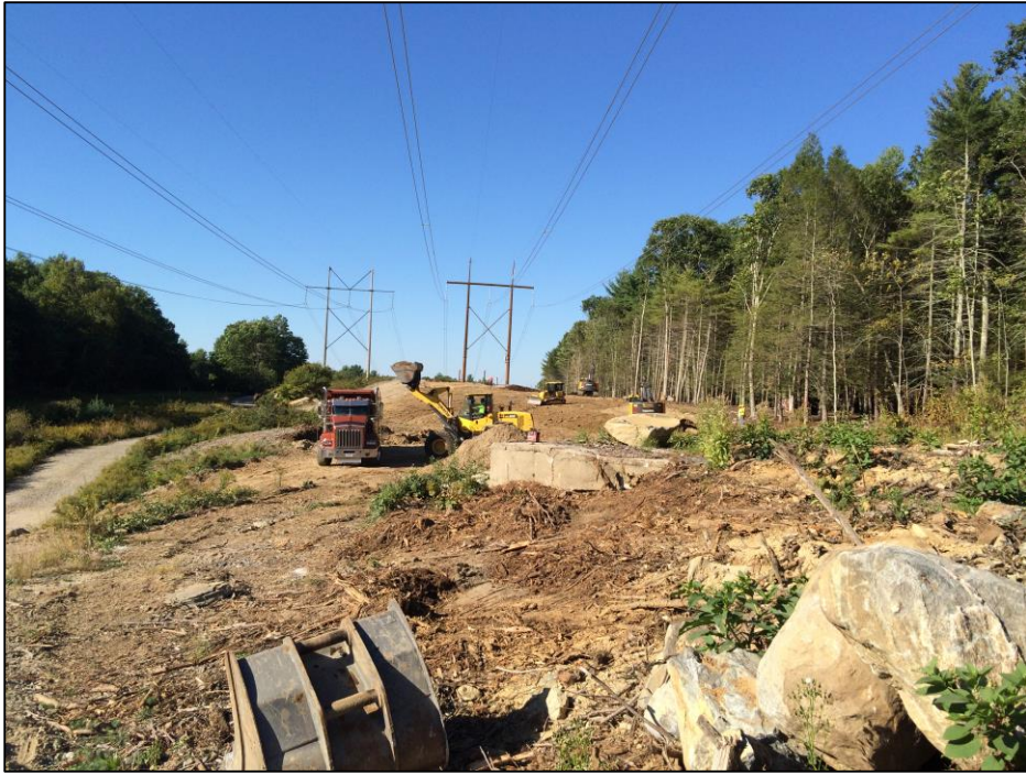
Photo #11: Re-grading and general earthwork at Str 308 as part of restoration operations. (9/24)
