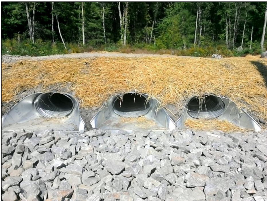
Photo #6: str 154 culvert seeded and temporarily stabilized with straw. (9/18)
