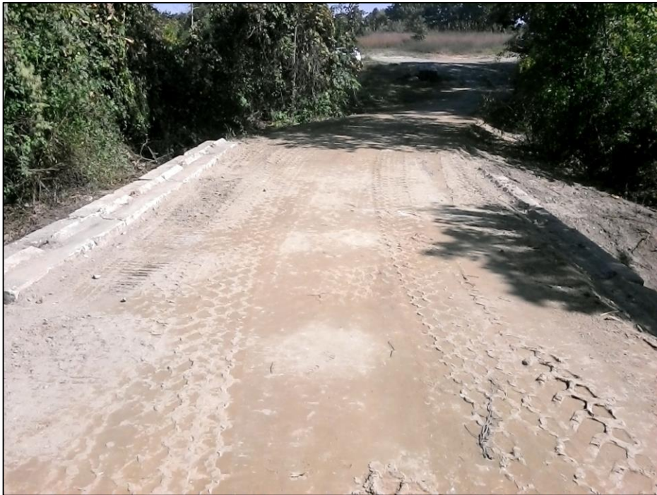
Photo #4: Day Street culvert installed but awaiting temporary stabilization. (9/18)
