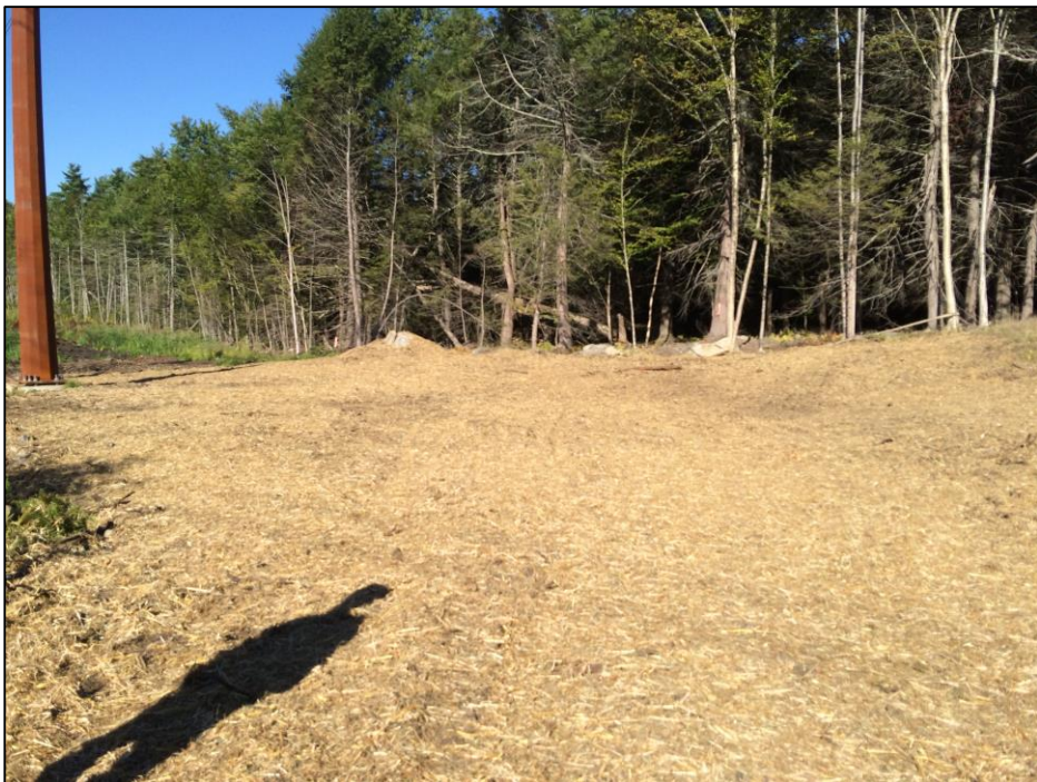
Photo #10: Str 307 seeded and temporarily stabilized with straw. (9/24)
