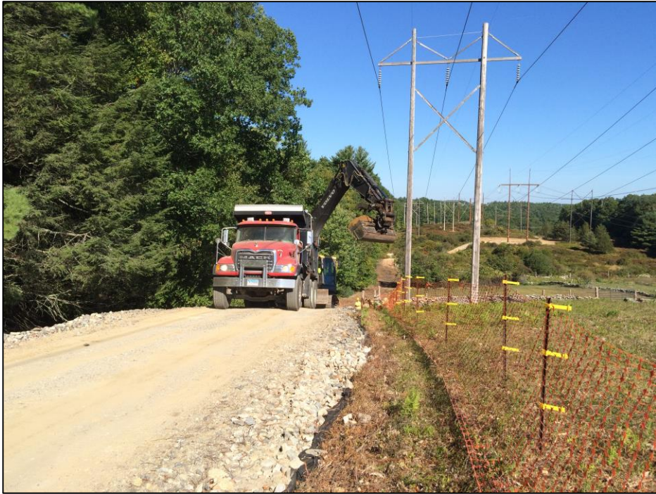
Photo #9: Str 253 access road removal. (9/24)
