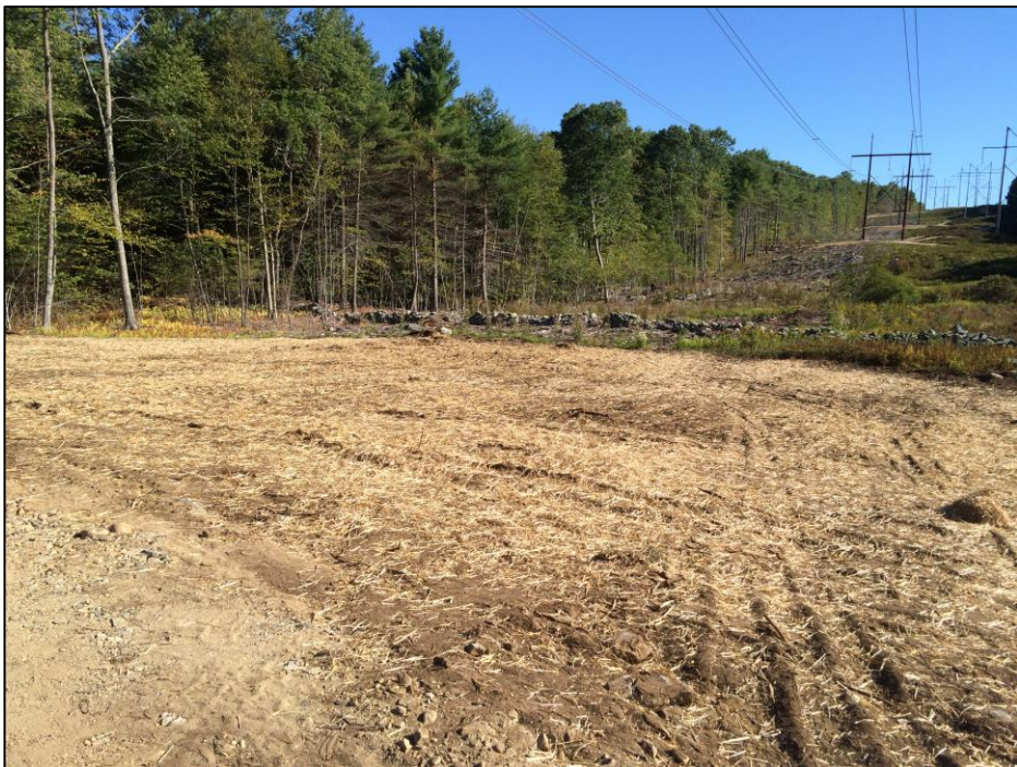
Photo #12: Str 331 seeded and temporarily stabilized with straw. (9/24)
