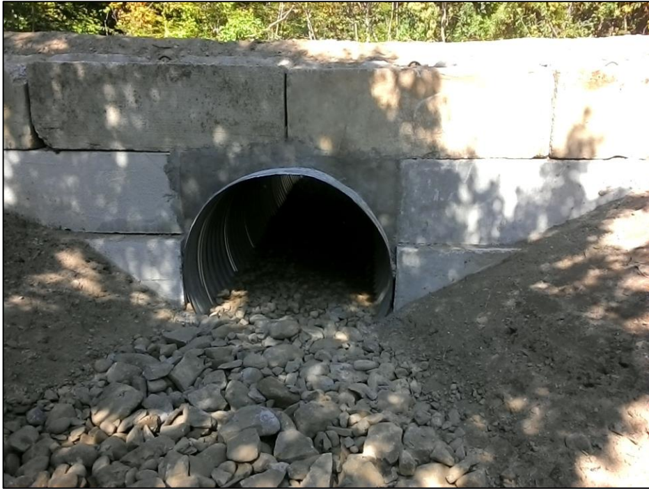
Photo #5: Day Street culvert outfall. (9/18)
