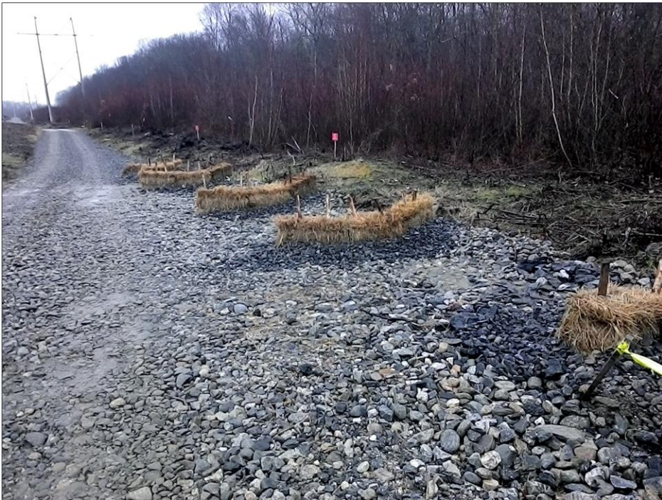
Photo #2: Check-dams functioning according to BMP manual down line of Str 157.
