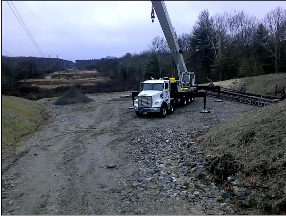
Photo #1: Crew preparing to clean up Str 168 for holiday shutdown.
