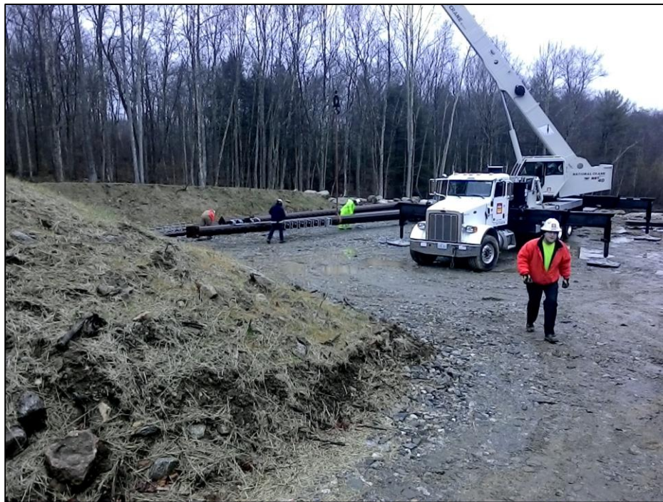
Photo #4: Crew preparing for Str 160 erection.
