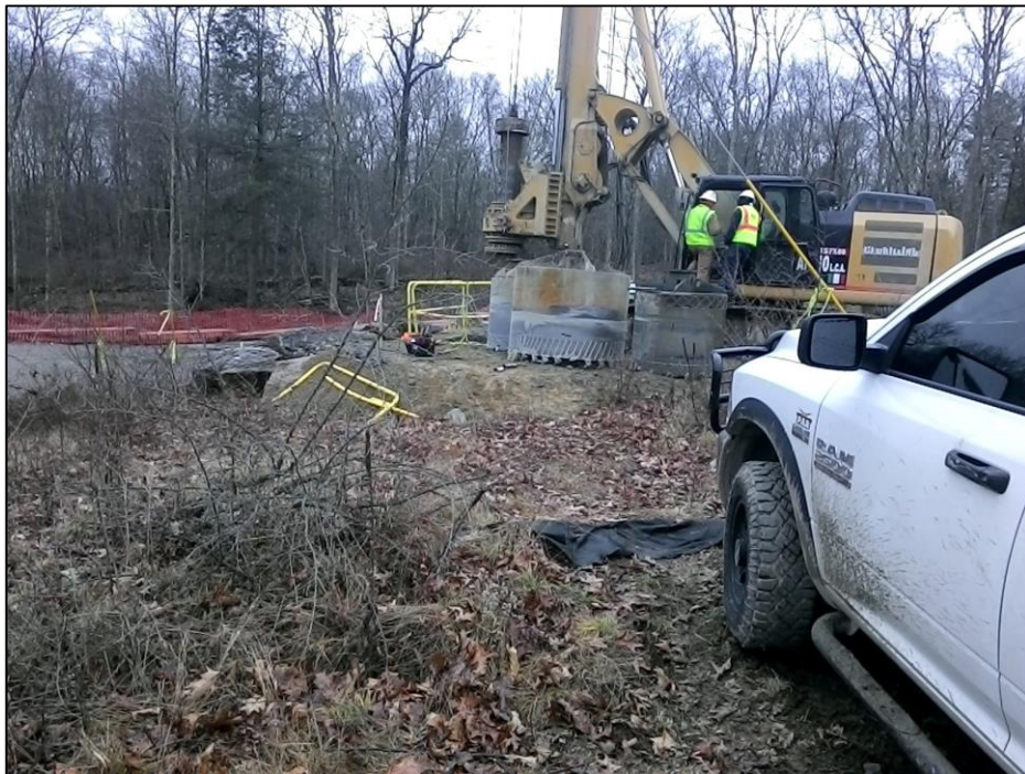
Photo #8: Rock coring for Str 183.
