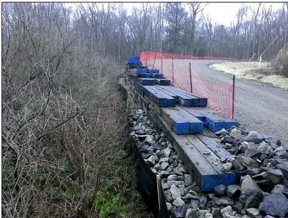
Photo #10: Erosion Controls and timber mat retaining wall down-line of Str 183.
