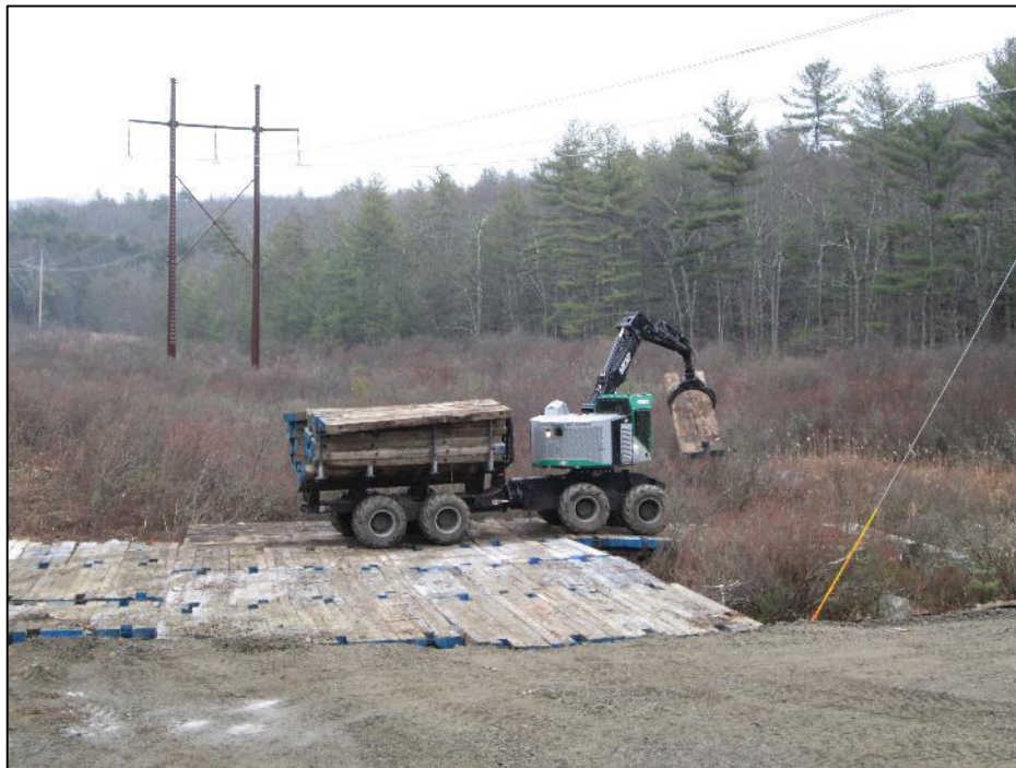
Photo #6: Building of Str pad 305 with timber mats in wetland. (12/16)
