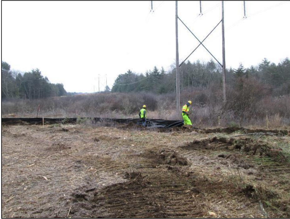
Photo #1: Observed installation of silt fence at Str 317. (12/16)
