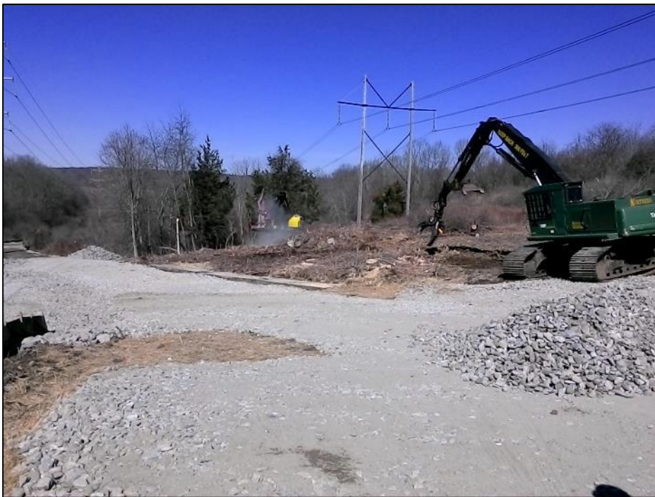
Photo #4: (Up-line) of tree clearing activities.
