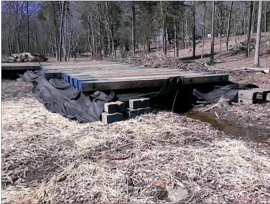
Photo #13: (down-line) temporary mat crossing over S20-21
