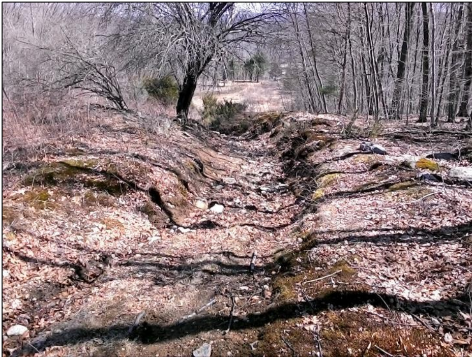
Photo #8: (up-line, right of str 71) View of existing ROW access road set to be replaced due to multiple years of erosion.
