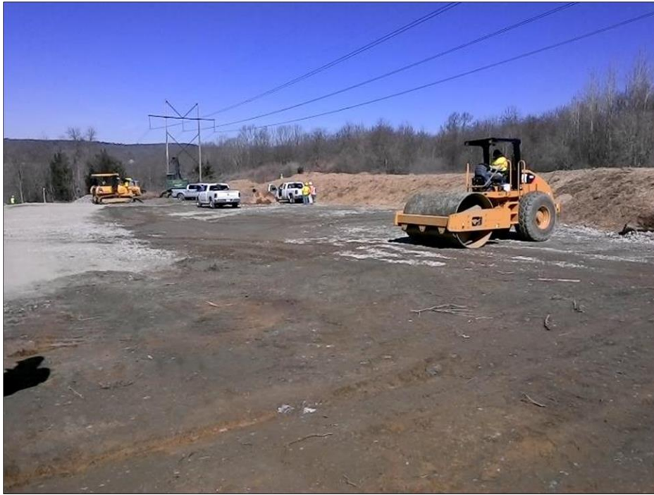
Photo #3: (Up-line) Construction of Pad 3.
