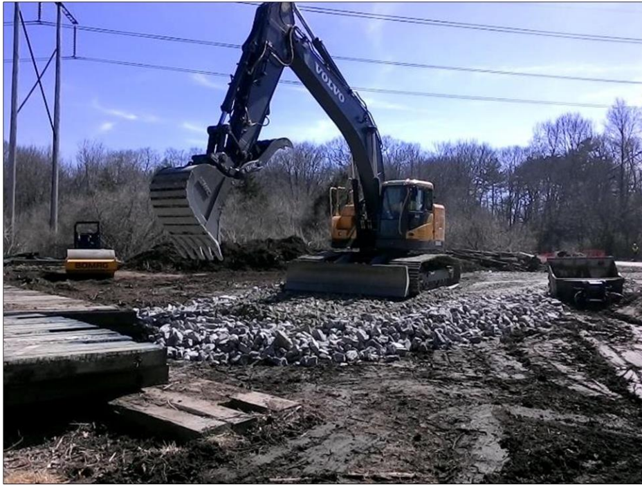
Photo #11: View of Str 91pad under construction.
