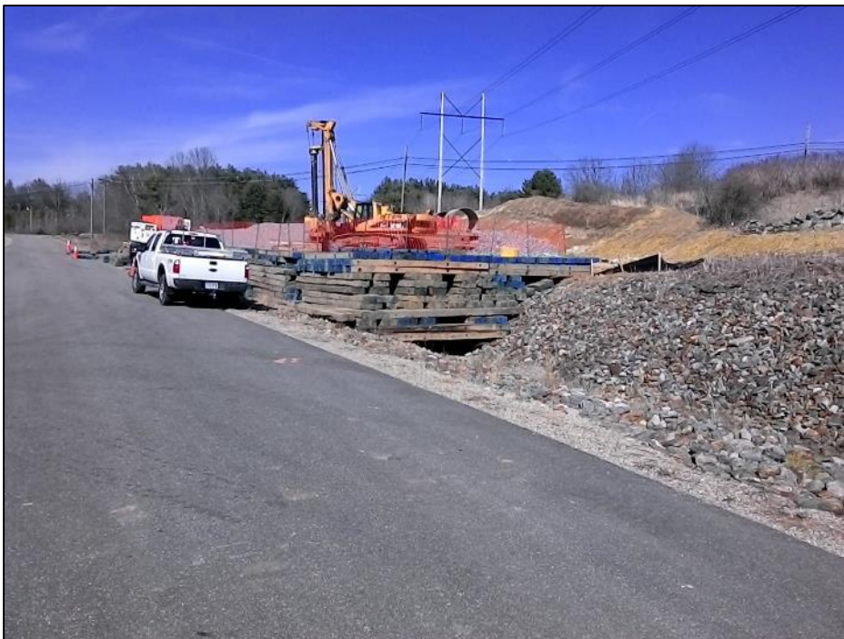
Photo #14: (up-line of 272) preparation of commencement of drilling operations.
