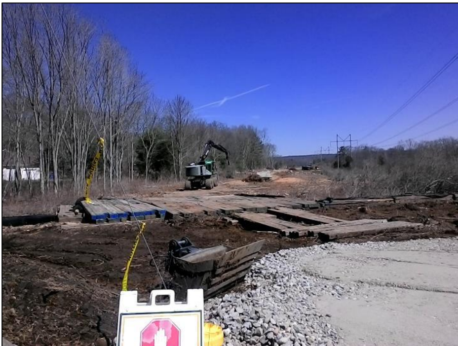
Photo #12: (up-line of str 91) Temporary mat crossing over S20-20
