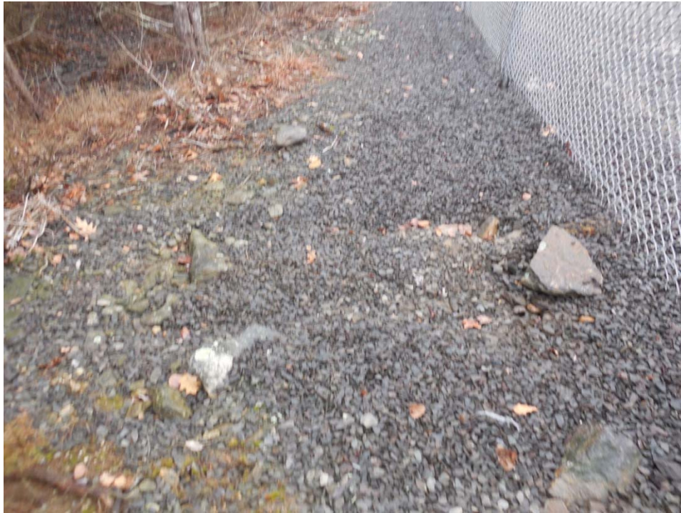
Photo #1: View (facing west) of runoff outlet at southwestern edge of substation with no apparent sedimentation.
