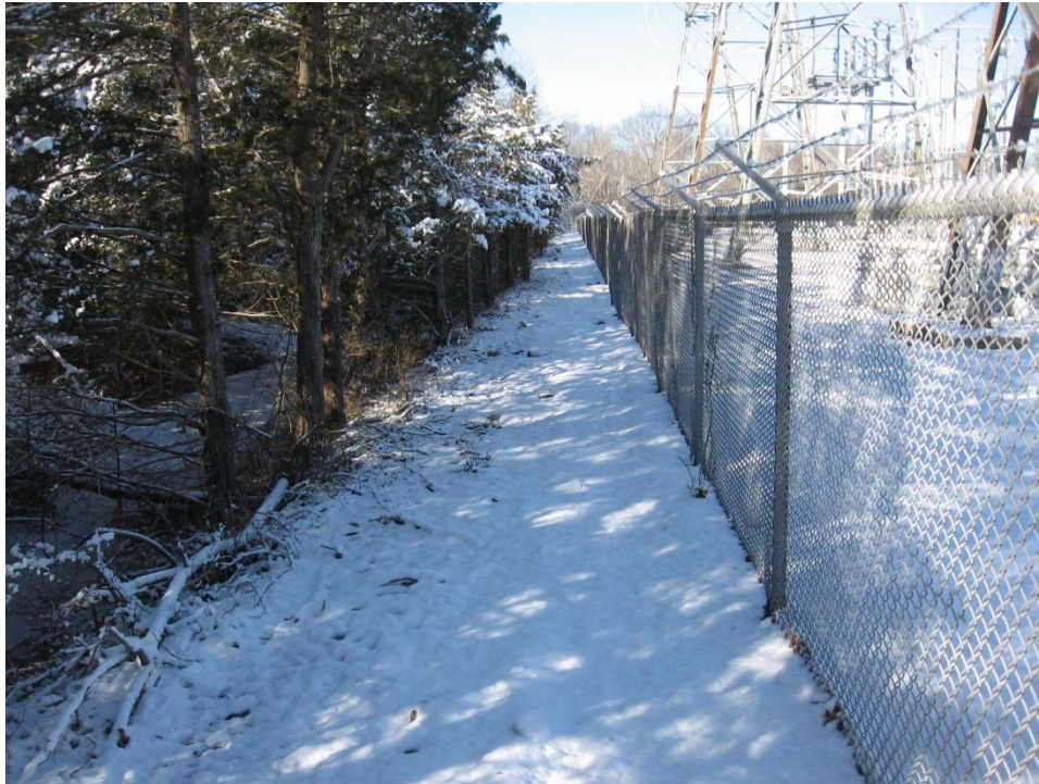
Photo #1: View (facing west) of southwestern edge of substation.
