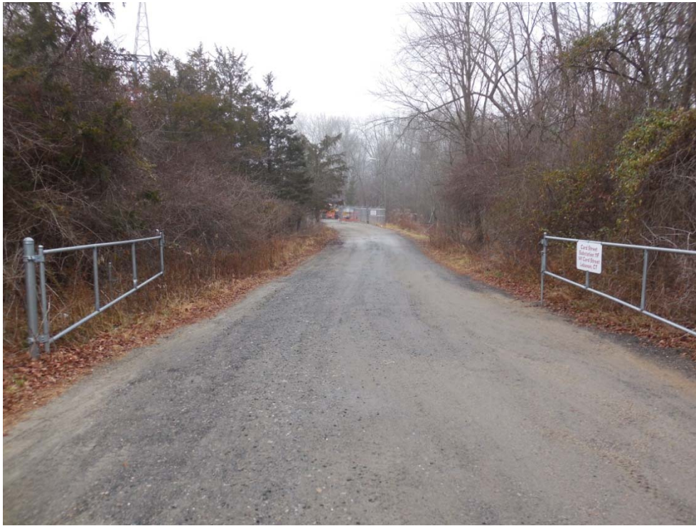
Photo #5: View (facing north) of heavily tracked and compacted entrance pad to substation.
