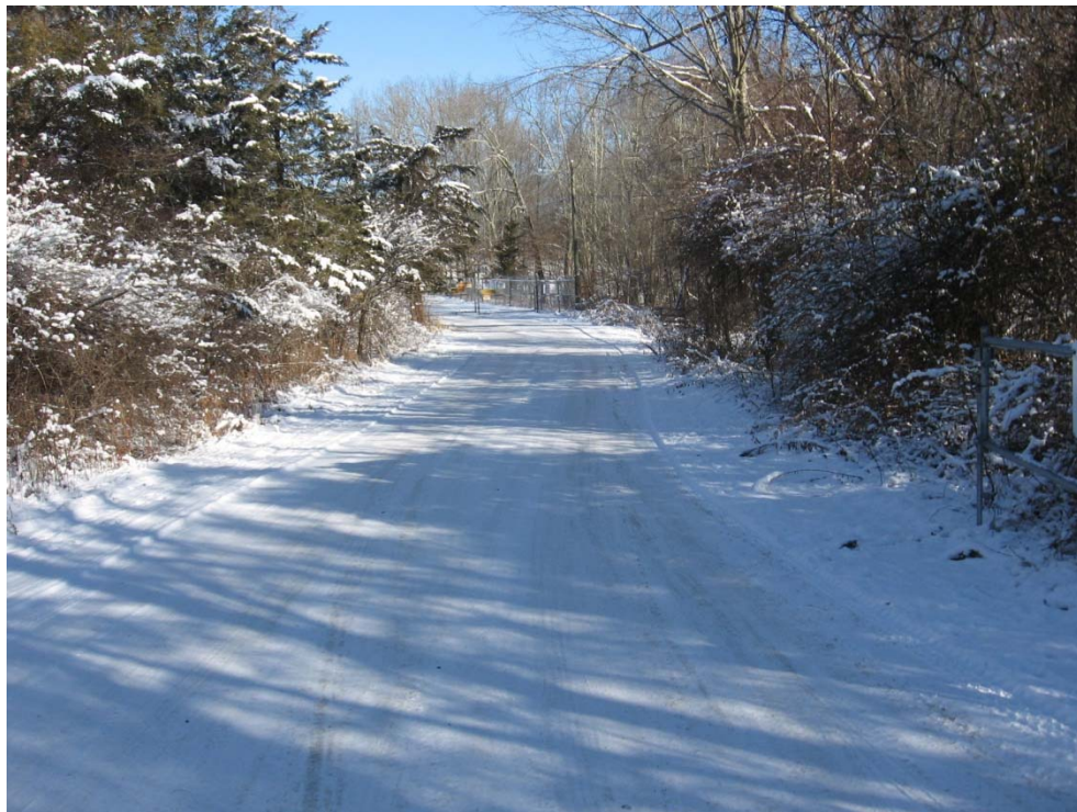
Photo #5: View (facing north) of frozen and stable entrance to substation.
