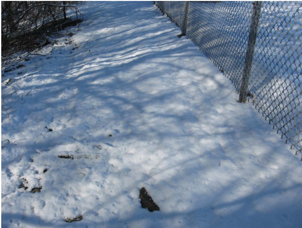
Photo #4: View (facing west) of third (main) runoff outlet at southwestern edge of substation with no apparent sedimentation.
