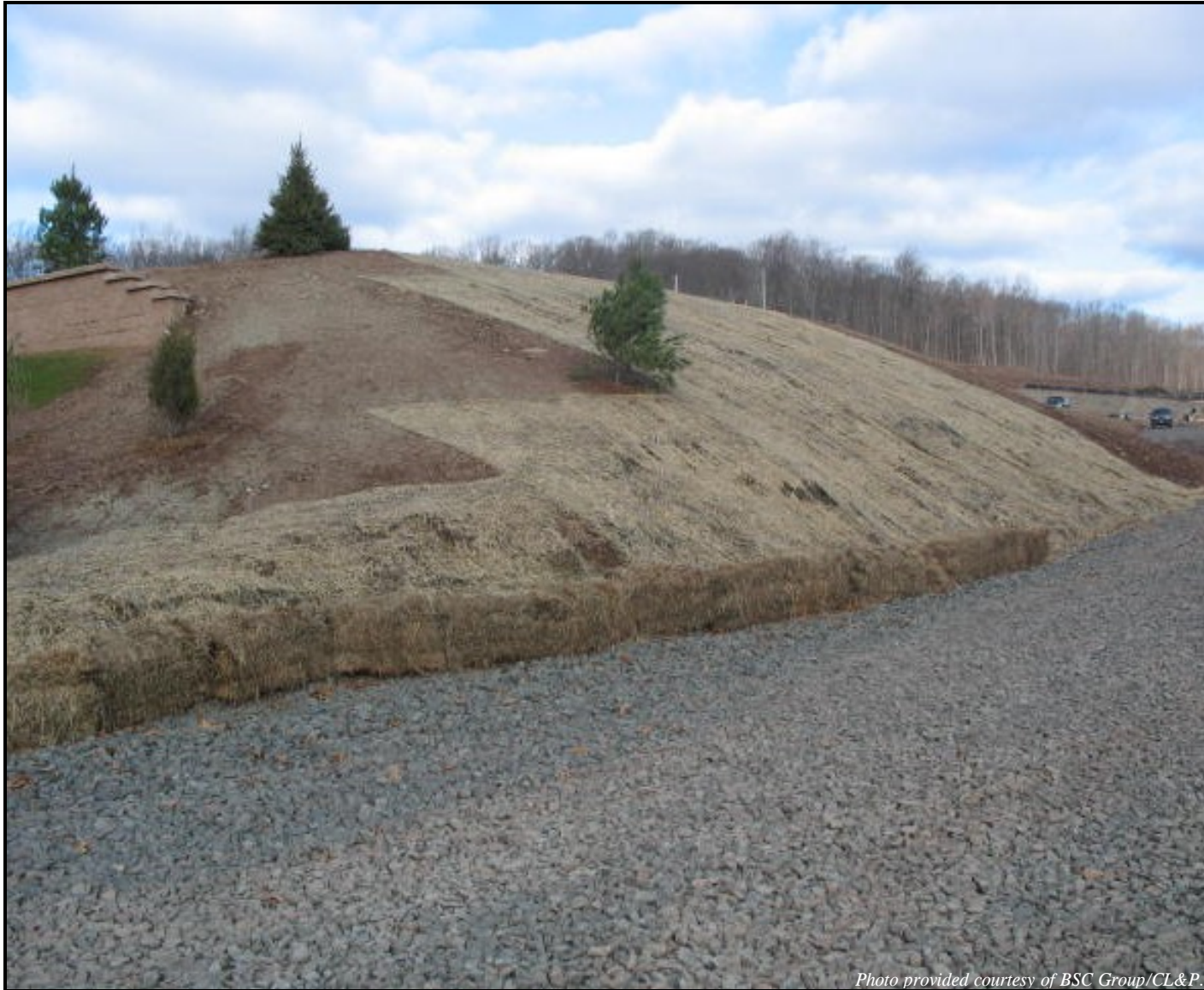
Photograph 4-6 View of properly installed erosion control blankets.
