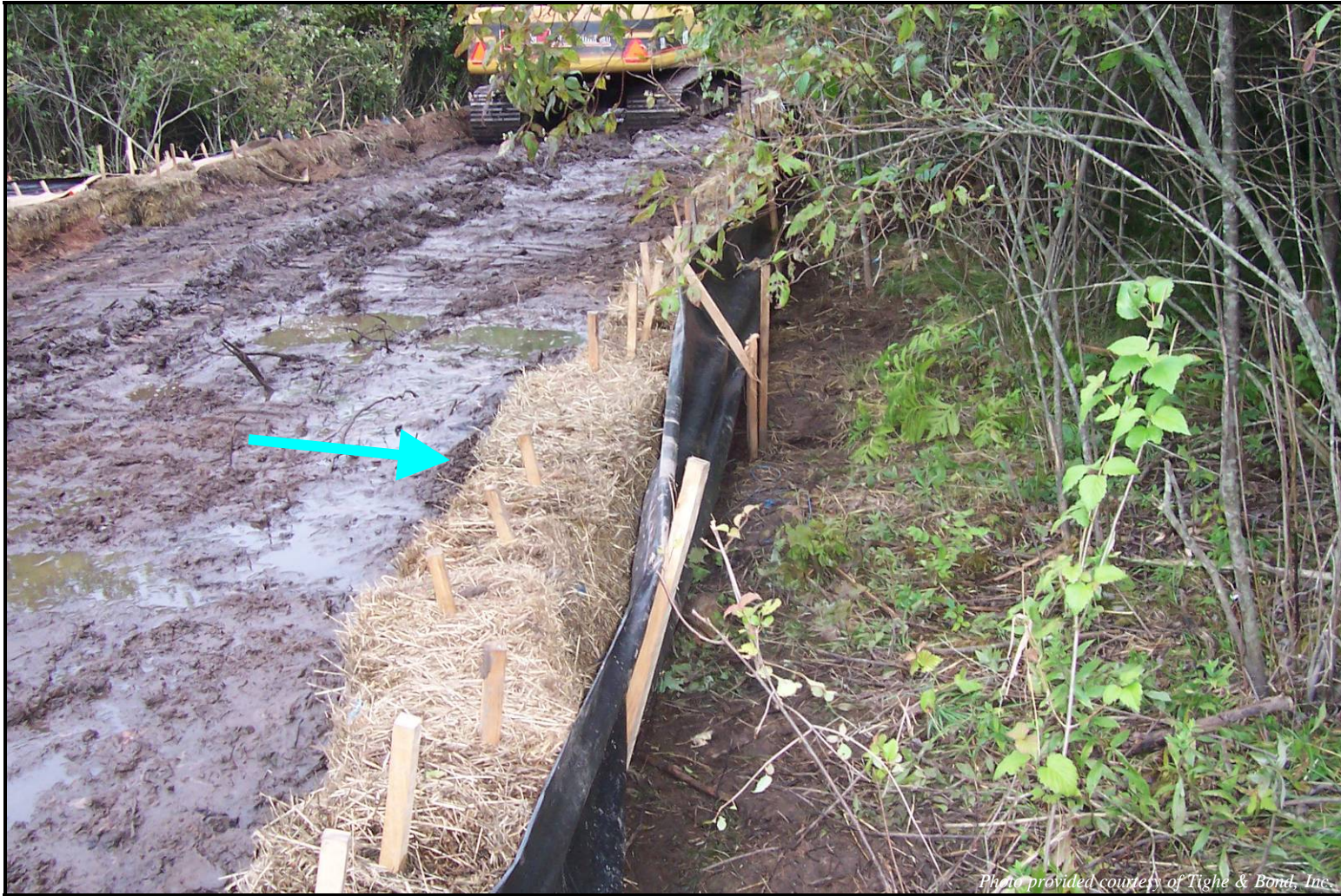
Photograph 4-1 Properly installed hay bale barrier with silt fence. Direction of flow indicated by blue arrow.
