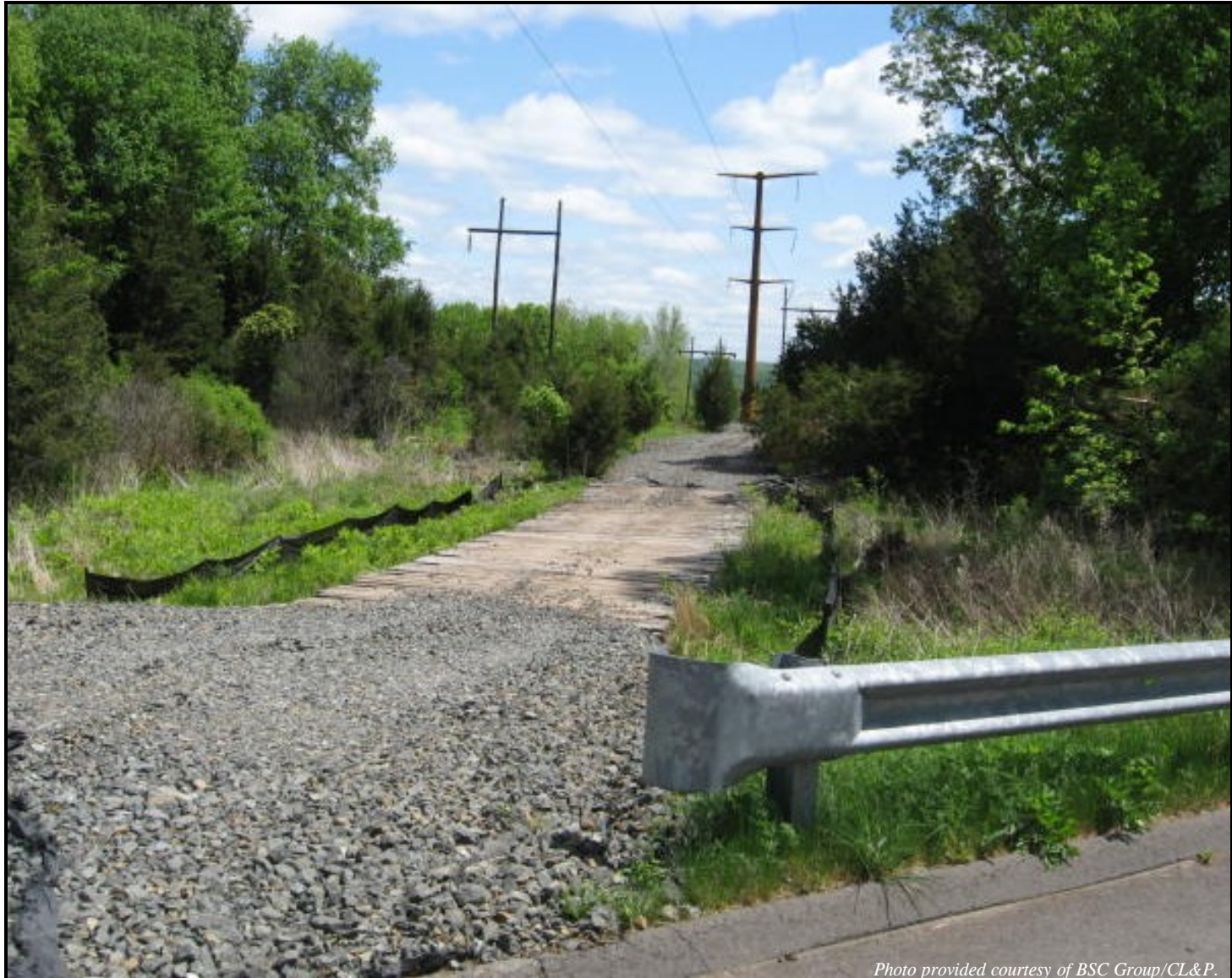
Photograph 6-1 Construction entrance track pads (large site/corridor work).
