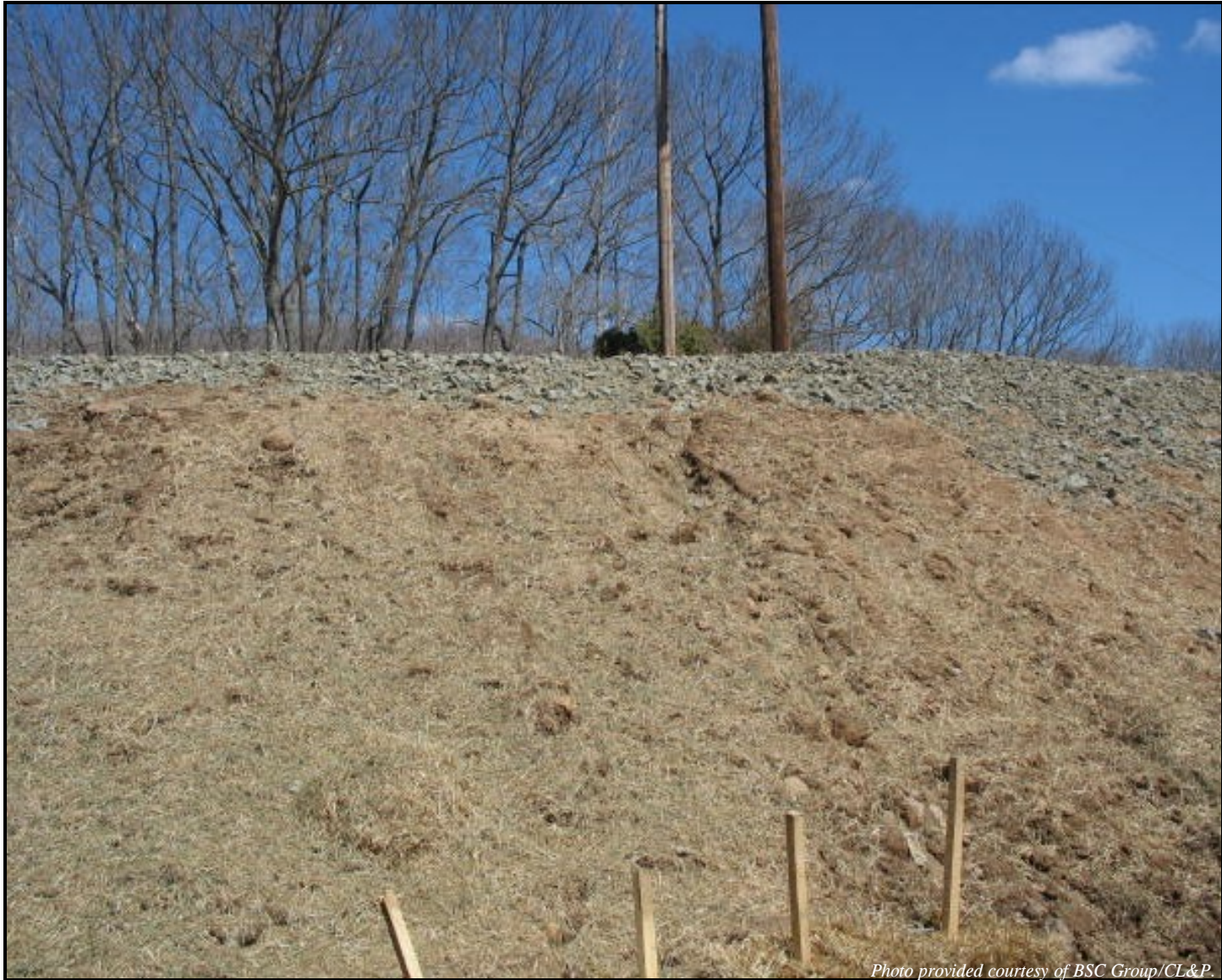
Photograph 12-1 Typical view of light mulching atop unstable, seeded soils.
