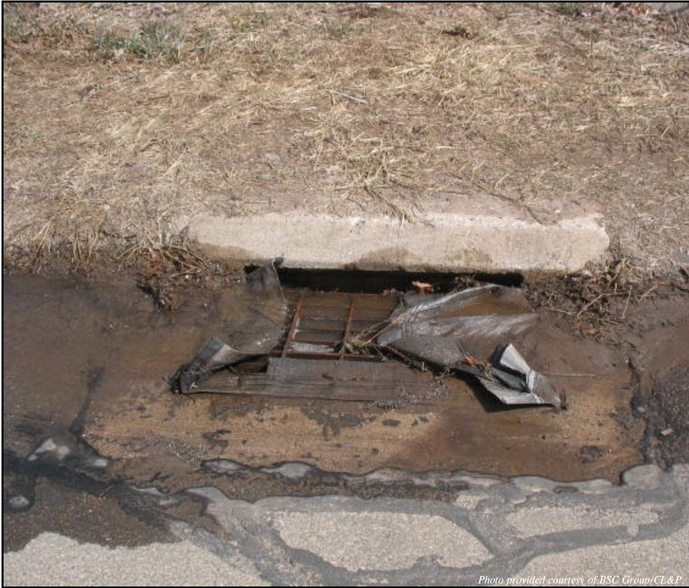
Photograph 9-1 Discharge to storm drain system. Catchbasin protected from sedimentation by filter fabric.
