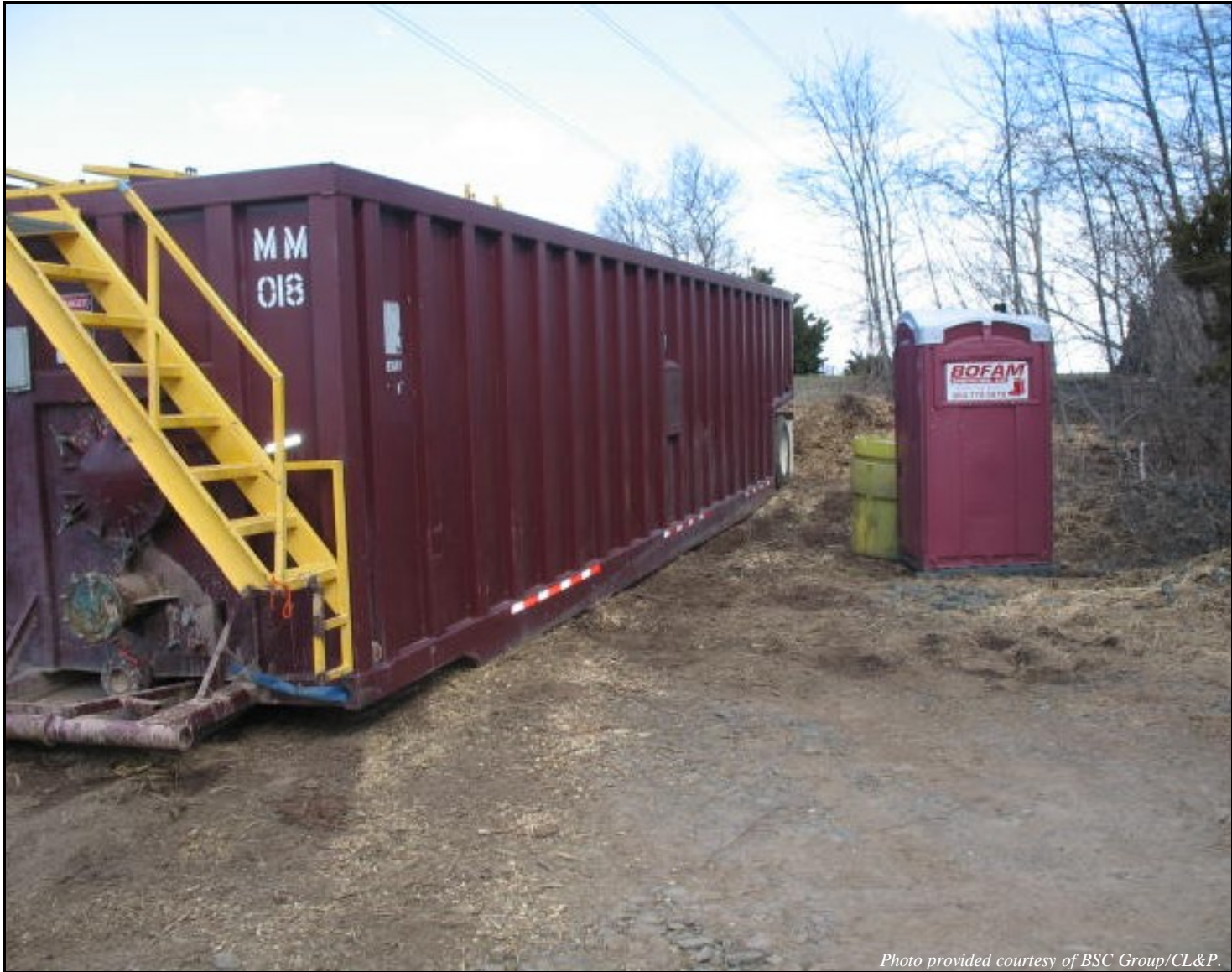
Photograph 9-5 Frac tank on-site for dewatering activities.
