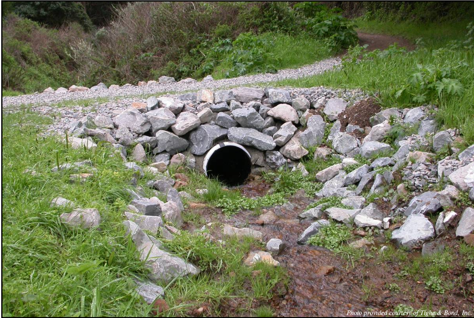
Photograph 5-2 Temporary (long-term) culvert and rip rap for stream crossing.
