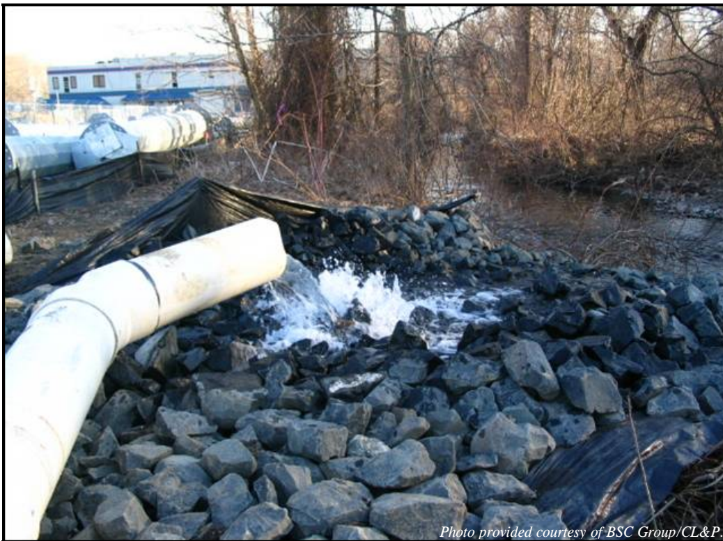
Photographs 9-3 and 9-4 Dewatering to filter “sock” surrounded by haybales (top) and to riprap underlain by geotextile fabric (bottom). Riprap provides velocity dissipation to minimize erosive force of dewatering discharge.
