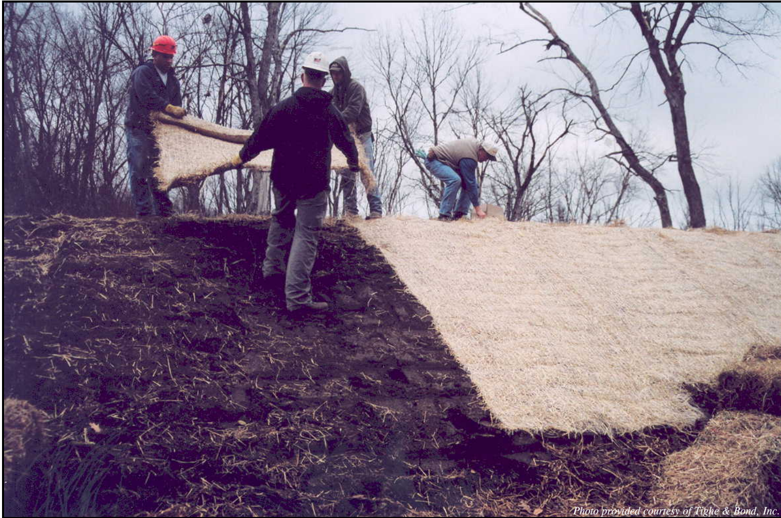
Photograph 4-5 Installing erosion control blanket on an unstable slope.
