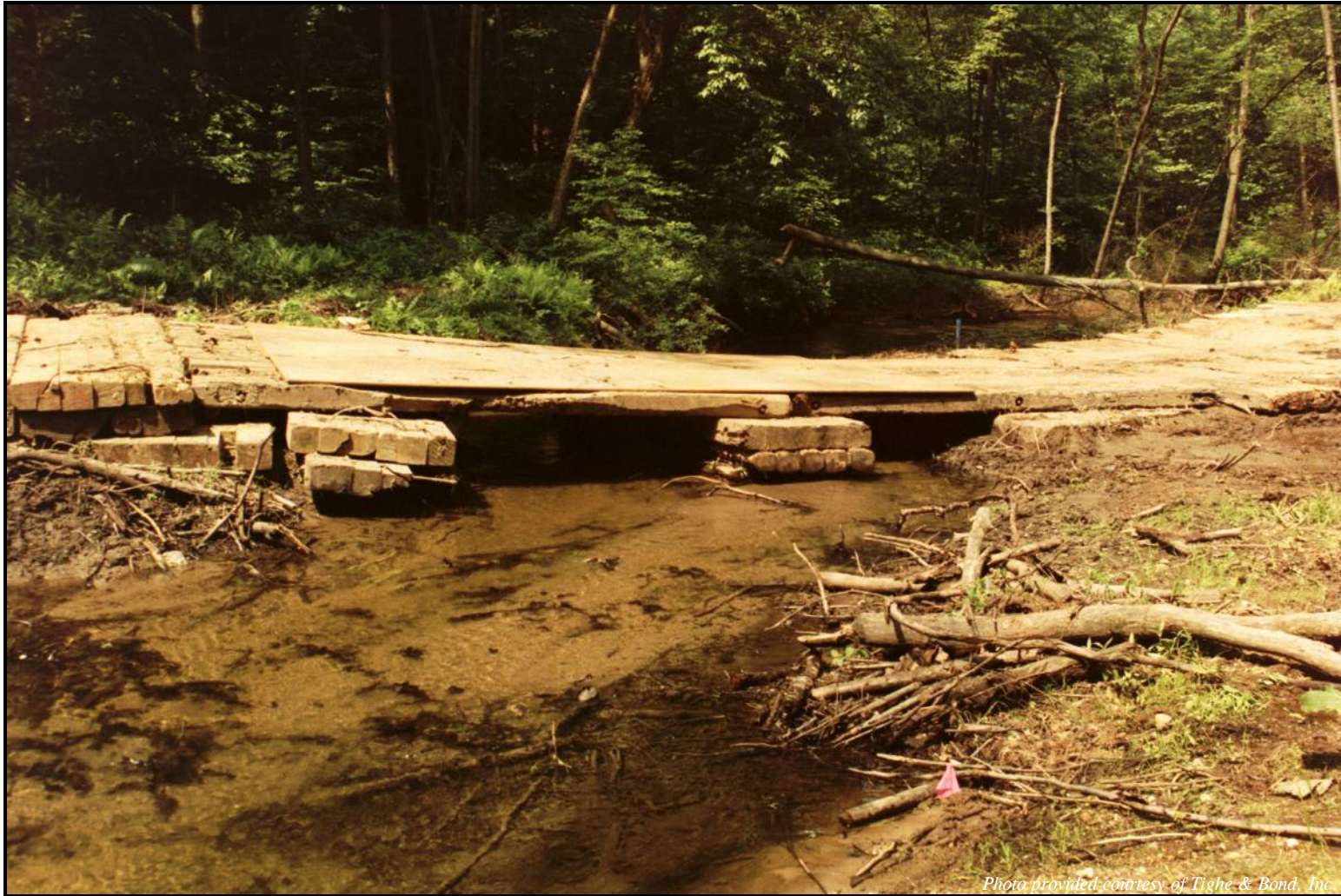
Photograph 5-1 Swamp mat bridge.
