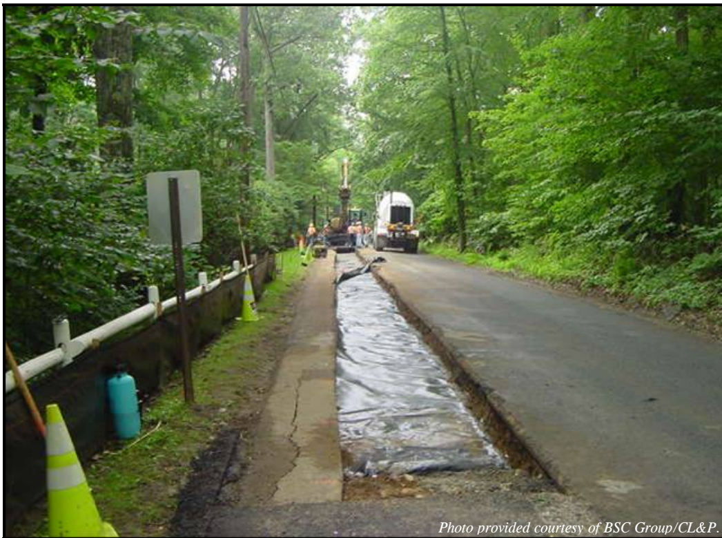
Photographs 9-6 and 9-7 Typical underground construction activities where dewatering may be required.
