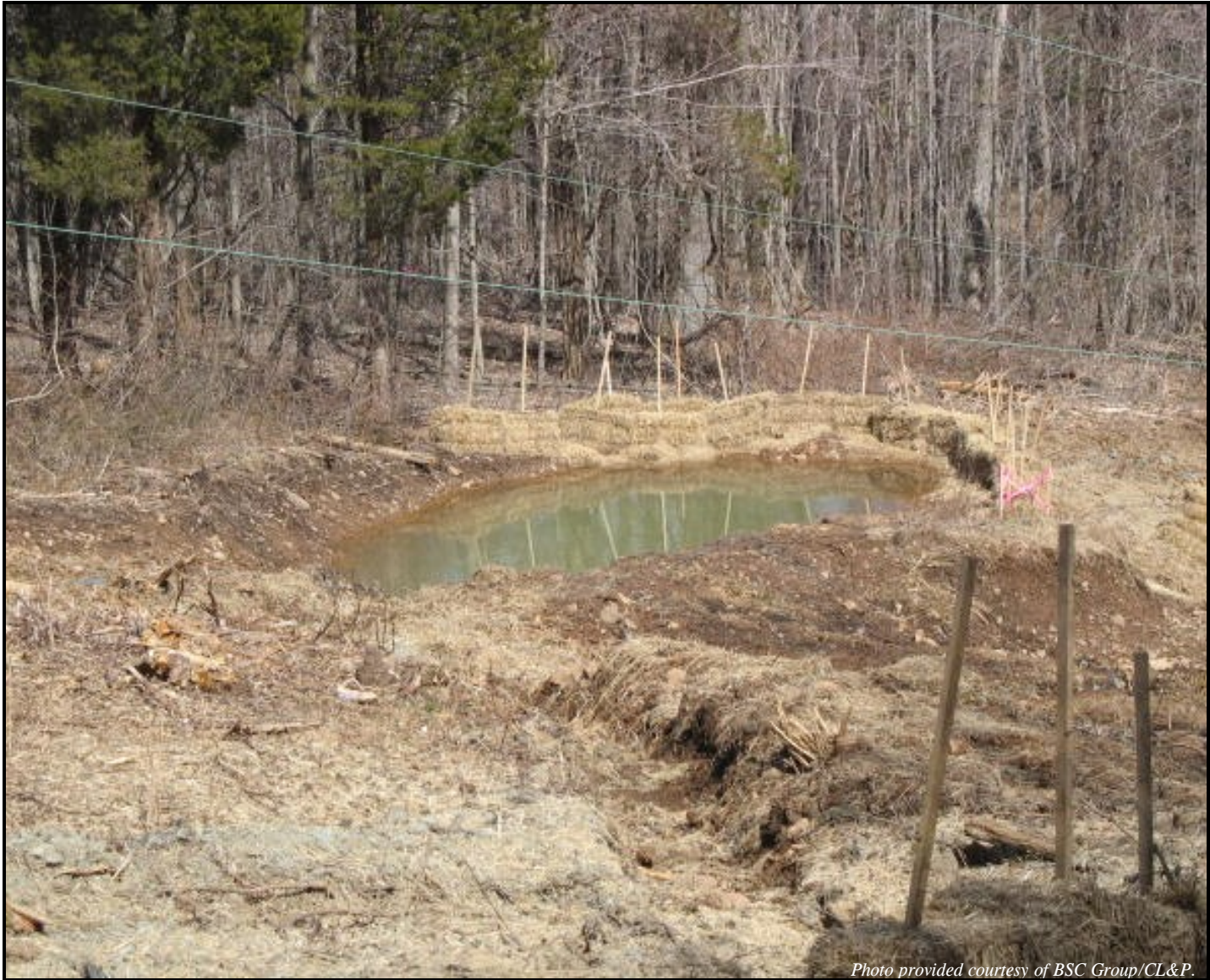
Photograph 9-2 Sedimentation basin.
