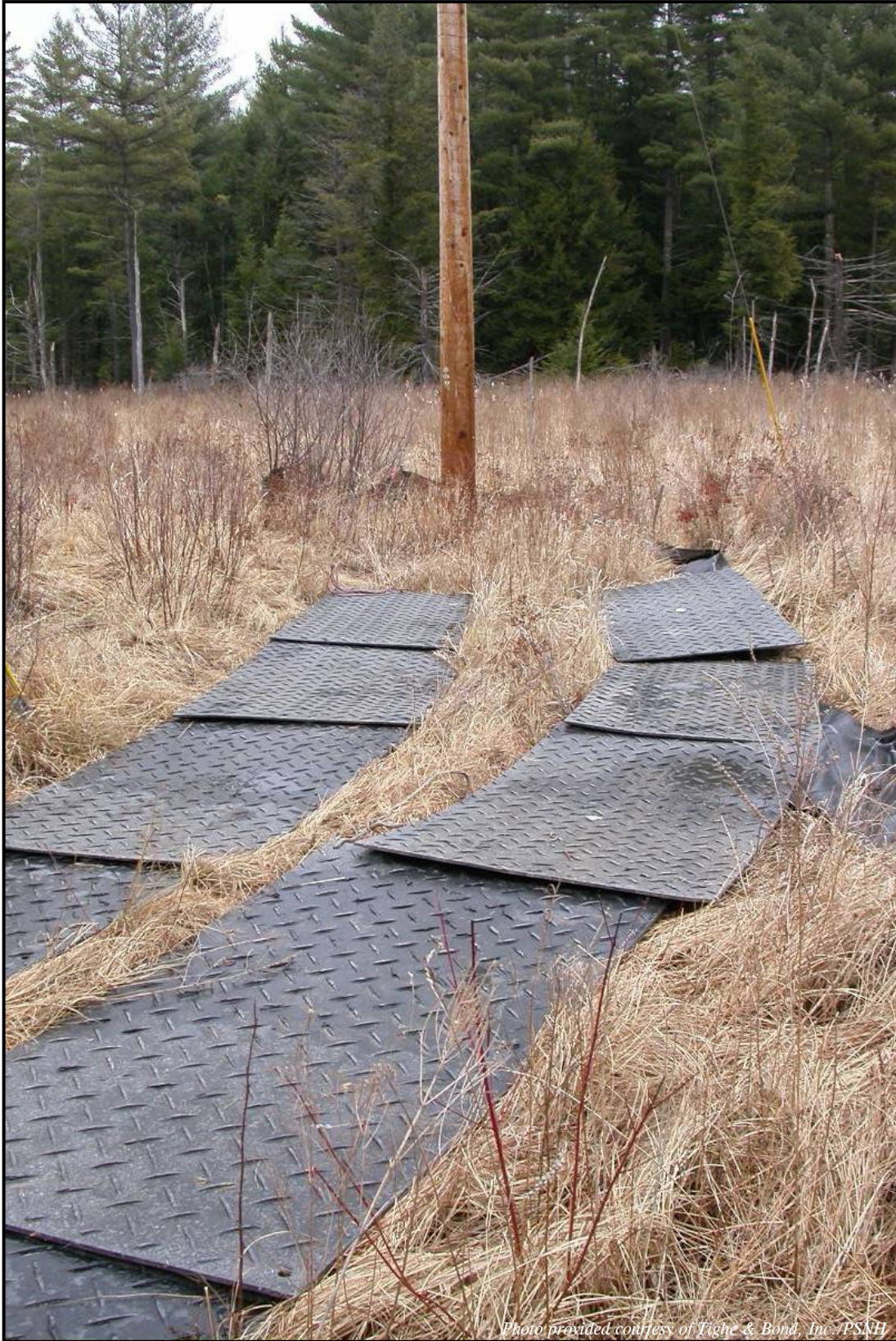
Photograph 5-4 AlturnaMAT® tracks to utility pole in wetland.
