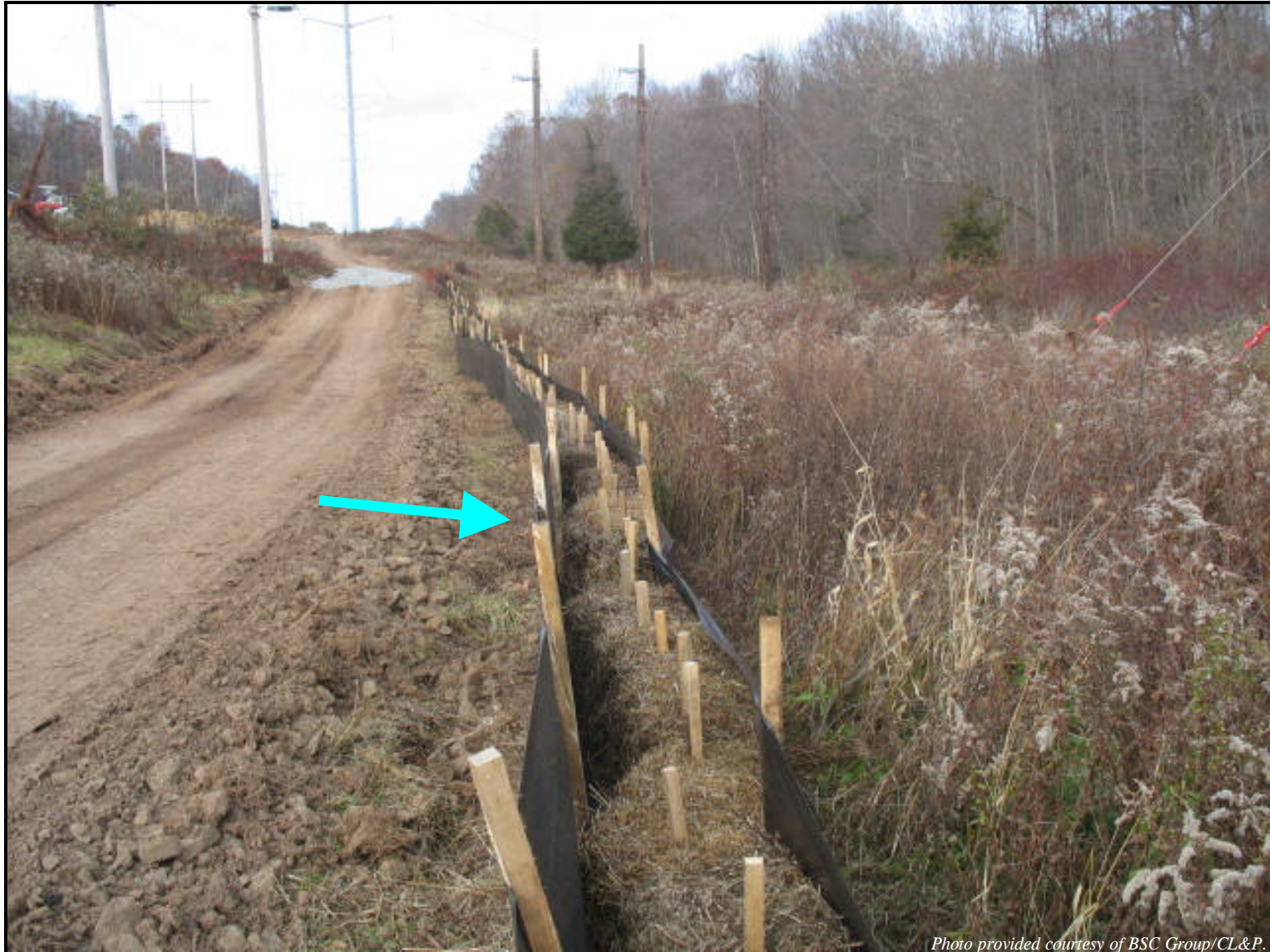
Photograph 4-4 Hay bale barrier with double-row of silt fence. Direction of flow indicated by blue arrow.
