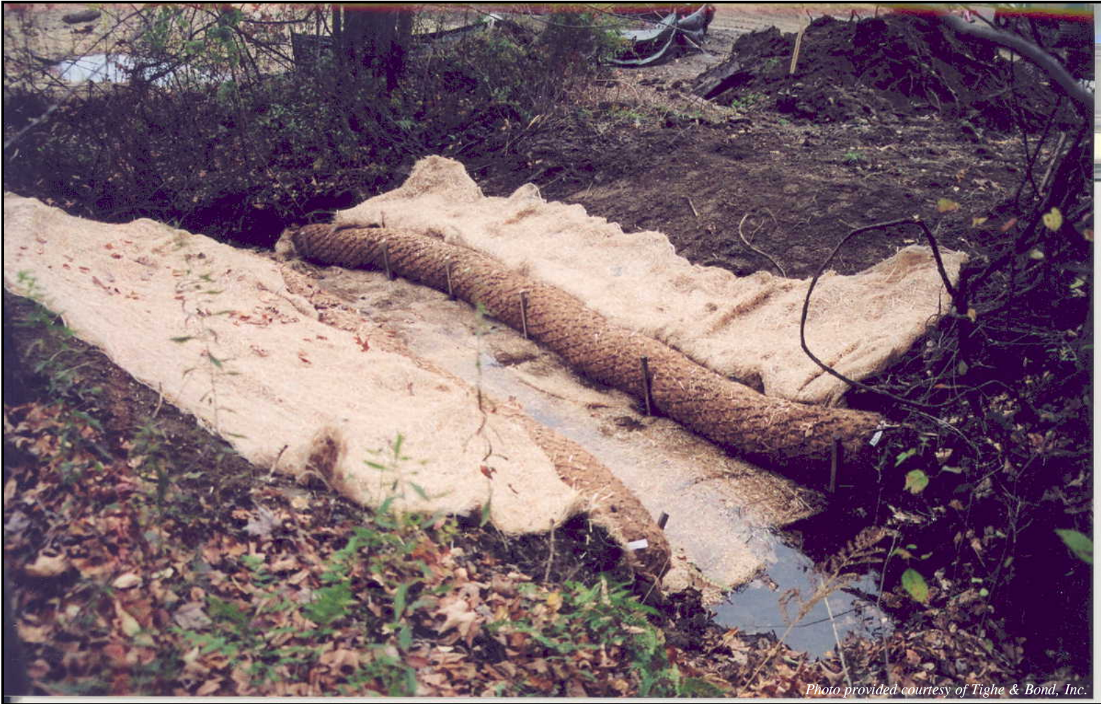
Photograph 12-2 Erosion control blanket and coir logs used to restore a stream bed and banks.
