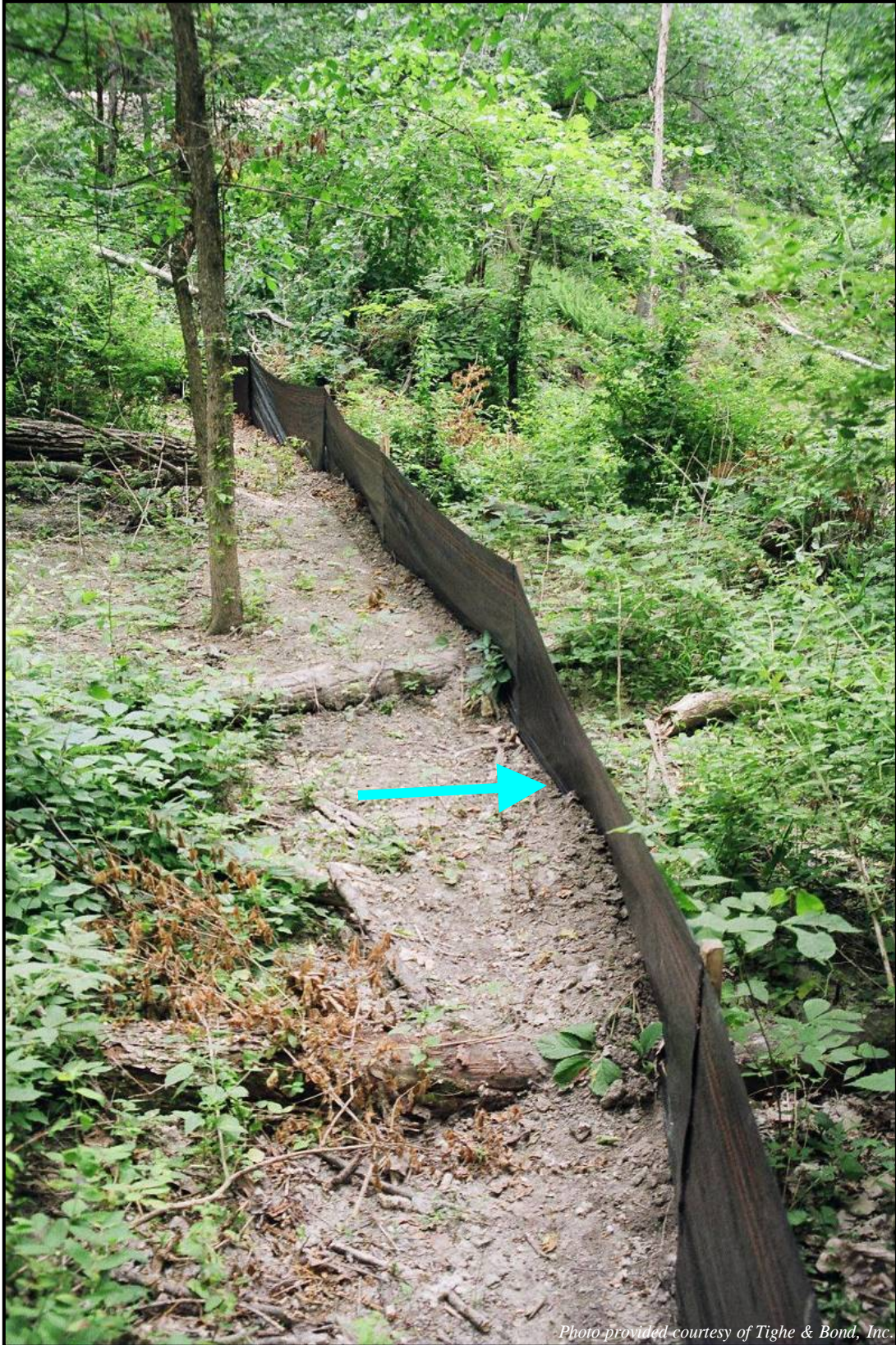
Photograph 4-2 Properly installed and functioning silt fence. Direction of flow indicated by blue arrow.
