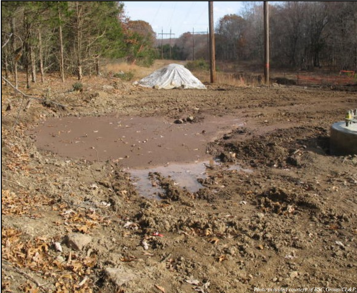
Photograph 4-9 [Polluted/contaminated] soil stockpile management.
