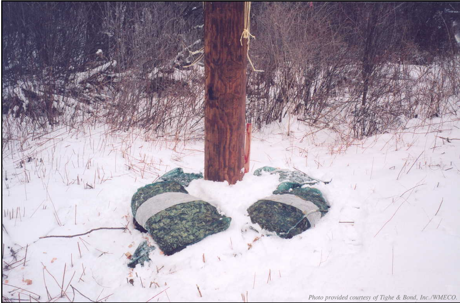
Photograph 4-7 Wood chips in photo-degradable bags used to stabilize soils.
