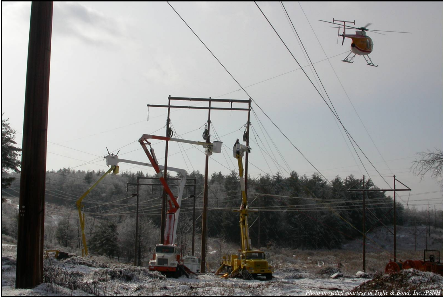
Photograph 5-5 Use of aerial equipment for transmission line construction.
