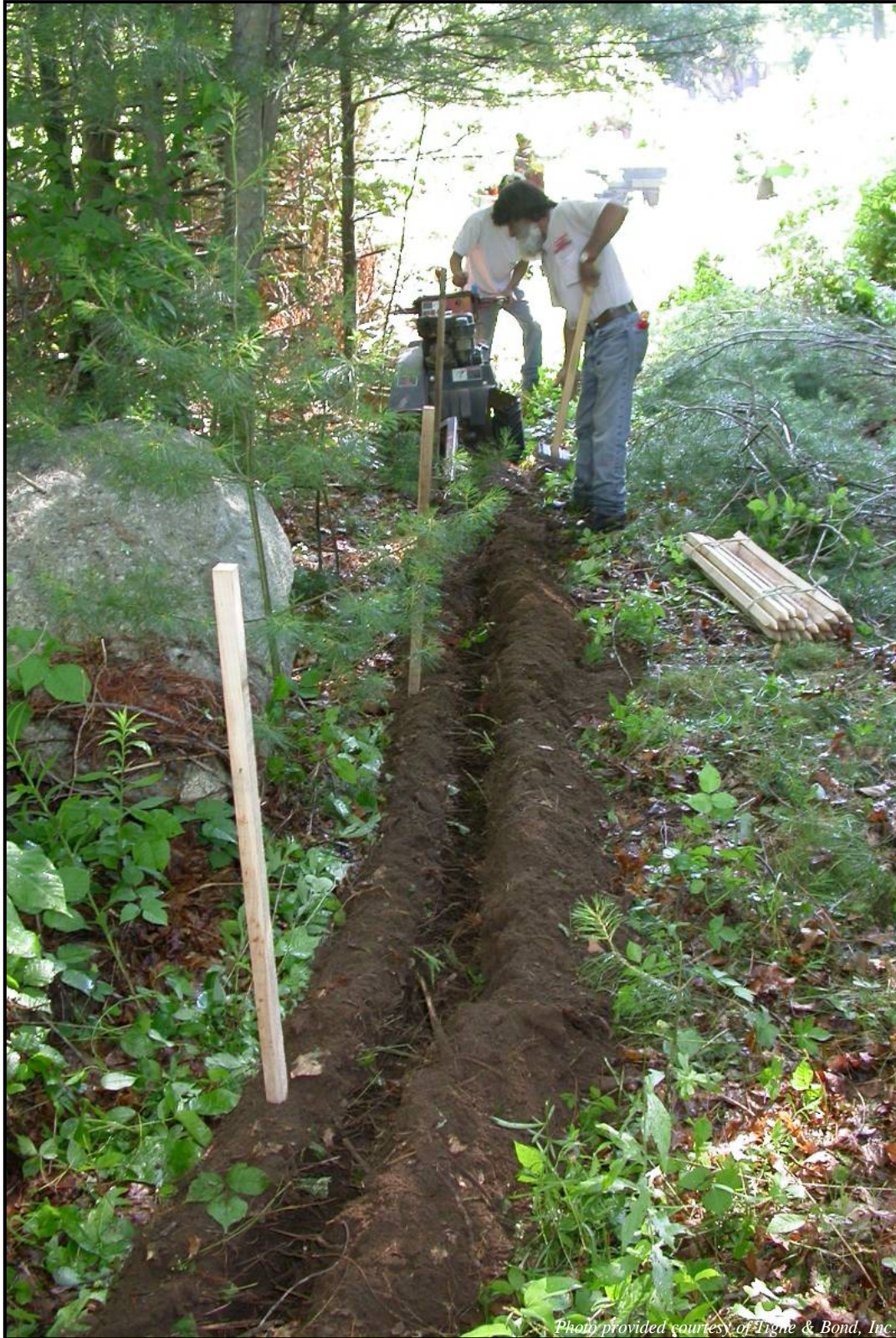
Photograph 4-3 Using a Ditch Witch® to quickly make a trench for proper silt fence installation.
