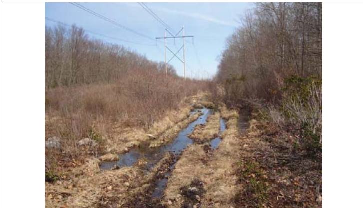
Northeast view of W20-129
