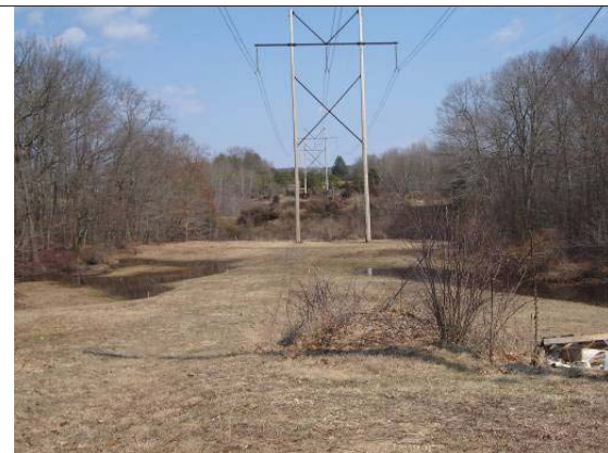
Northeast view of W20-31
