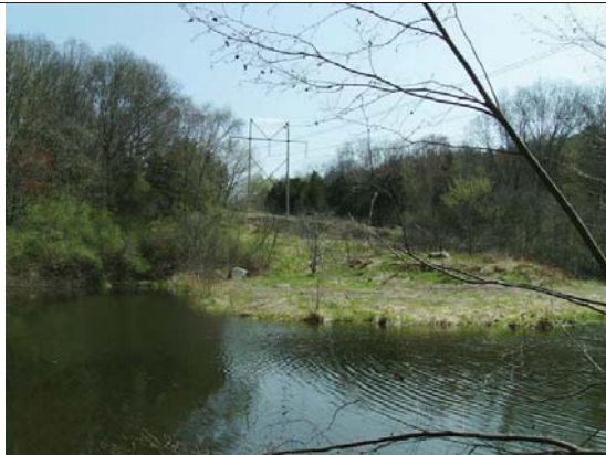
Northeast view of W20-148
