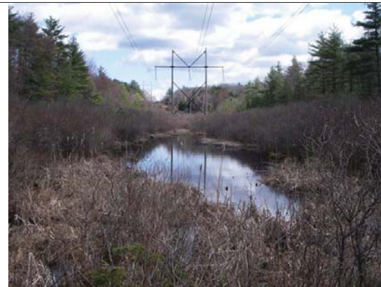
Northeast view of W20-195
